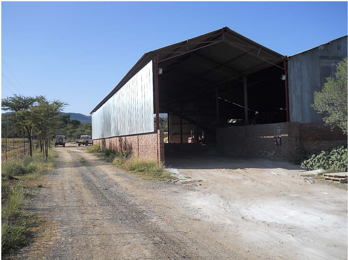
Figure 2. View of the loading bay in the sand drying plant.
