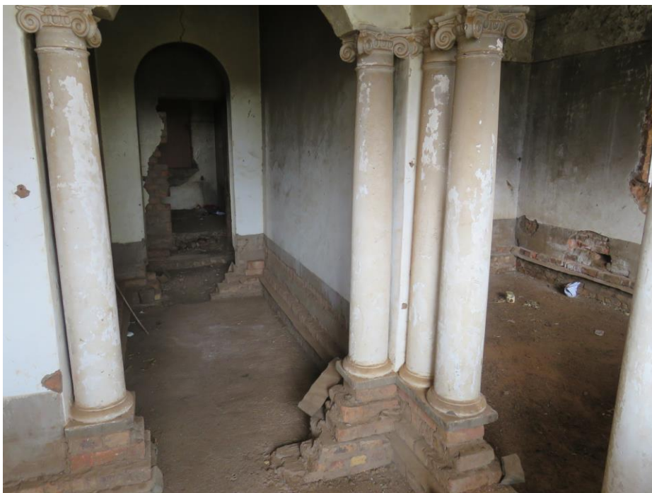
Figure 12: Interior view of the house.
