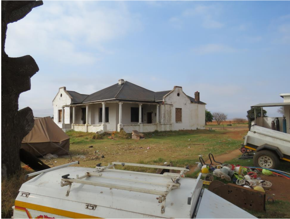
Figure 11: The farm house, just outside of the development area.
