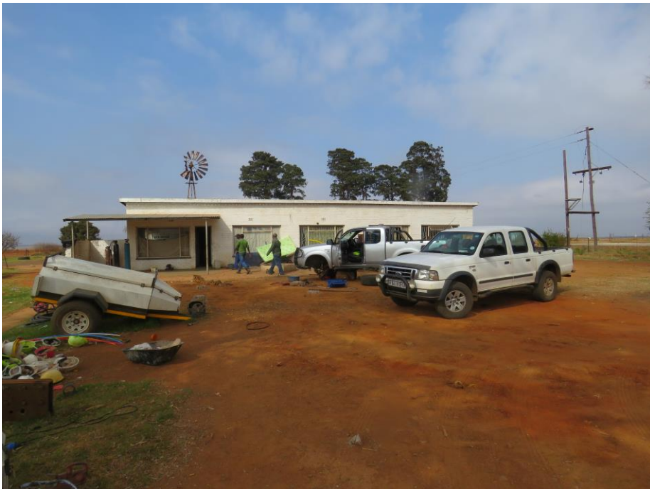
Figure 10: Closer view of the building on site.
