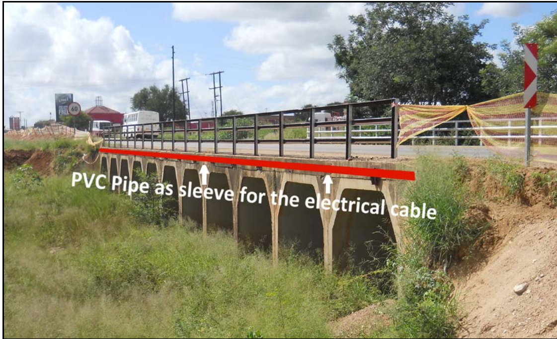
Figure 3. View of the bridge crossing.
