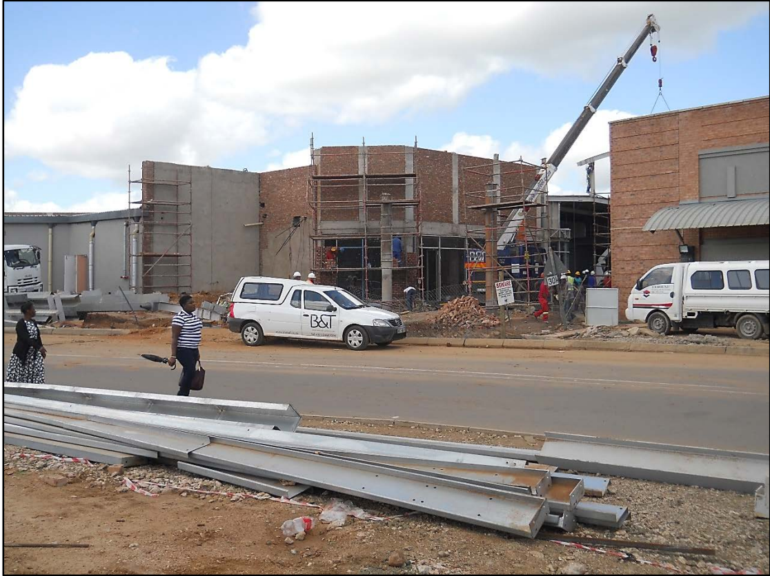
Figure 8. View of the area where the cable trench crosses First Street to enter the Masingita Mall.
