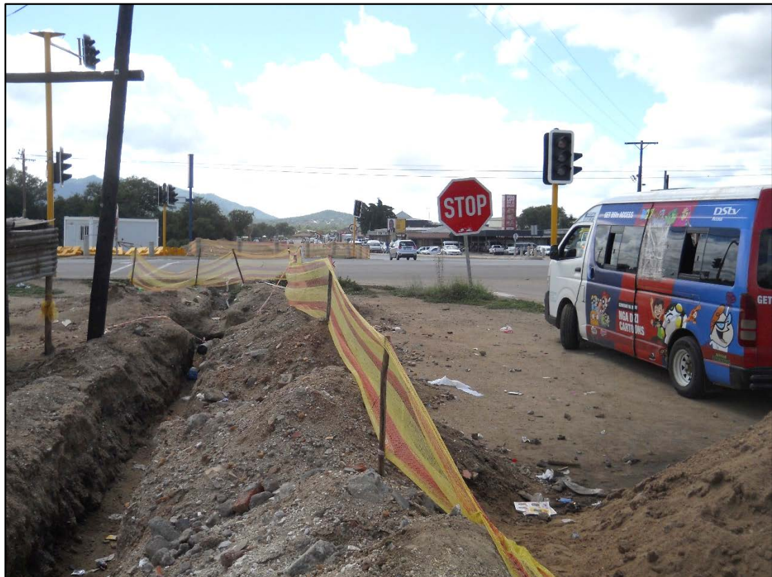
Figure 4. View of the cable trench at the R81 crossing – easterly direction.
