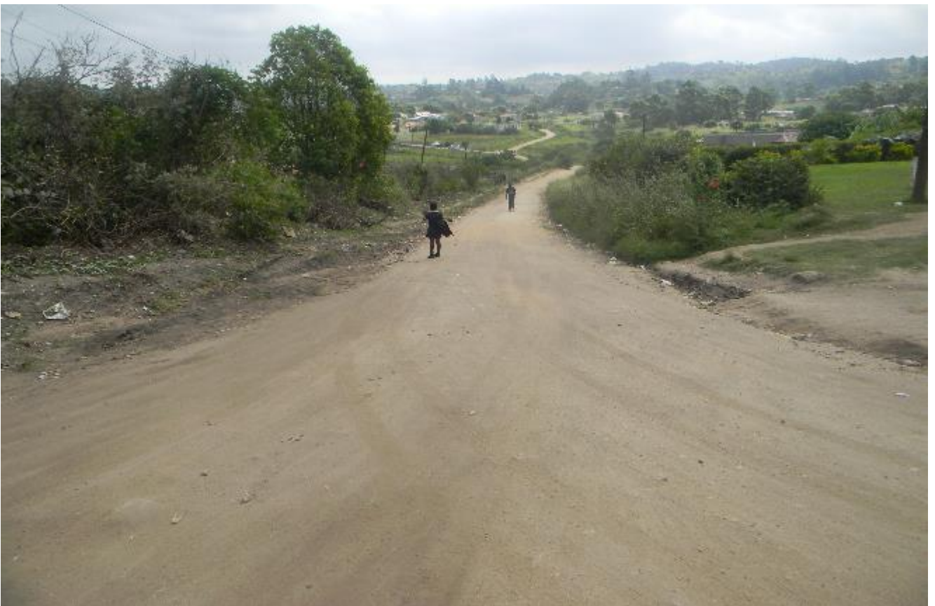
Plate 16: Photo 16: View of pipeline route along road servitude (Photograph © by Author 2017)
