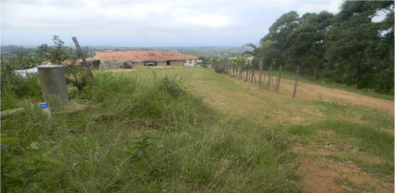
Plate 5: Photo 5: View of existing pipeline earmarked for upgrading running through homesteads (Photograph © by Author 2017)
