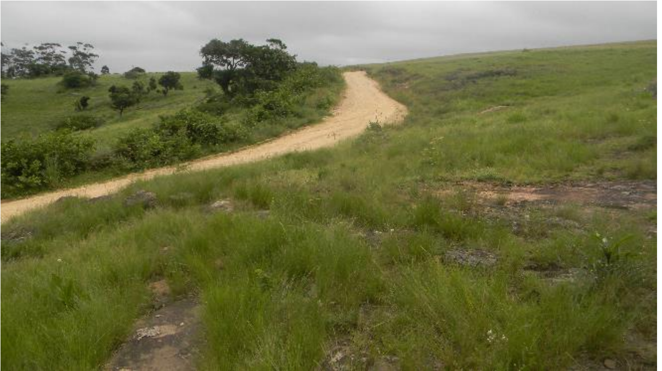
Plate 17: Photo 17: View of pipeline route along road servitude (Photograph © by Author 2017)
