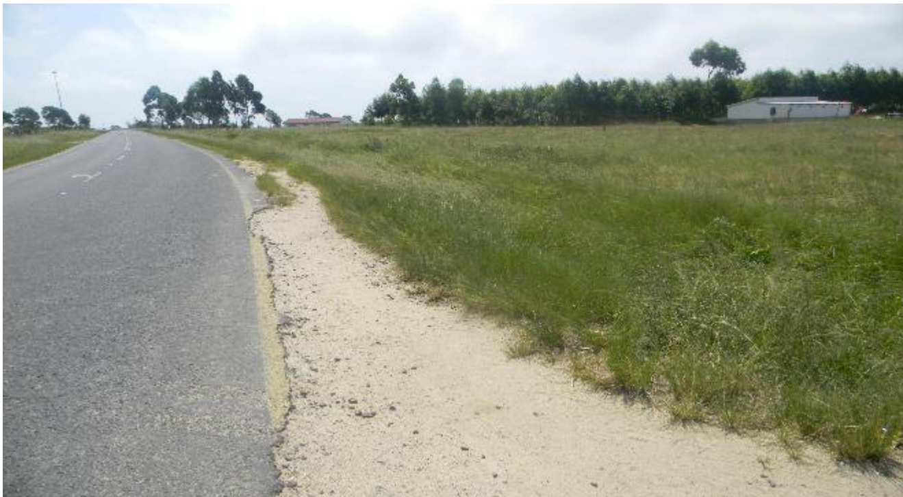
Plate 13: Photo 13: View of pipeline route along road servitude (Photograph © by Author 2017)
