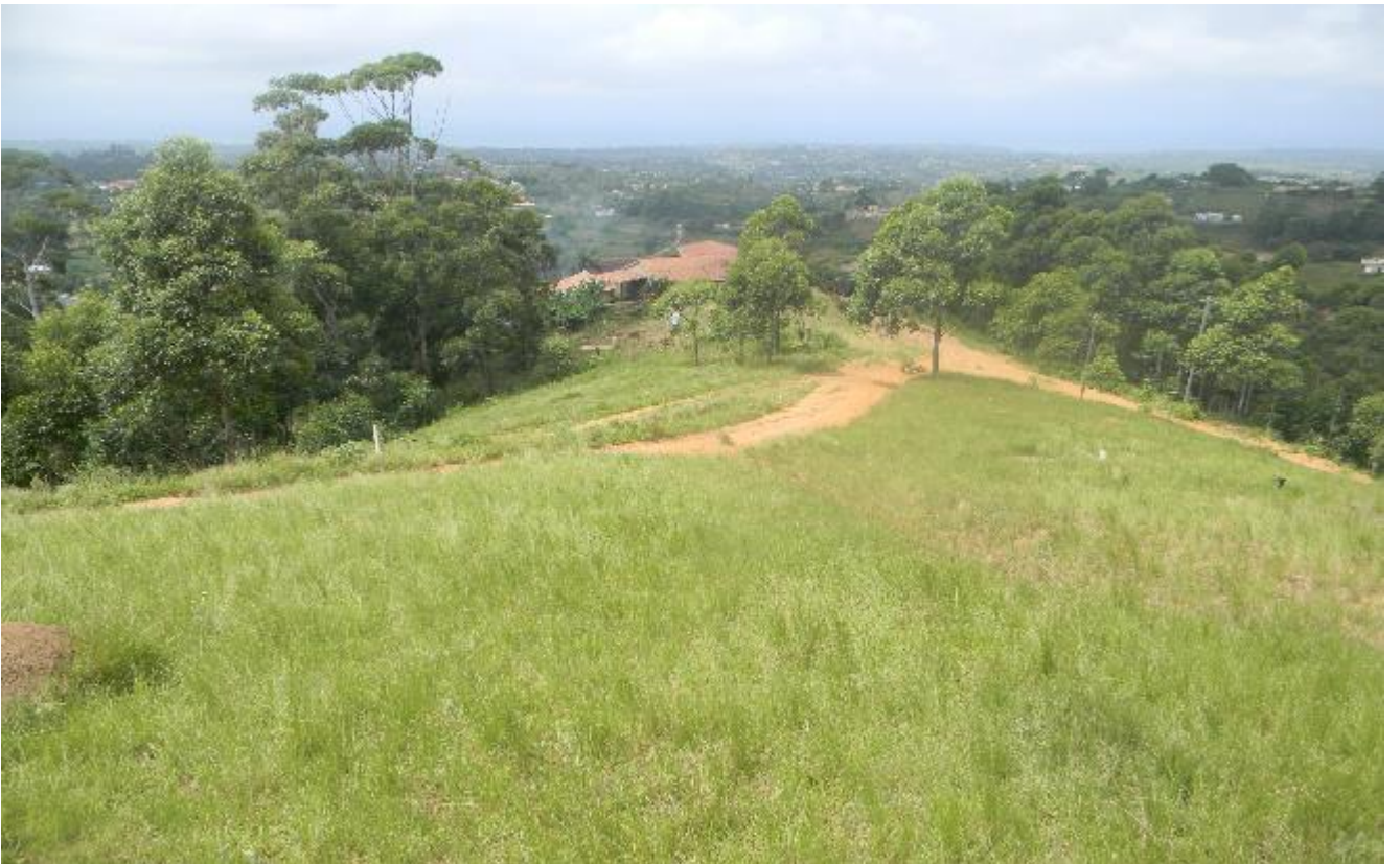
Plate 4: Photo 4: View of proposed pipeline route (Photograph © by Author 2017) Note that the new pipeline is intended to replace the existing pipeline along the same servitude
