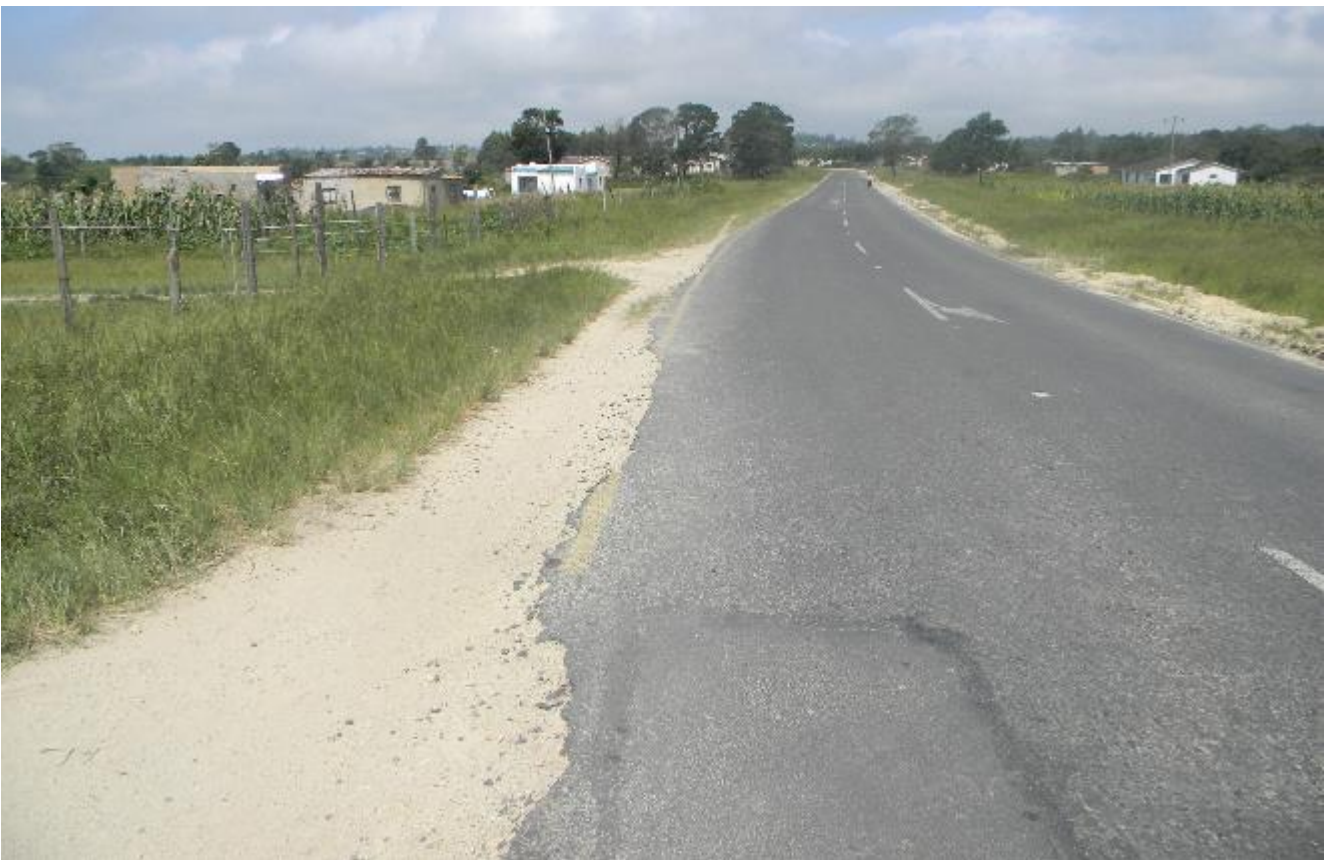
Plate 12: Photo 12: View of pipeline route along road servitude (Photograph © by Author 2017)
