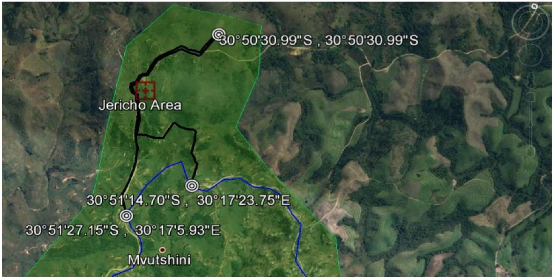
Figure 2: - Jericho Area Site and directions to access to the proposed Pipeline servitude and reservoir sites (Keyenviro 2017)
