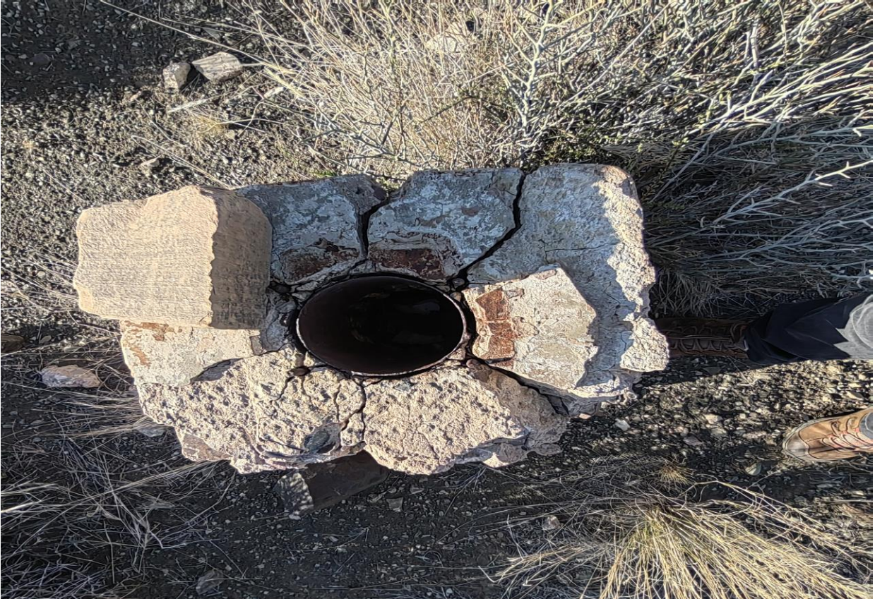
Plate 13: showing an abandoned borehole within the proposed prospecting site
