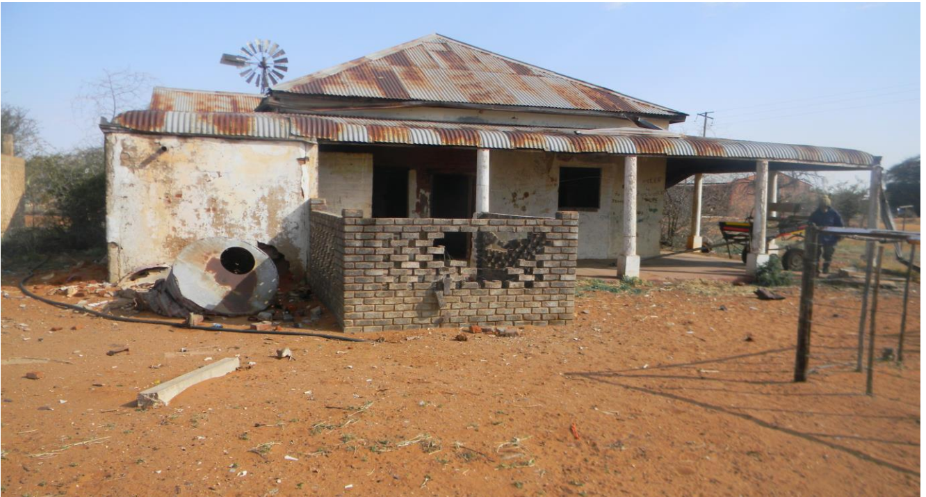
Plate 27: showing a historical farmhouse in its delapidated state of conservation.
