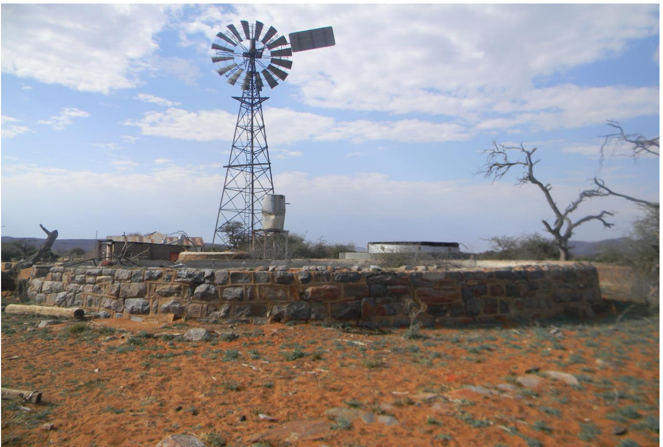
Plate 20: showing wind pump and water reservoir
