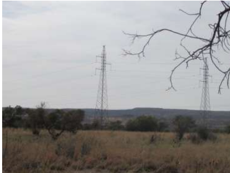
Figure 5: View of the existing Eskom Lines in the area.
