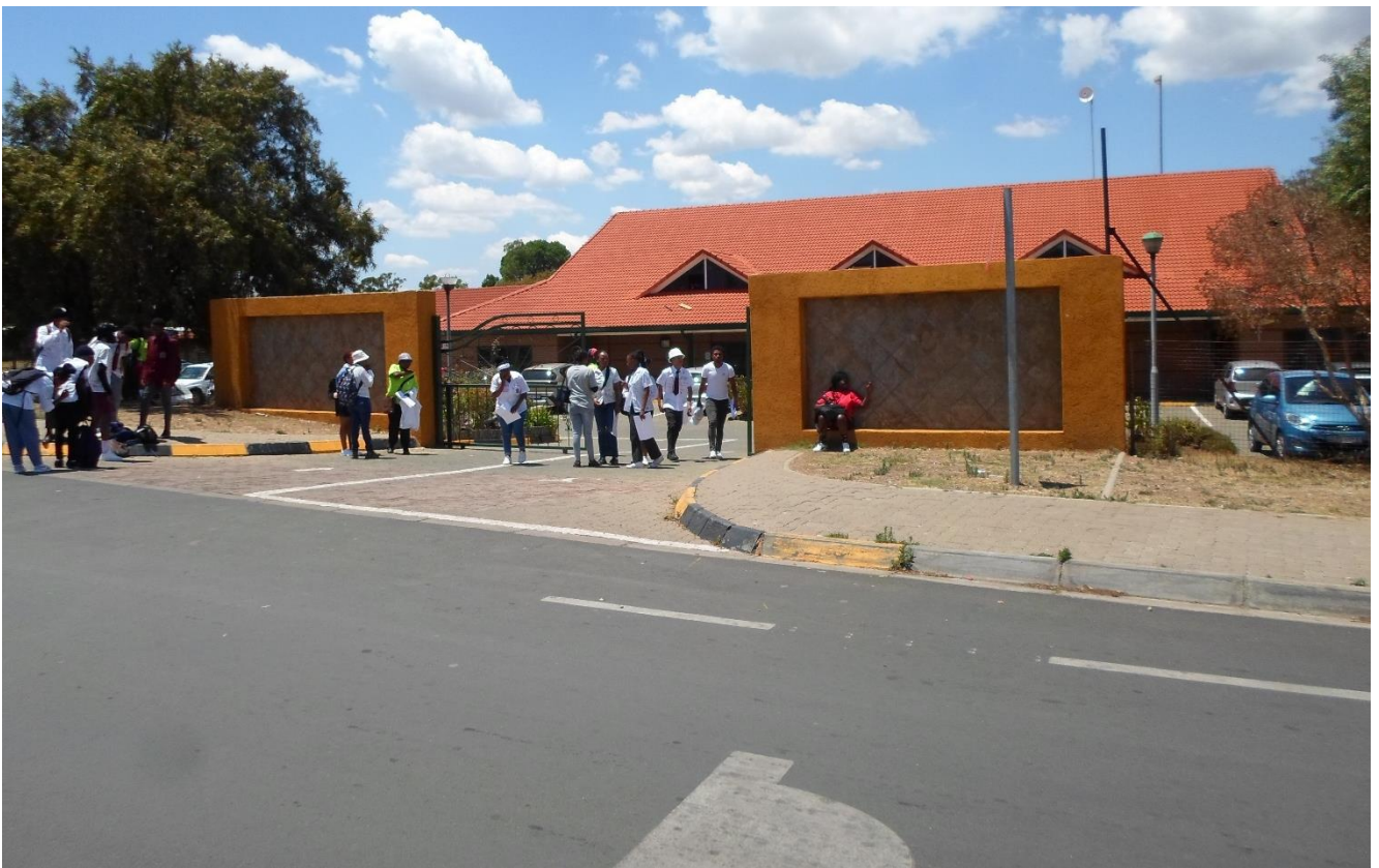
Plate 15: showing the proposed school upgrade site
