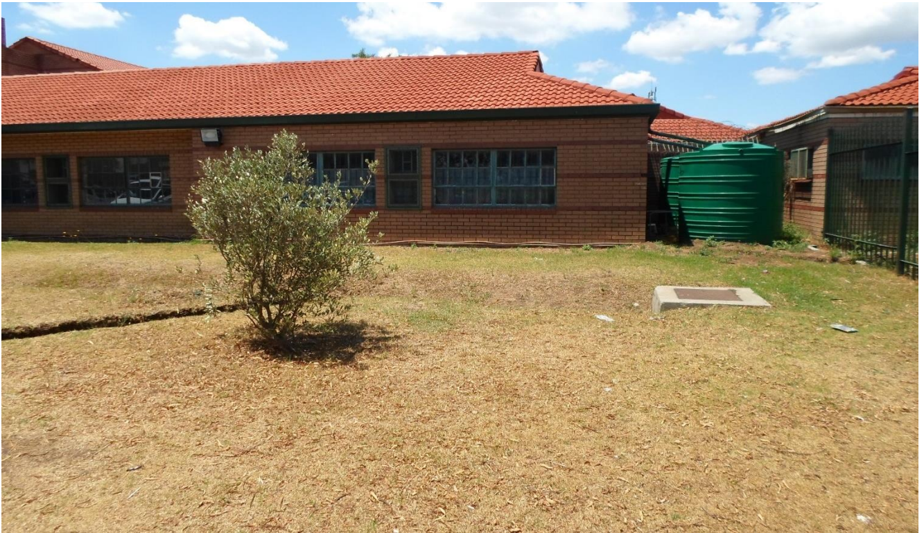
Plate 14: showing the proposed school upgrade site
