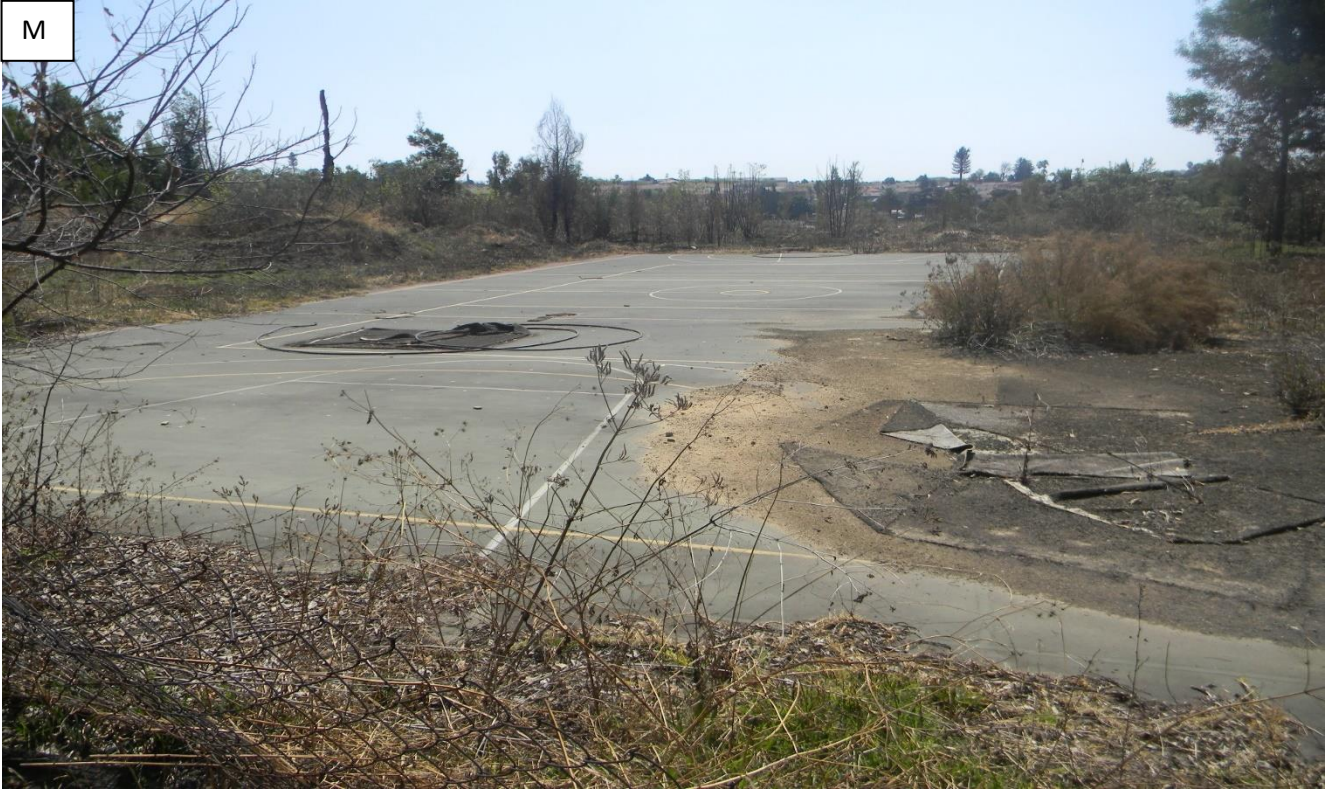
Plate 14: Photo M, Showing dilapidated tennis court within the proposed development site
