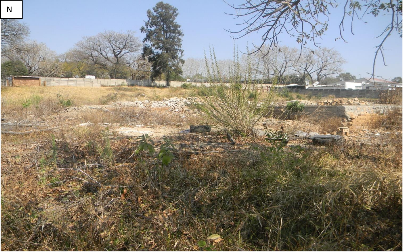
Plate 15: Photo N, Showing derelict structures within the proposed development site.
