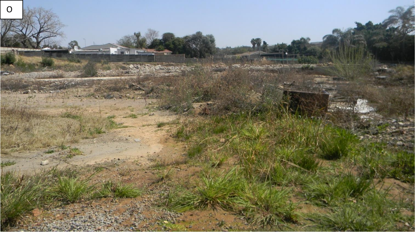
Plate 16: Photo O, Showing derelict structures within the proposed development site.
