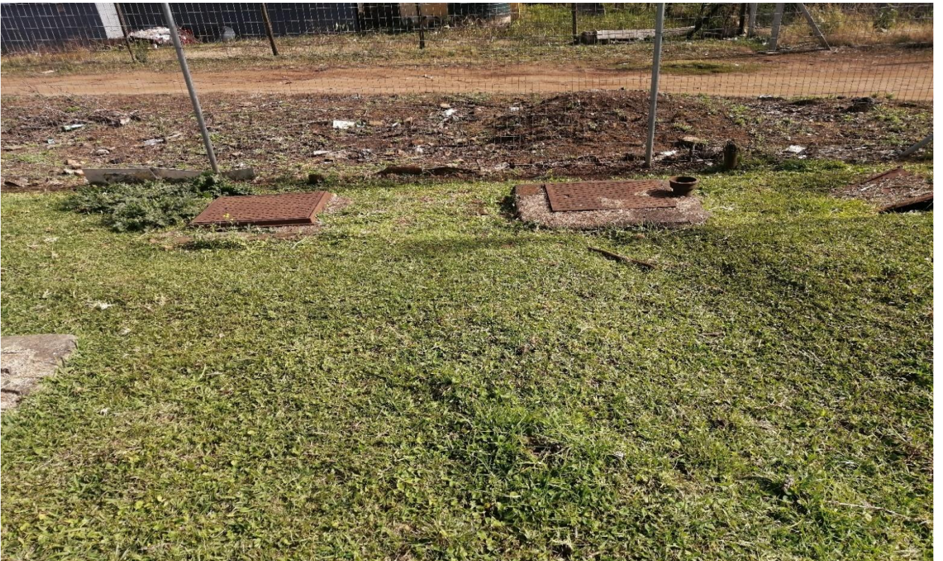
Plate 17: Showing pre existing sewer pipelines.
