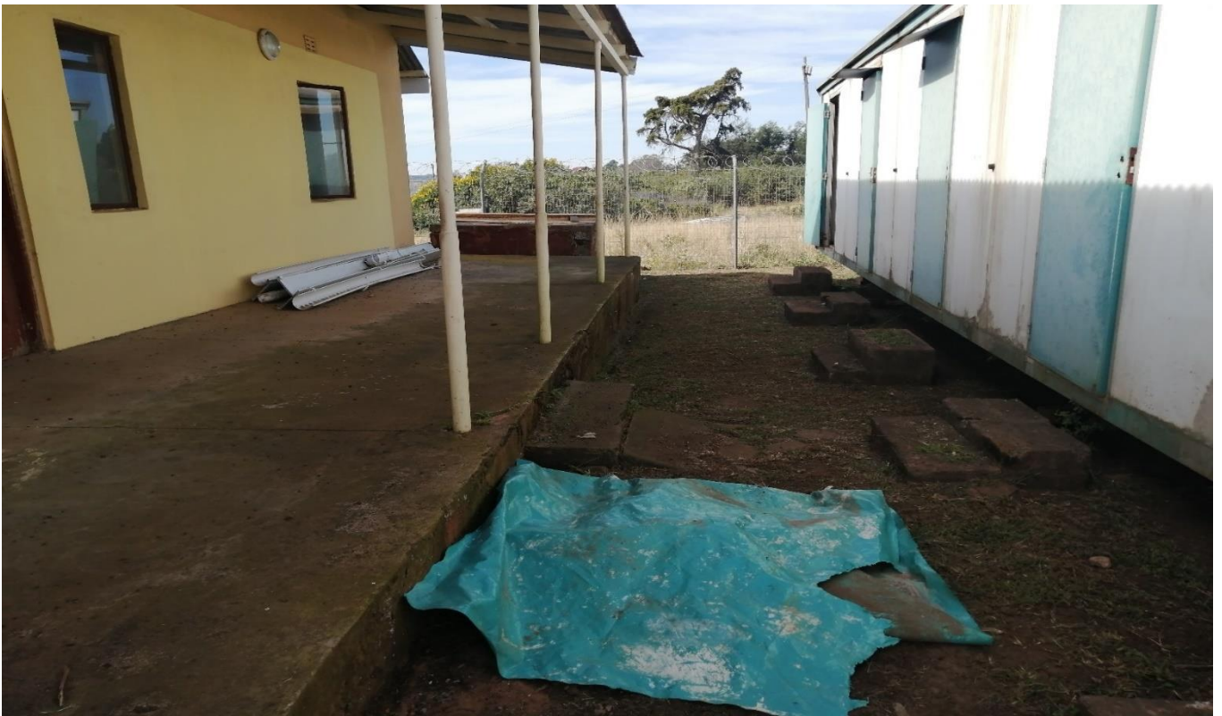
Plate 8: Showing pre existing buildings within the proposed reestablishment development site.
