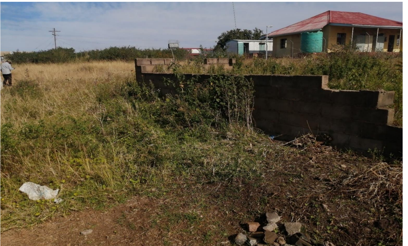
Plate 3: Showing preexisting structures within Saint Faiths Police Station scheduled for reestablishment.
