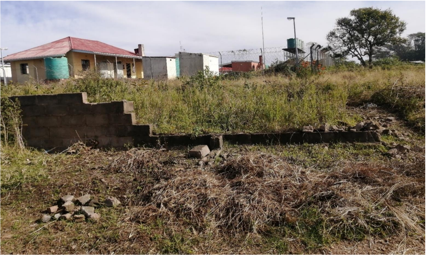
Plate 2: Showing remnants of a building within the proposed development site.
