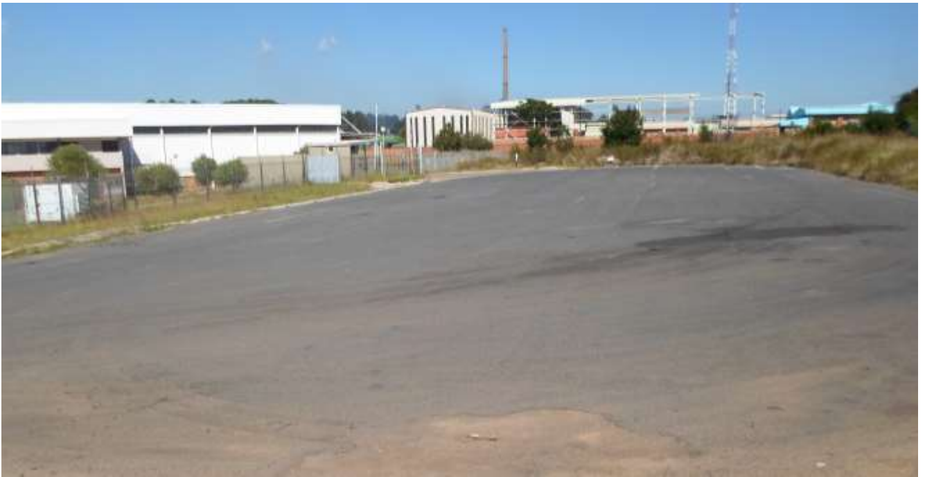
Plate 13: Photo 13: View of access roads and existing buildings within the vicinity of the proposed development site (Photograph © by Author 2022).
