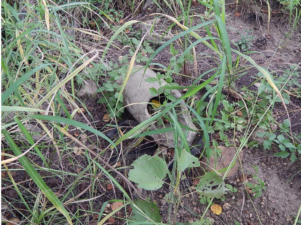
Fig. 13: Recent concrete pipes were observed in the northern section.
