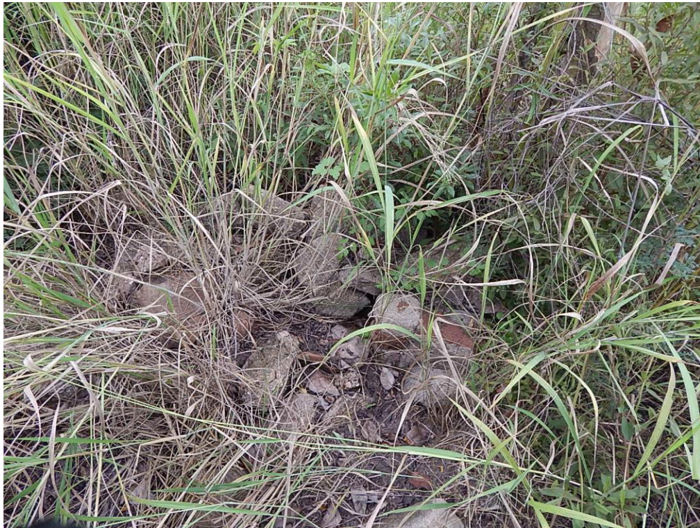
Fig. 12: Recent building rubble (or a possible foundation) was observed in the northern section.
