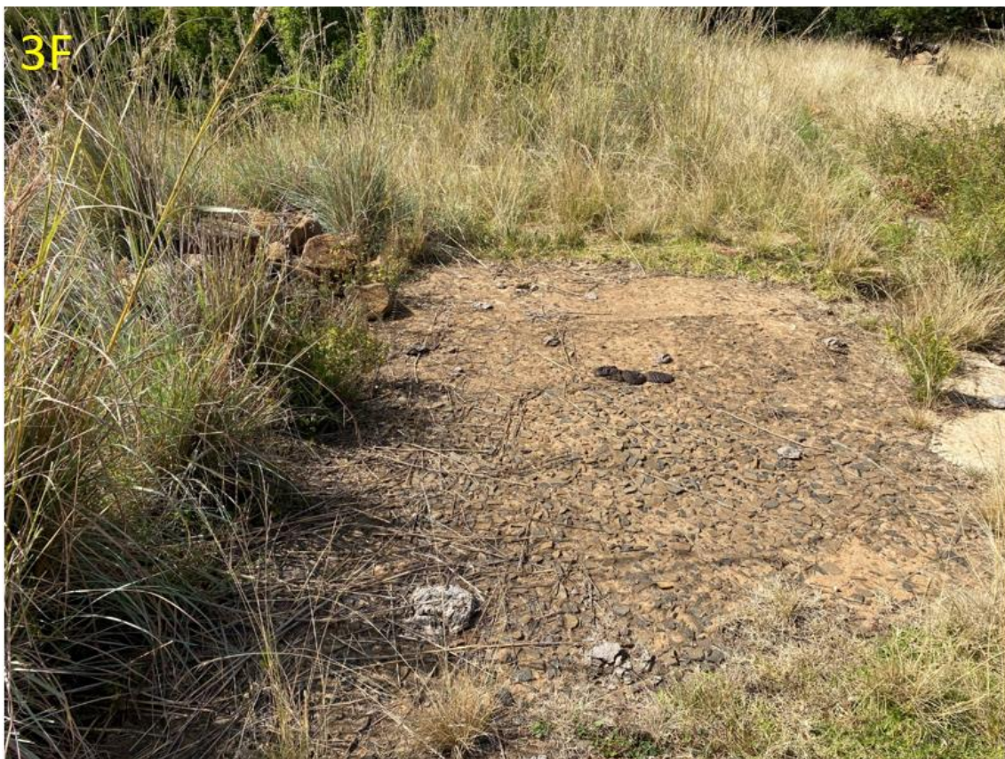
Photograph 18: Foundation of pumphouse (possibly older than 60 years) (3F)
