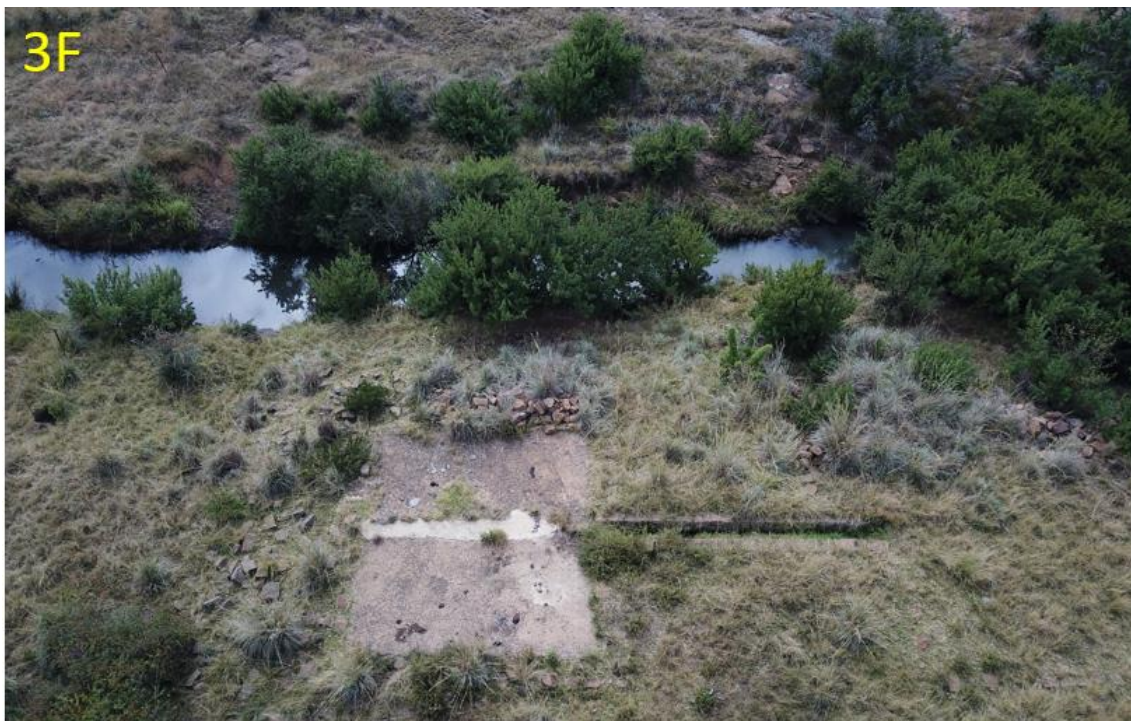
Photograph 17: Foundation of pumphouse (possibly older than 60 years) (3F)
