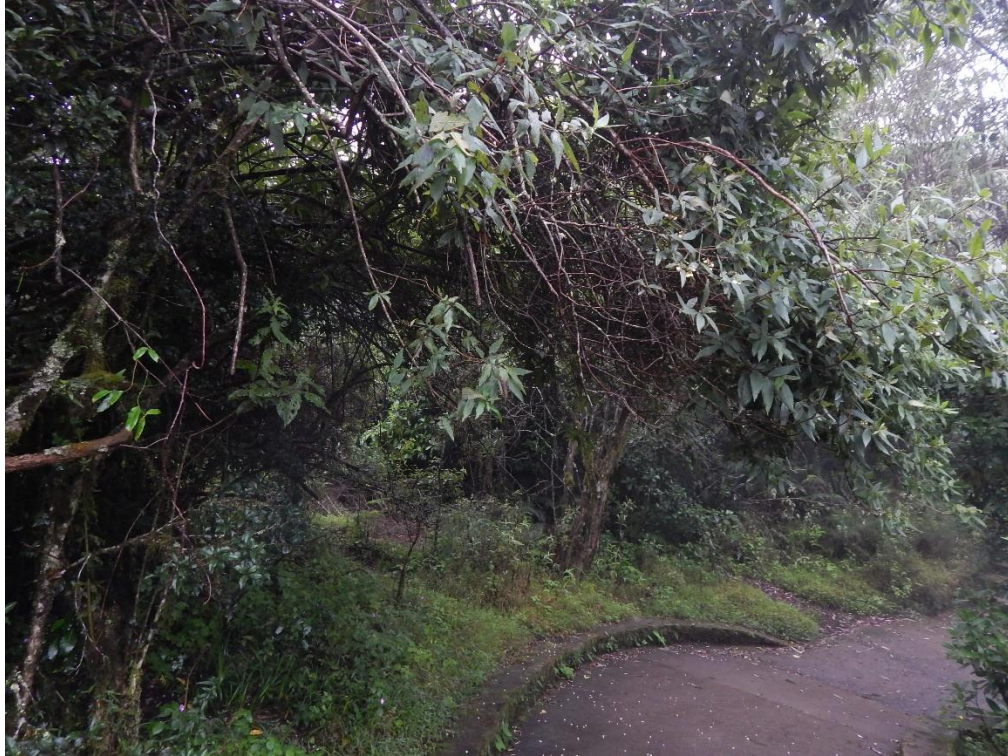
Fig. 11: Existing concrete walkway.
