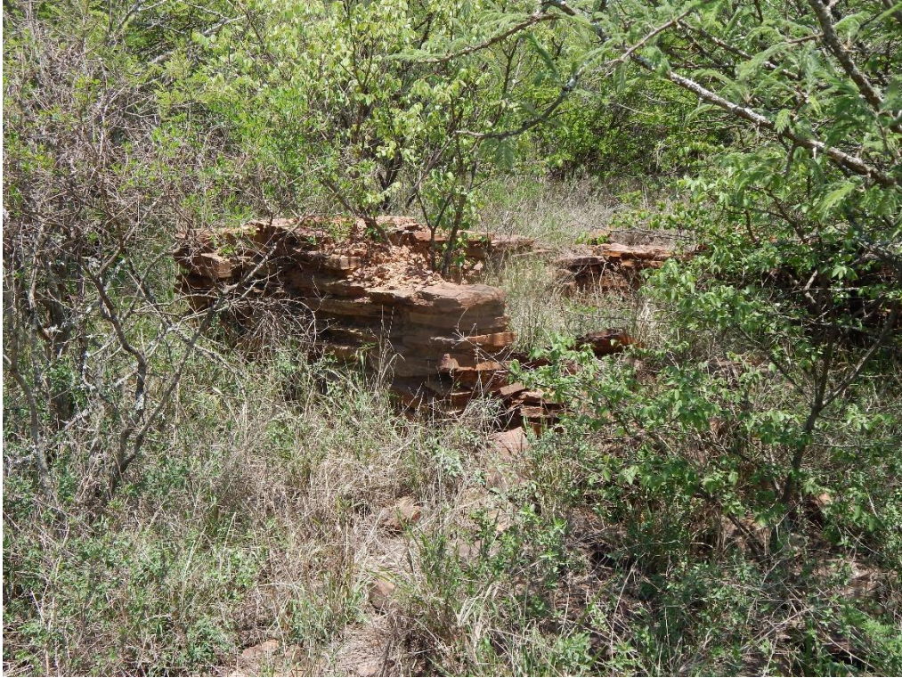
Fig. 11: One of the foundations of a recent house.
