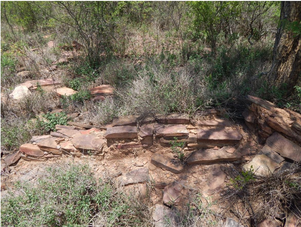
Fig. 10: The foundations of recent workers' houses are visible to the west of the current workers' accommodation.
