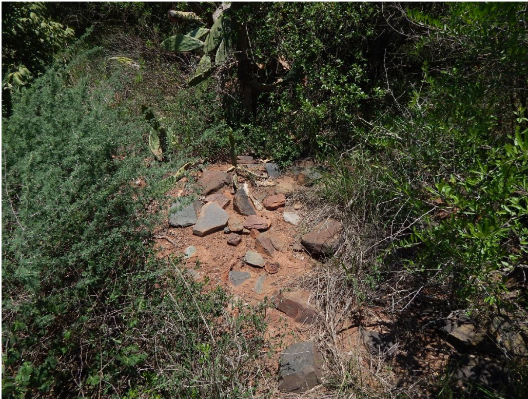
Fig. 14: Disturbed foundations are visible in this area.
