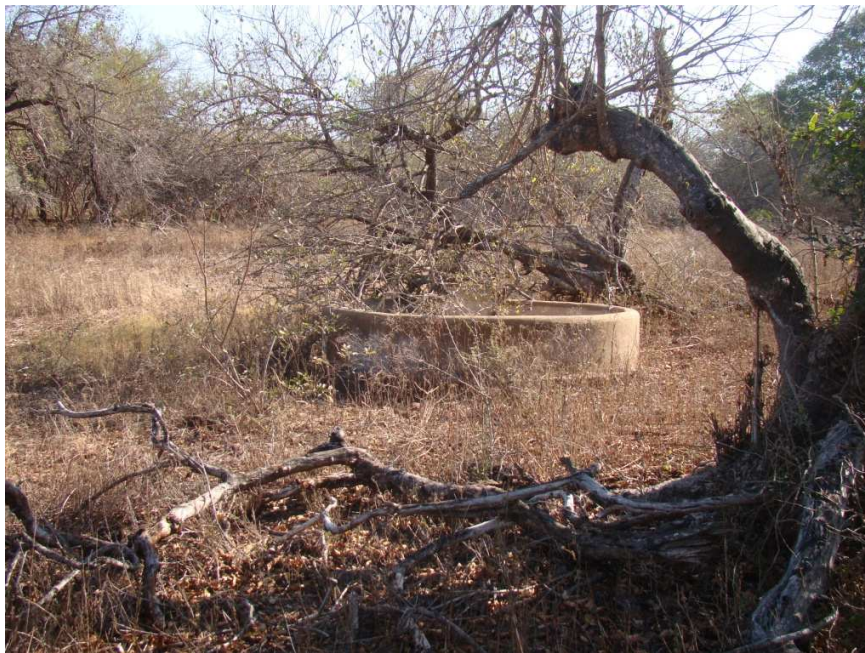
Fig. 20: A small concrete dam is situated close to the pump house and canal.
