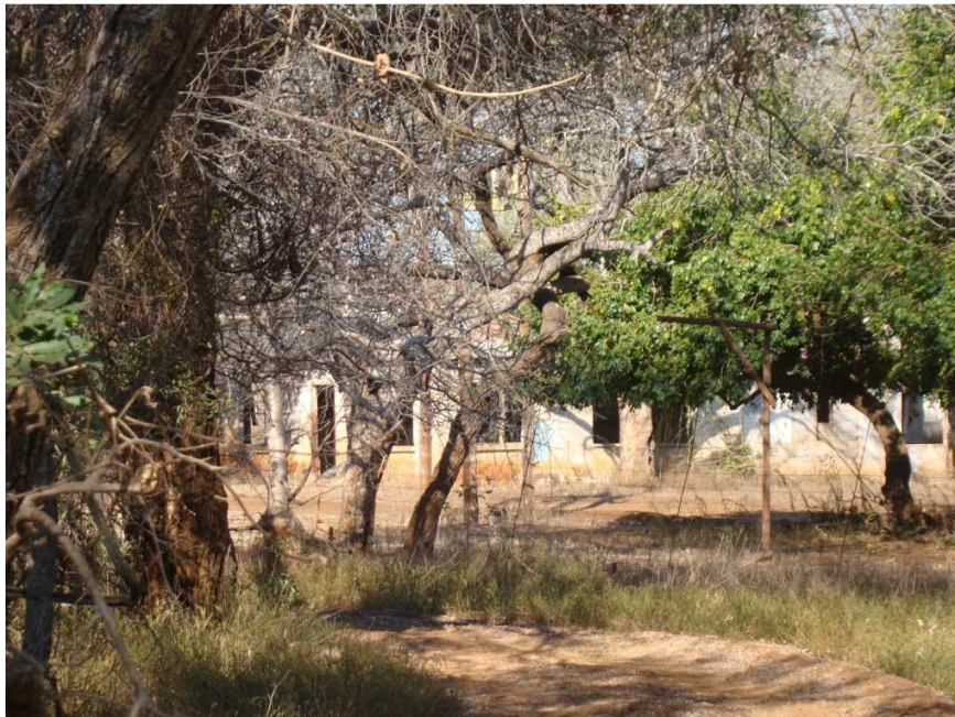
Fig. 22: The farm infrastructure as mentioned above is associated with an old farm house. This ruin is not within the Herculina study area.
