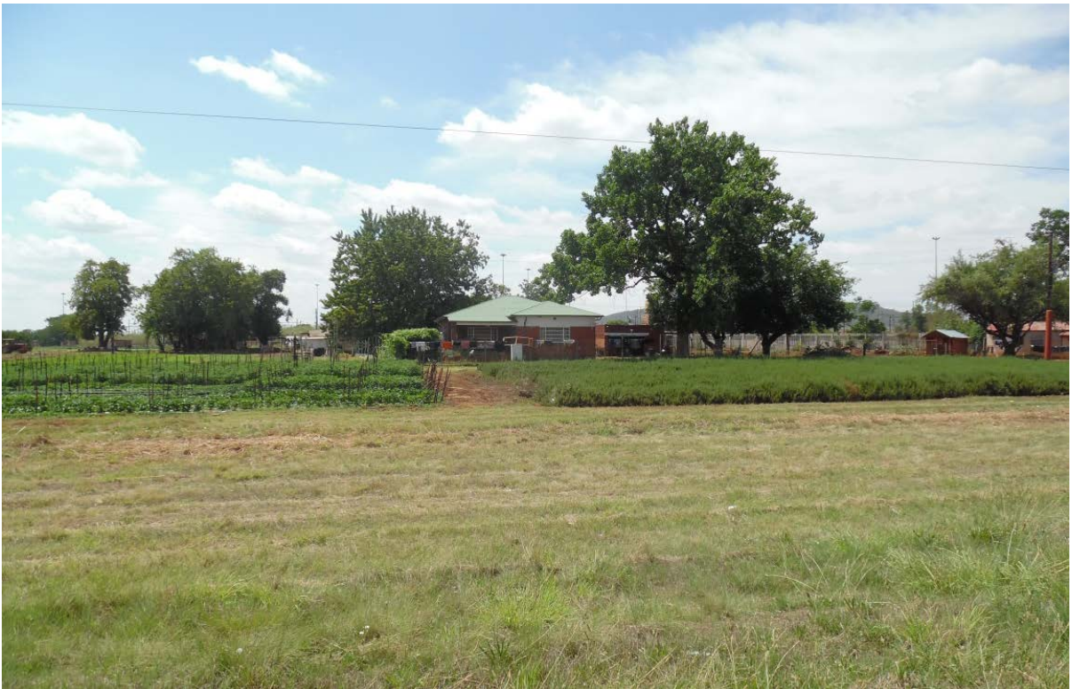
Figure 15: Structures older than 60 years
