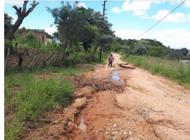
Figs. 1 – 6: The general condition of the informal roads is severely eroded and flooded in places. The upgrading of the roads will ensure accessibility to the residential area (courtesy AFRIKA Enviro & Biology).
