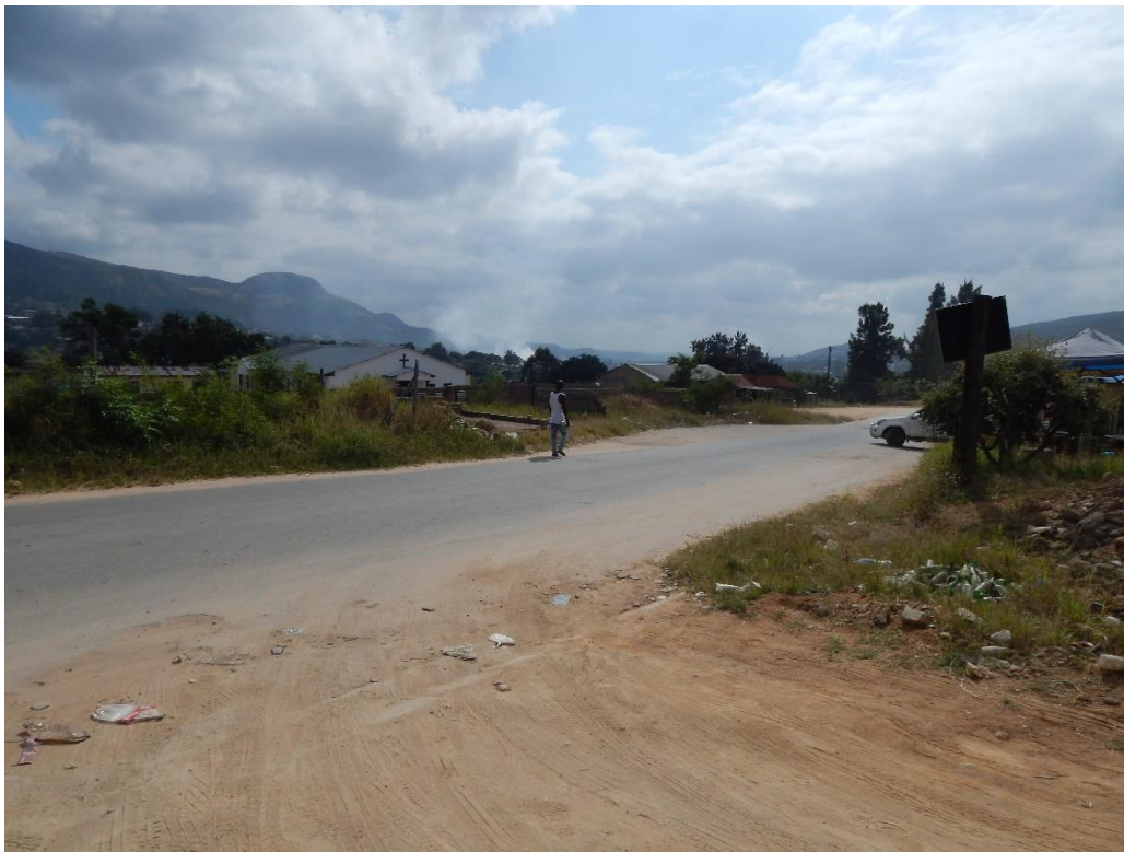
Fig. 29: The planned upgrading of the informal roads will stop here at the tarred road (point C).
