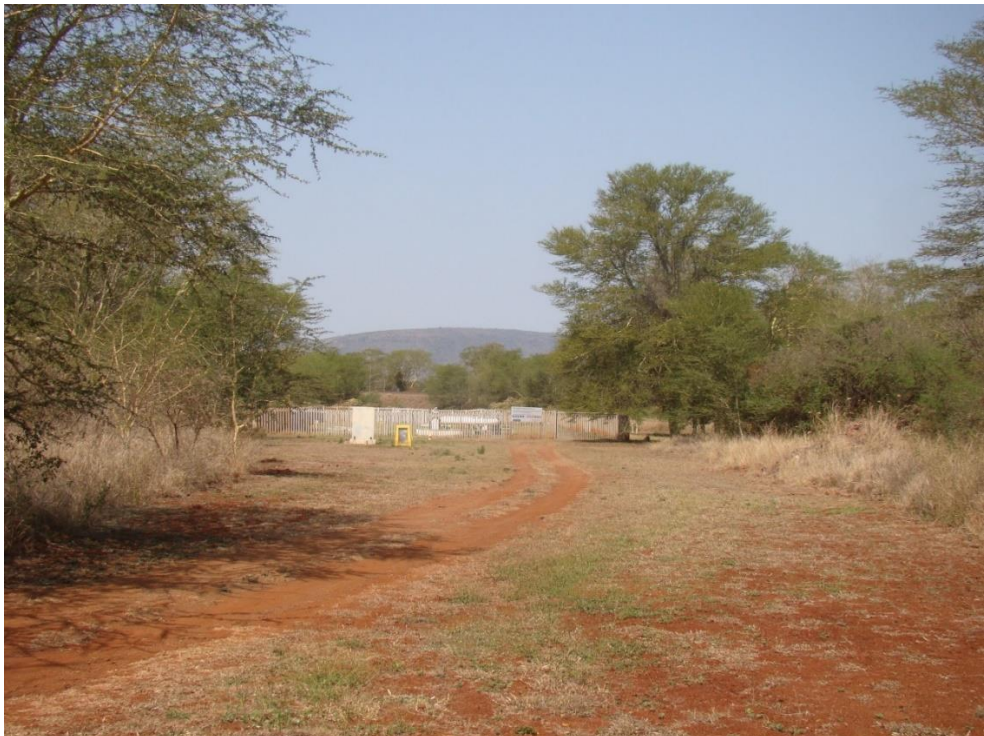
Fig. 10: The SASOL gas pipeline pump station .
