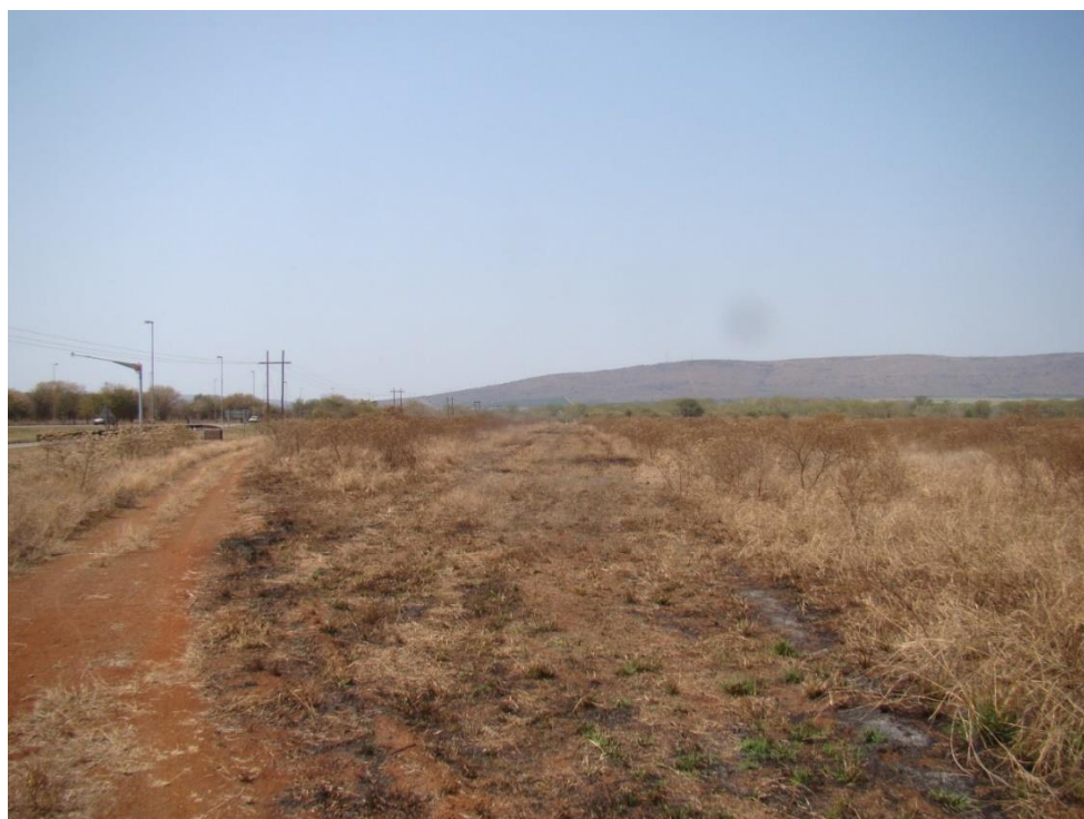
Fig. 4: View to the east in the path of the SASOL gas pipeline. The N4 is to the left and a fallow sugarcane field to the right. The area was burnt.
