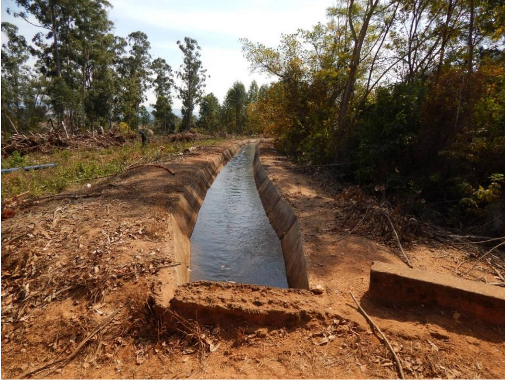
Fig. 19: The original earth Canal was lined with concrete during the 1960's.
