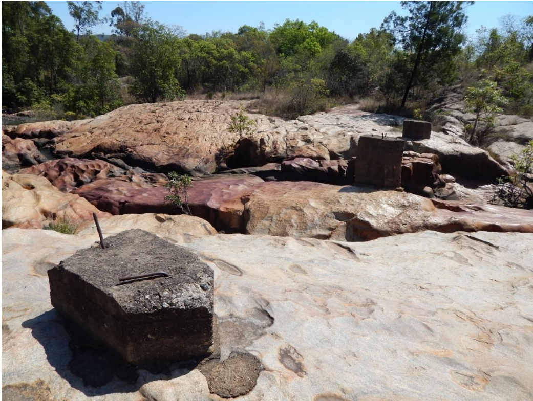
Fig. 18: Concrete supports (Mill infrastructure), are still visible in the river.
