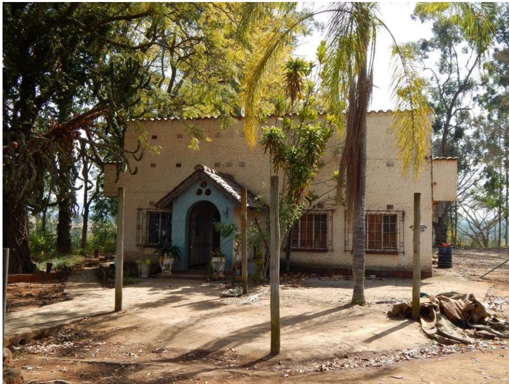
Fig.14: The historic (1910) farmhouse which was altered and compromised during the early 1970's by Mr. Beckenstrater (Sr).
