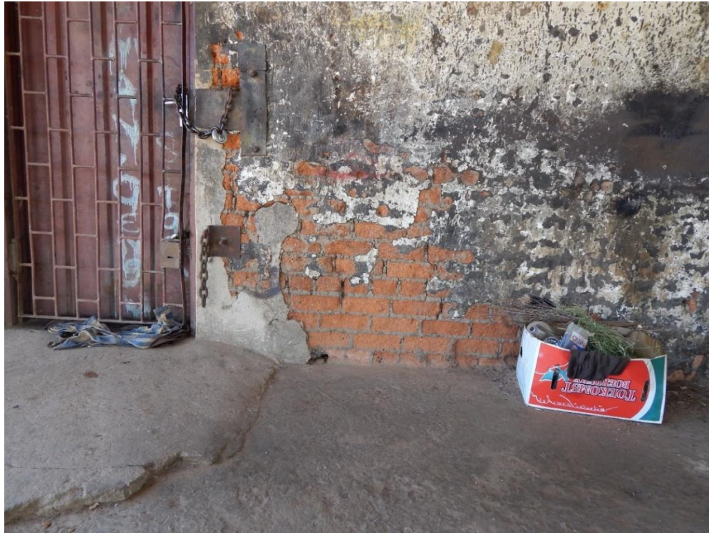
Fig. 16: The structure was originally built with baked bricks. It was changed to be used as a workshop in later years.
