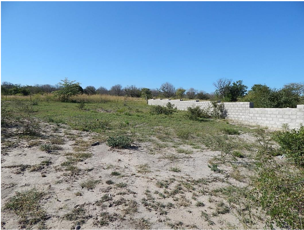
Fig. 6: The south-eastern section with the concrete border wall, visible.
