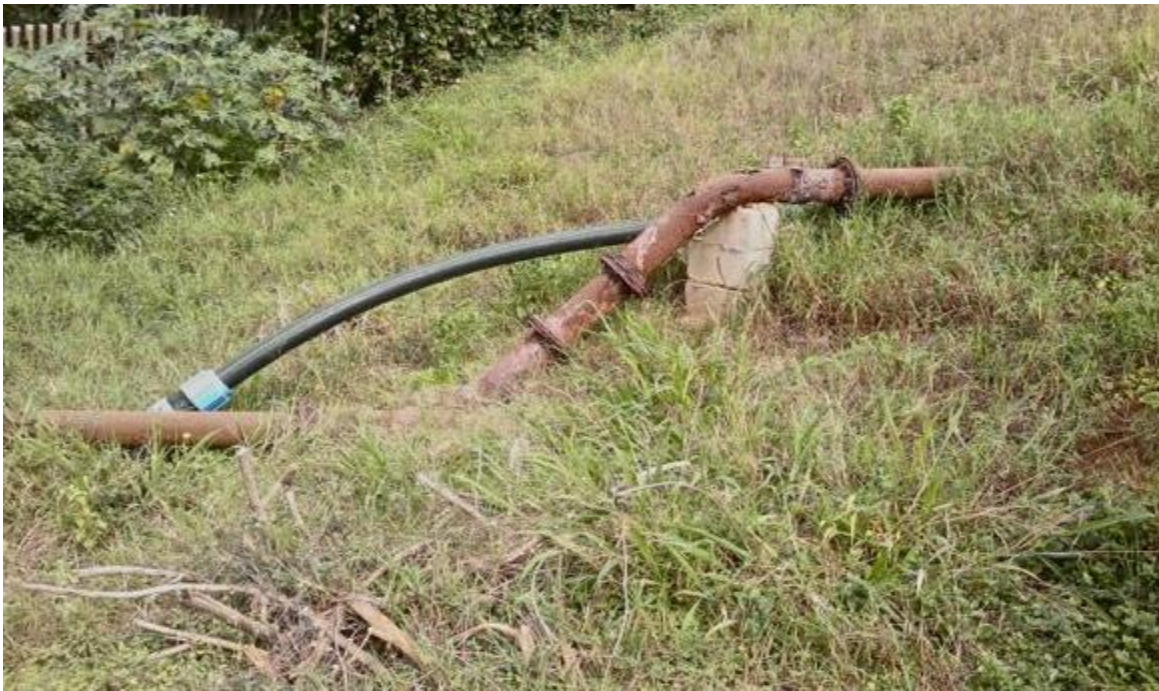
Figure 6: Old water or sewerage pipeline
