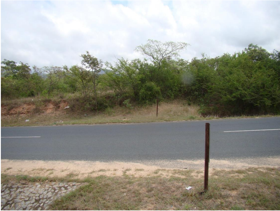
Fig. 11: The road reserve where the line will cross the tarred road at an existing culvert.
