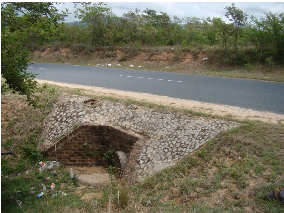
Fig. 12: The culvert where the line will cross underneath the tarred road.
