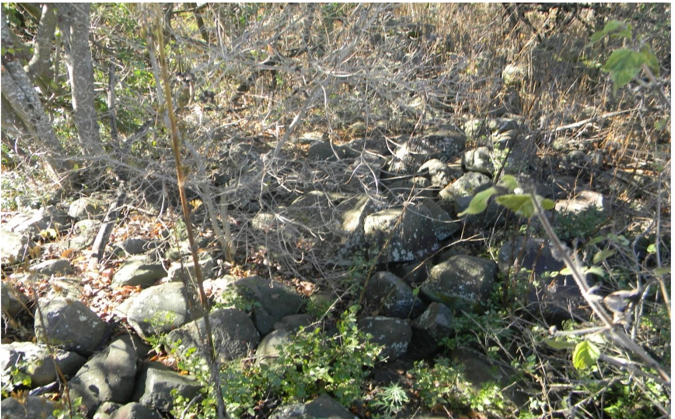
Plate 45: showing surviving walls of the Angolo Boer War Fortress of Ngisana.
