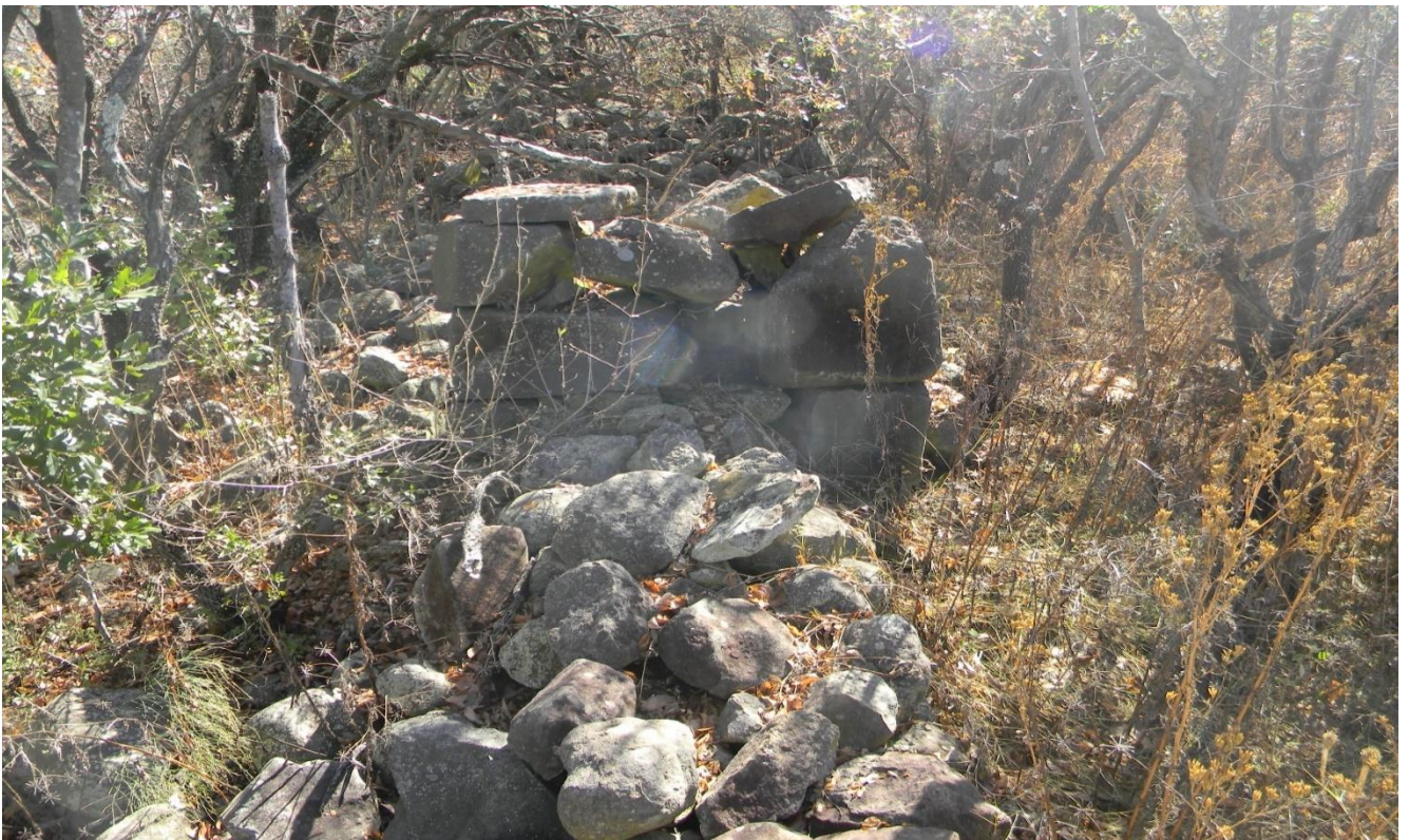
Plate 50: showing spectacular walls at the Boer Fortress.
