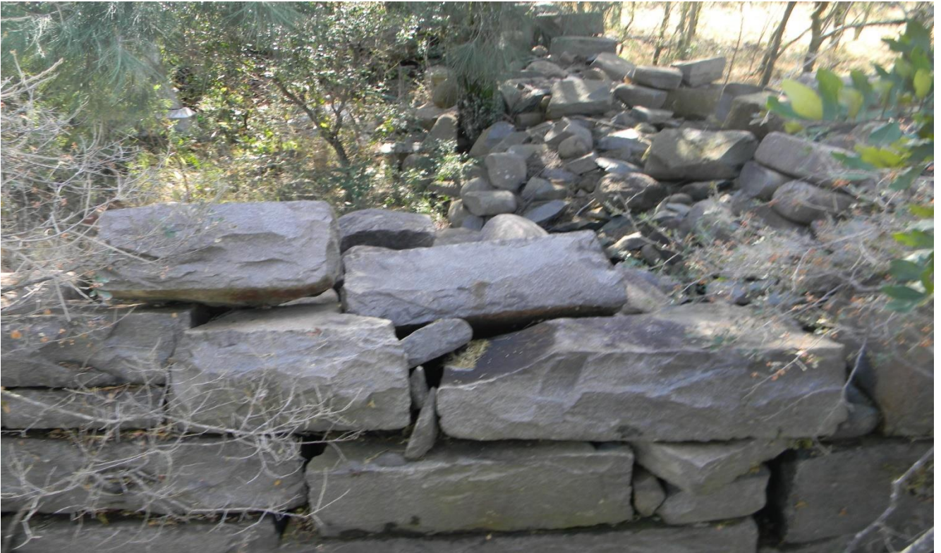
Plate 21: showing sections of the stone walled enclosure at the De Waal Family cemetery.
