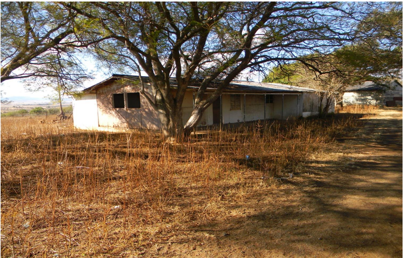
Plate 55: showing farm house which is probably more than 60 years old.
