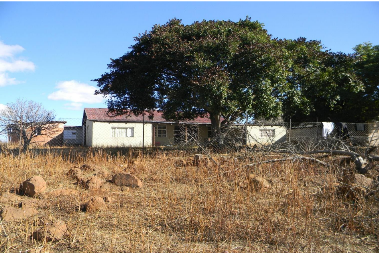
Plate 58: showing farm house which is probably more than 60 years old.
