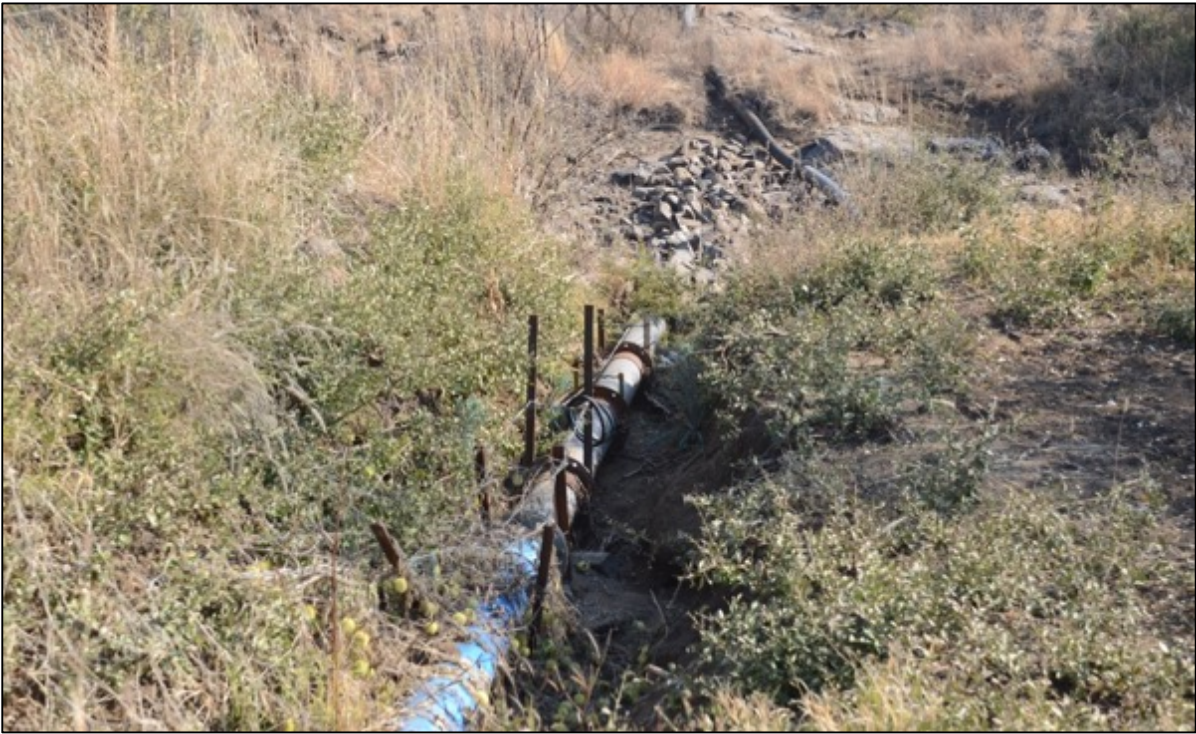
Figure 15. Pipeline at the Crossing Point
