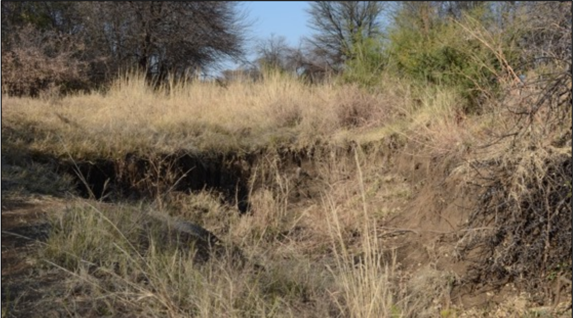
Figure 13. Groundworks at Bierspruit
