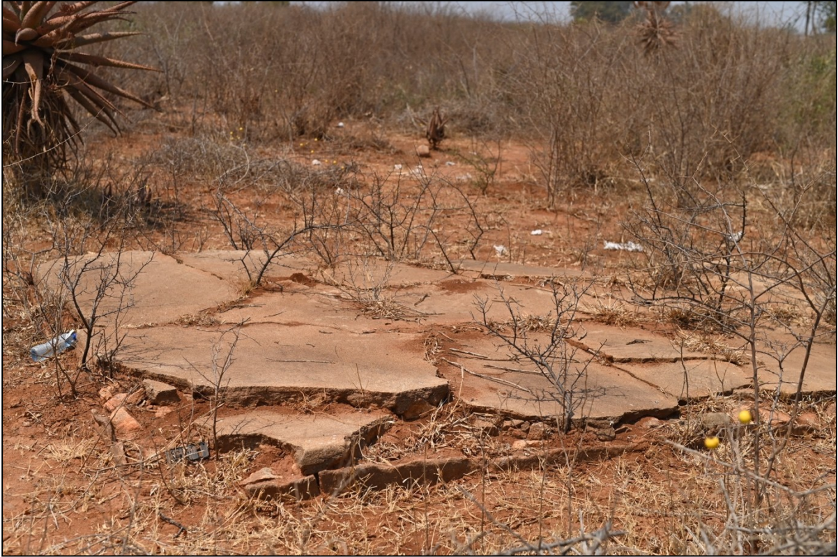
Figure 6. Cement foundations observed on site
