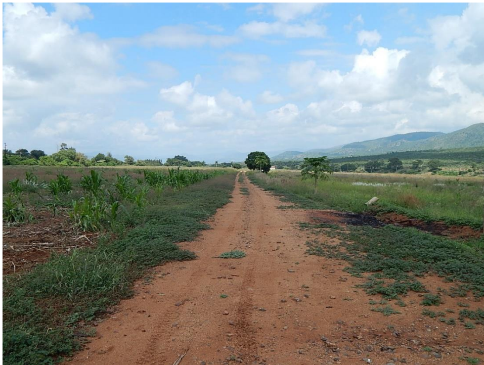
Fig. 12: Another view of the middle section facing west, the earth canal is to the right of the road.
