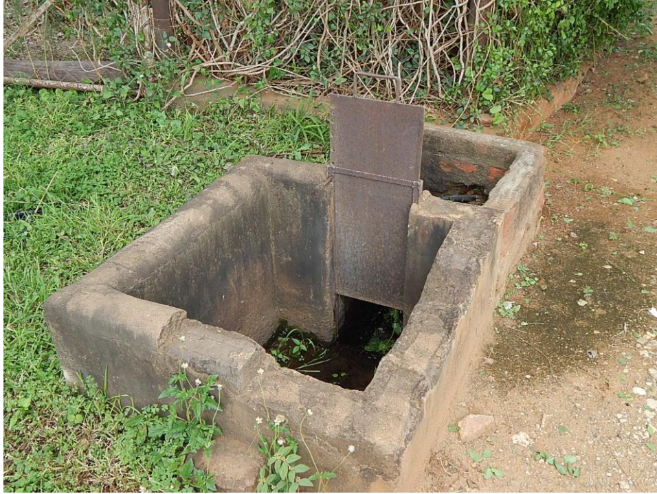
Fig. 23: A few small weirs are visible near the farm residence, to regulate water into the canals.
