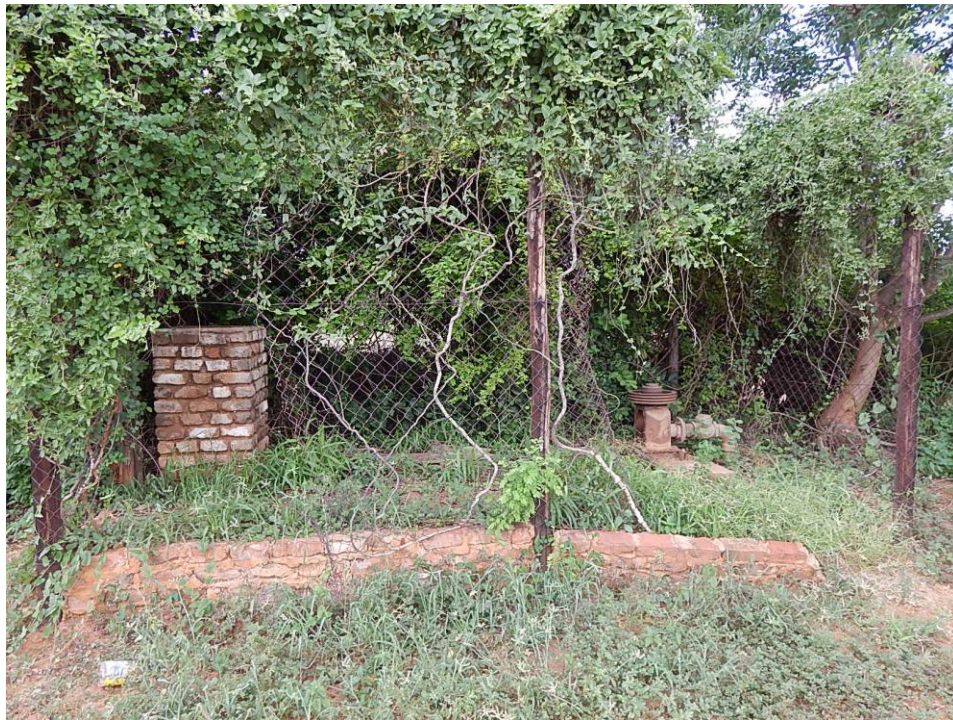
Fig. 20: The infrastructure of a water pump.
