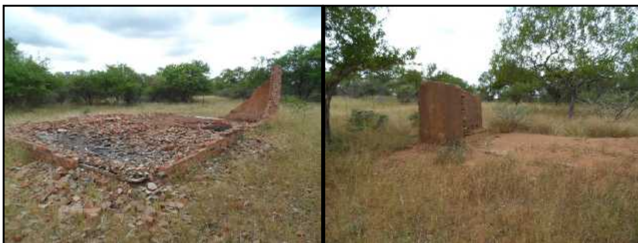
Figure 48- Pictures showing the two structures forming site MB-22. Left is a red refractory brick and right mud bricks.
