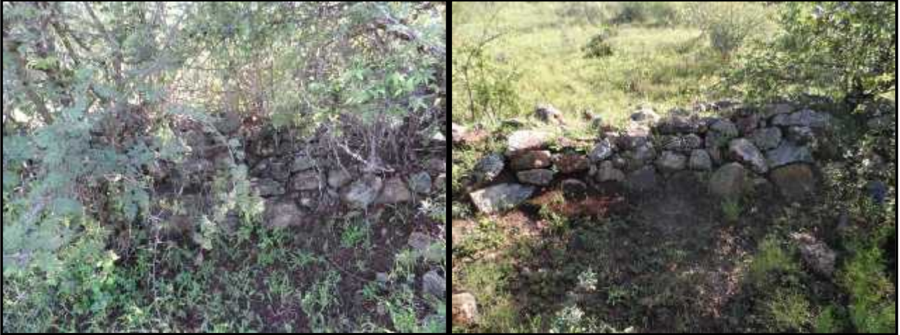
Figure 75- Remaining walls of the big kraal
