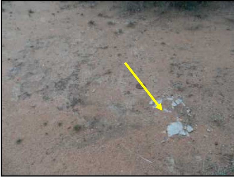
Figure 46- Daga floor with ruminant of cement (yellow arrow).
