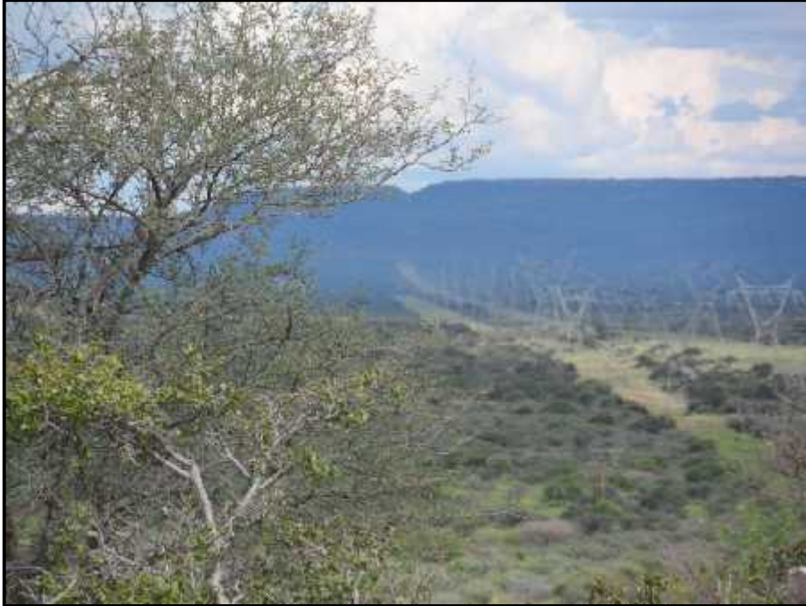
Figure 10 -Eskom transmission corridor.
