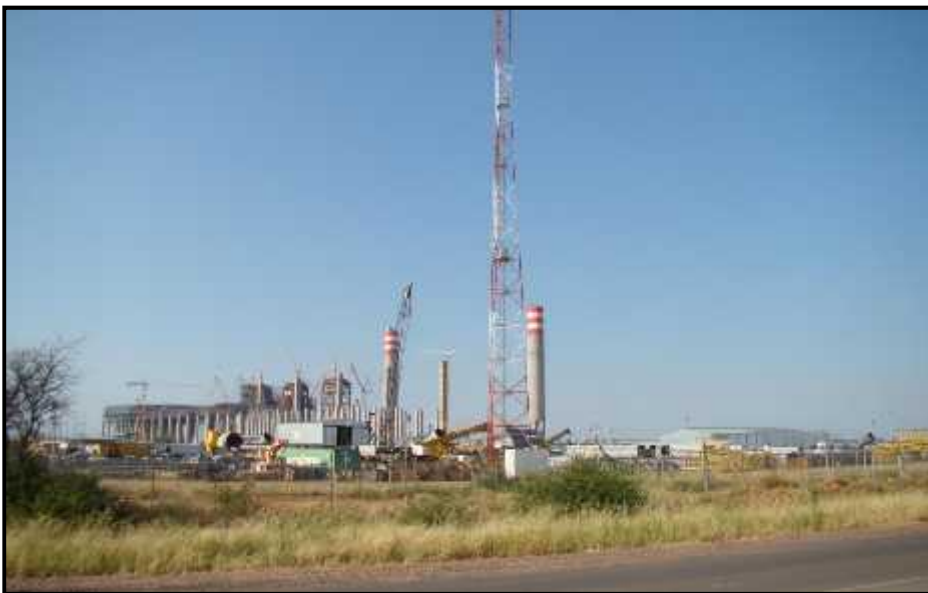
Figure 9-Construction activities at Medupi Power Station.@ Murimbika and Tomose, 2012.
