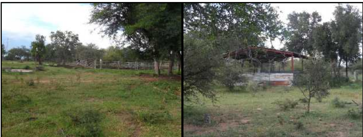
Figure 36 - Cattle loading ramp and fence. Steel and corrugated IRB iron sheet shed
