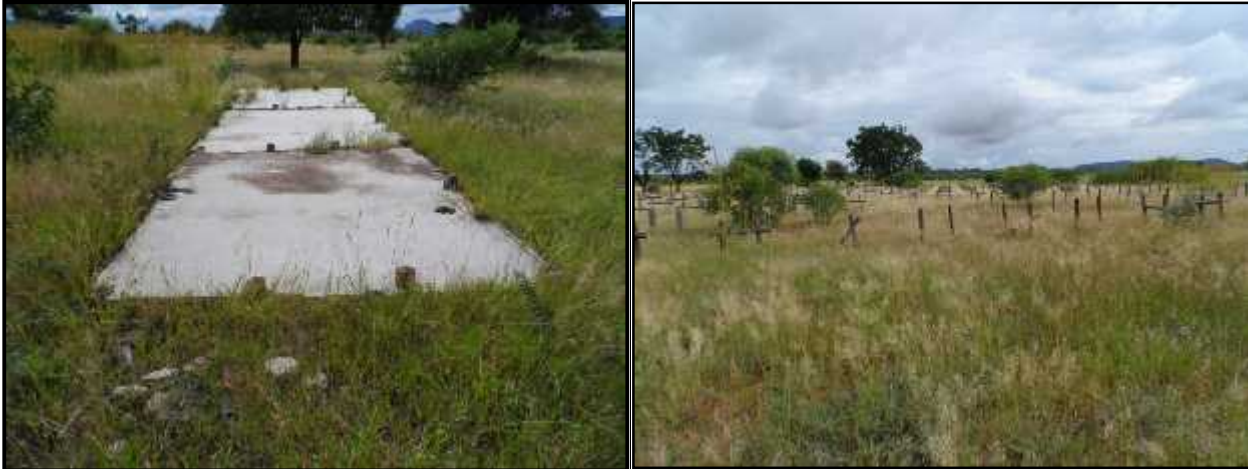
Figure 63 - Shed foundation and pole structure either to hag stuff or support plant life
