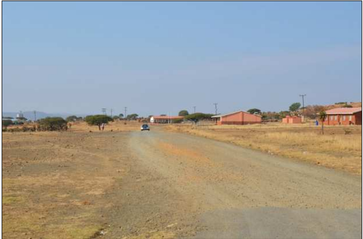
Figure 3. Road upgrade start
