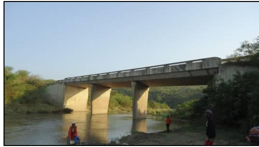
Fig 25 Bridge on R 61 over the river
