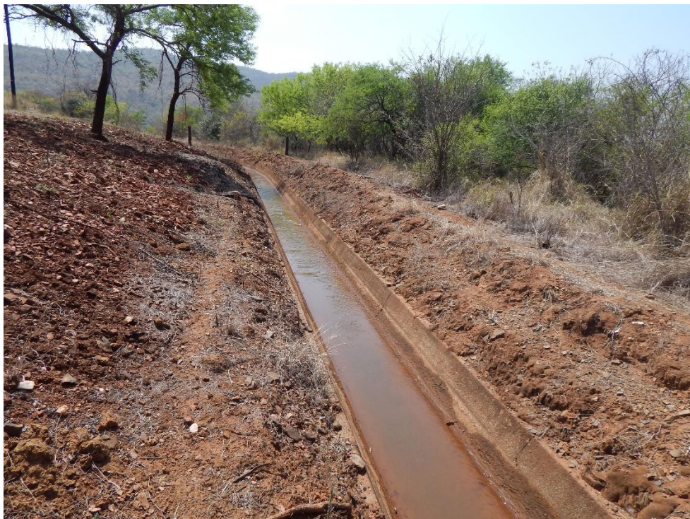
Fig. 42: Another view of the concrete water canal.
