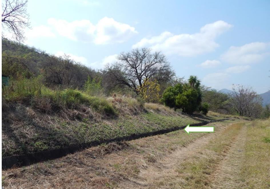
Fig. 7: A long concrete water canal forms the southern boundary of study area 1.
