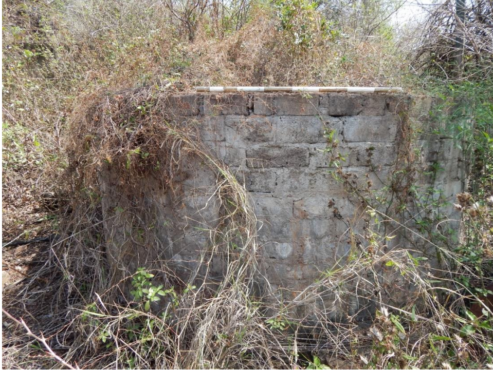
Fig. 21: Concrete / brick water tanks were observed in the eastern section of the study area. Water for the Clinic, was supplied from here in the past.
