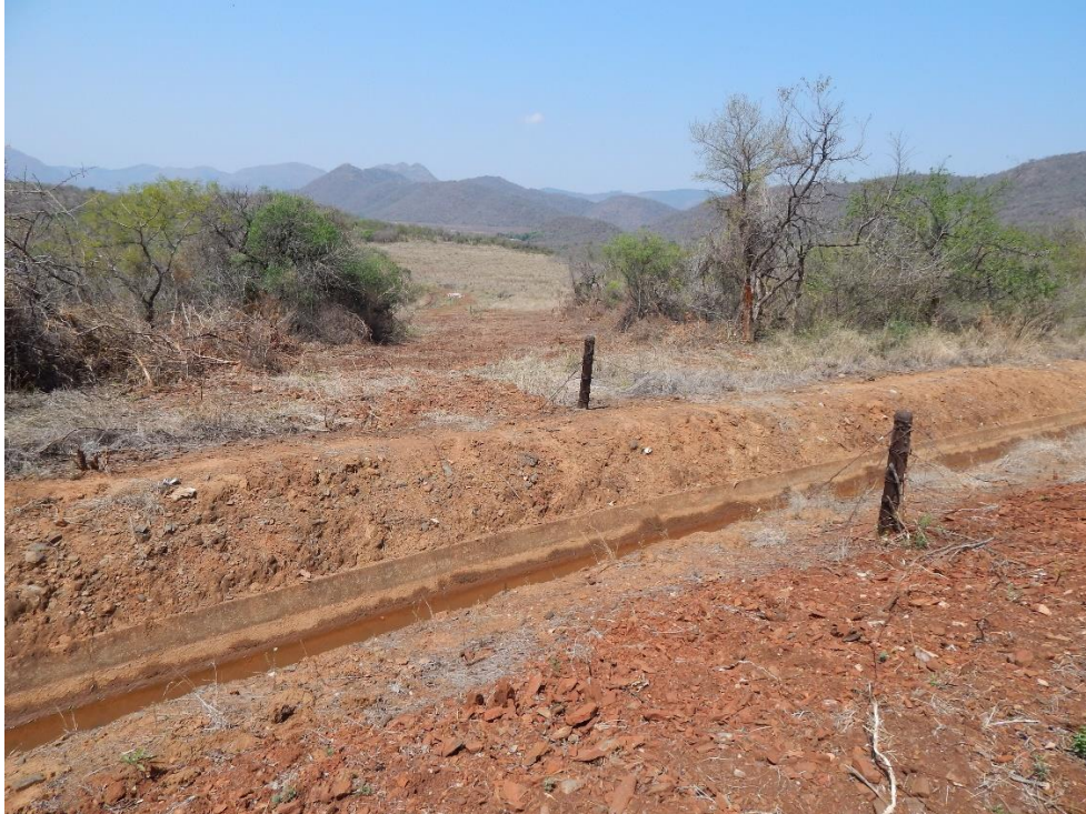
Fig. 41: A concrete water canal cuts through this section in the east. View towards the eastern boundary.
