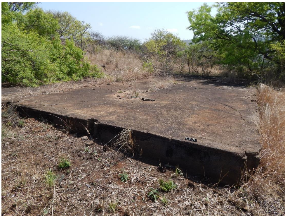
Fig. 35: The foundations of an old sawmill, which burnt down in the 1980's.
