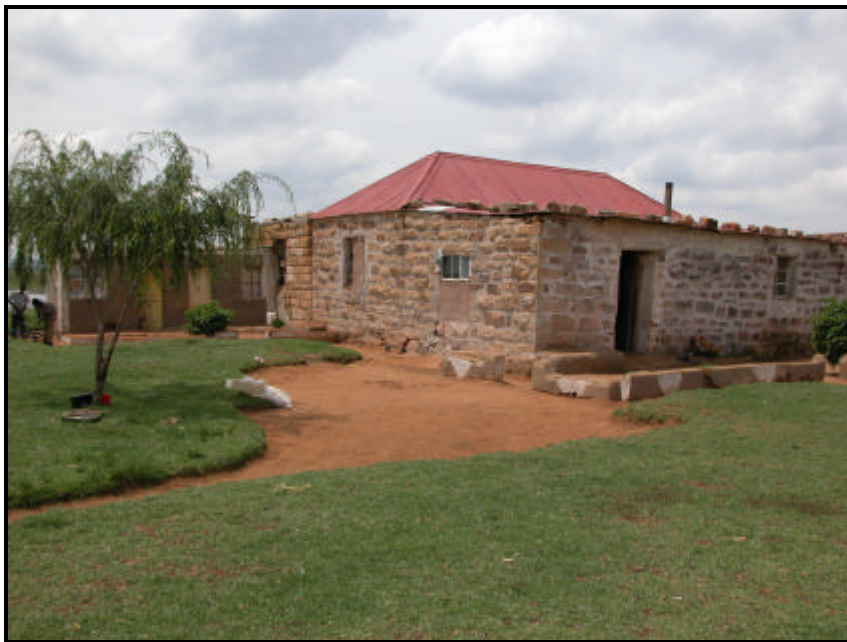
Figure 15 – Historic farmhouse with additions
