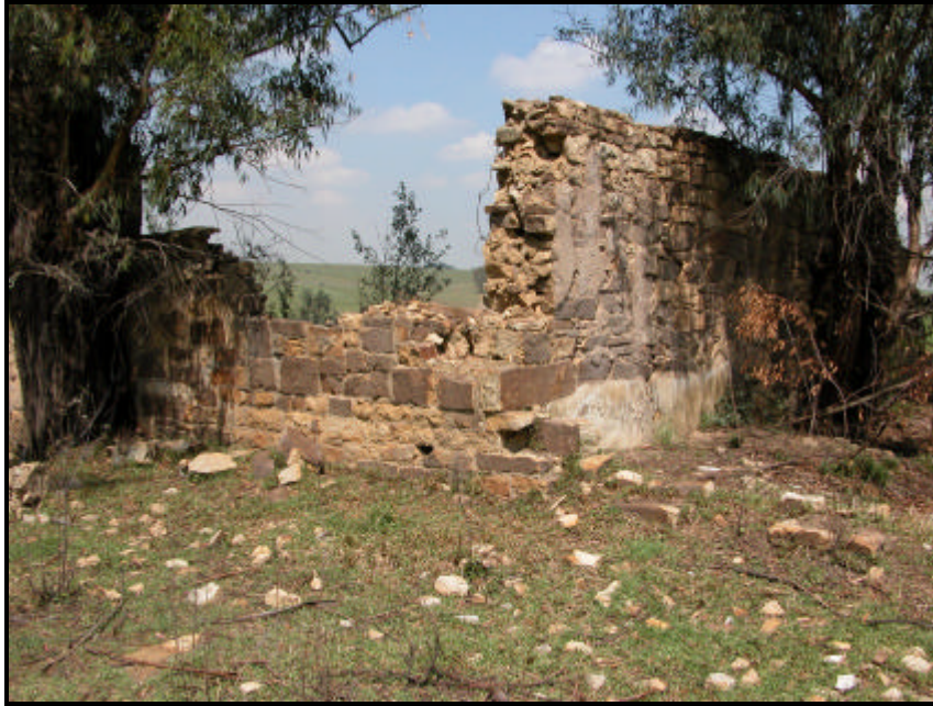
Figure – Stone outbuilding
