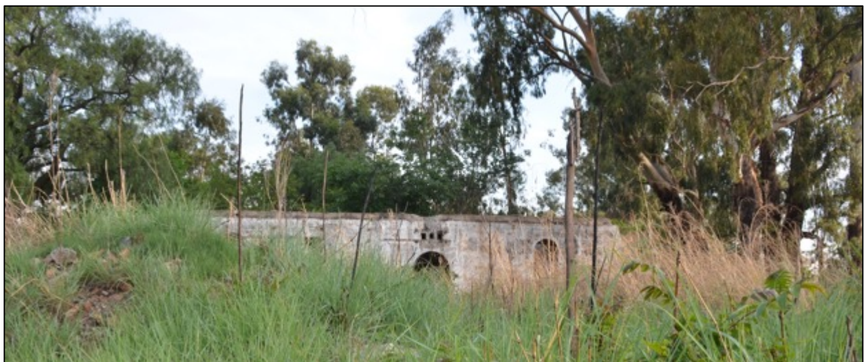
Figure 18. Historic mining structures on site
