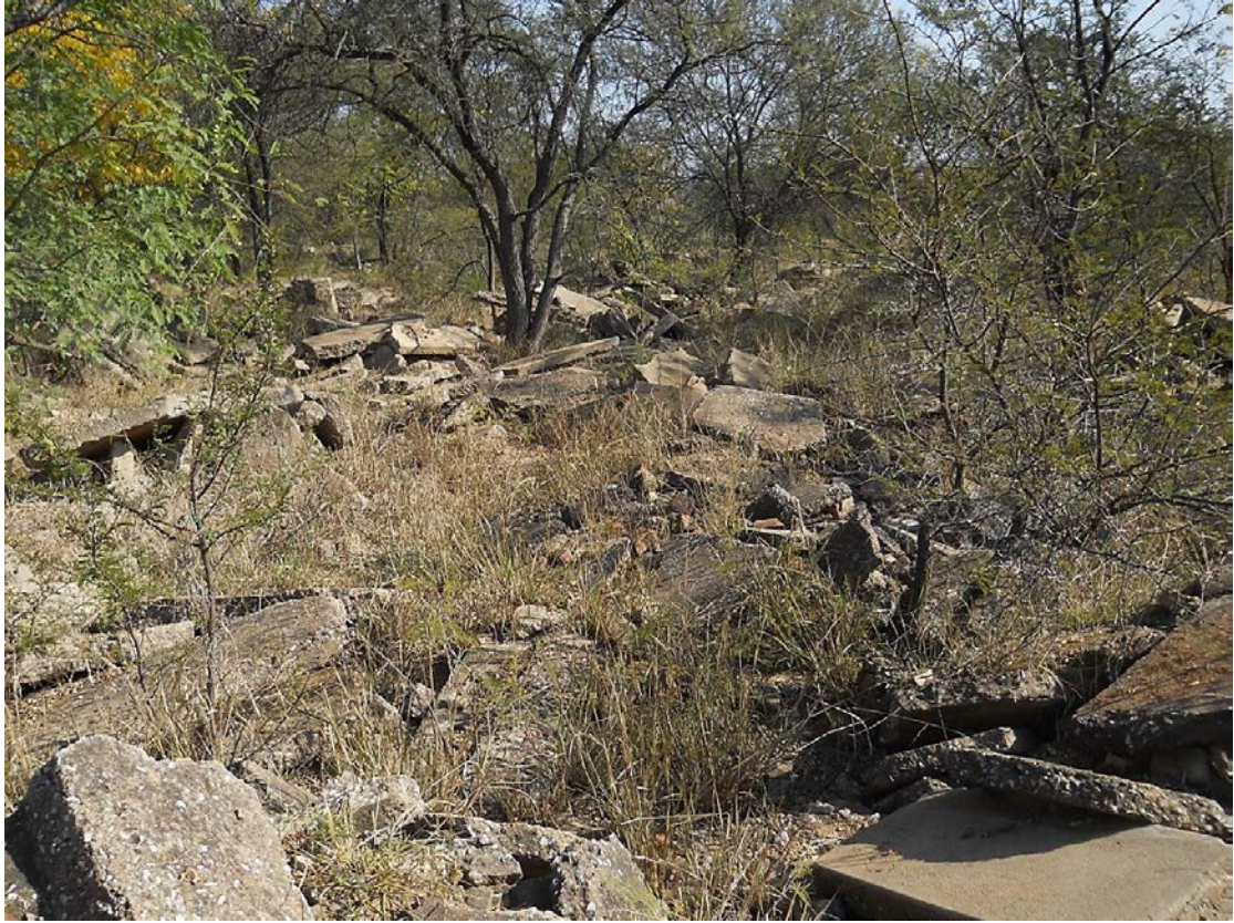
Figure 1. View of dumped building rubble which virtually covers the entire project area.
