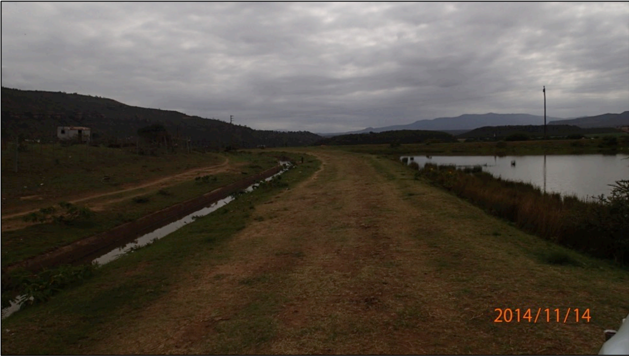
Figure 15. Nokopela Road Upgrade Section 2 (road along the Water Canal)
