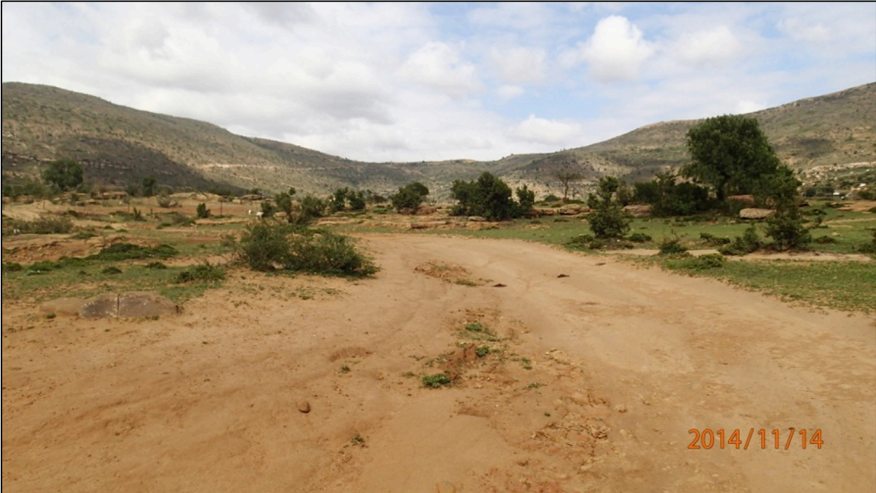
Figure 14. Nokopela Road Upgrade Section 1: End
