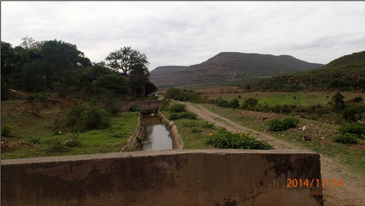
Figure 17. Nokopela Road Upgrade Section 2 (Water Canal)
