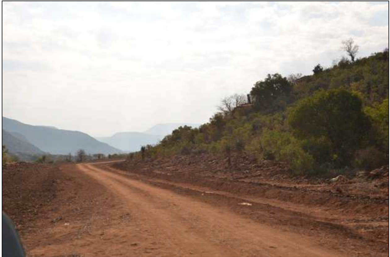
Figure 3. Areas of road already under construction
