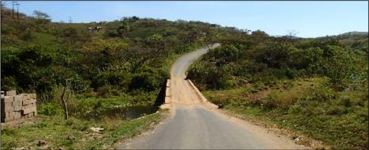
Figure 6. Bridge at the coordinates S29° 04' 56.64" E31°21' 09.67"
