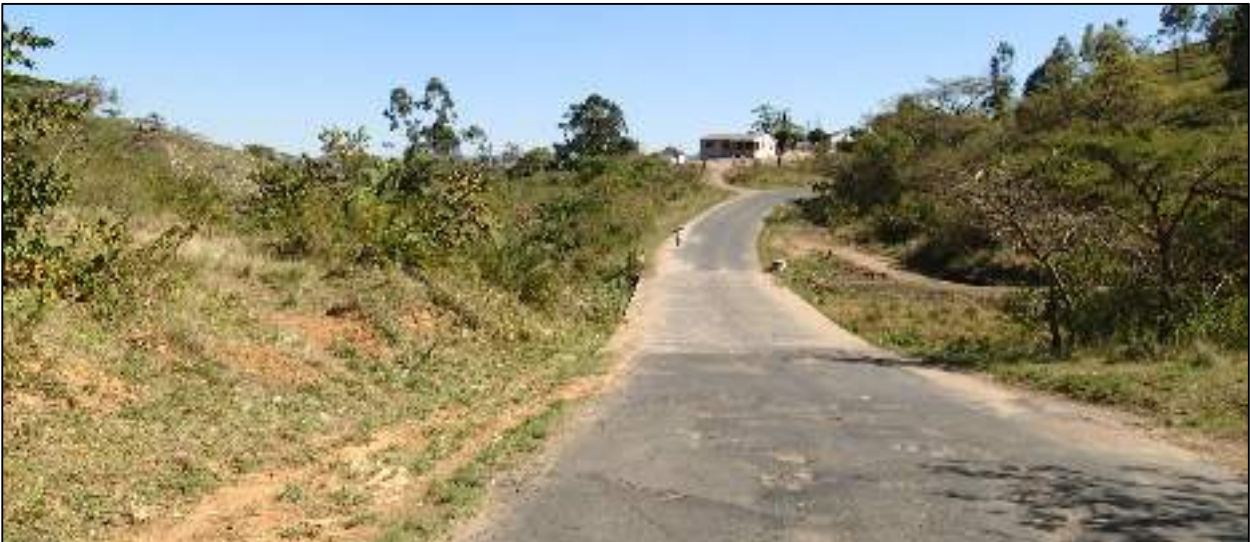
Figure 5. Bridge at the coordinates S29° 05' 14.13" E31°21' 16.53"
