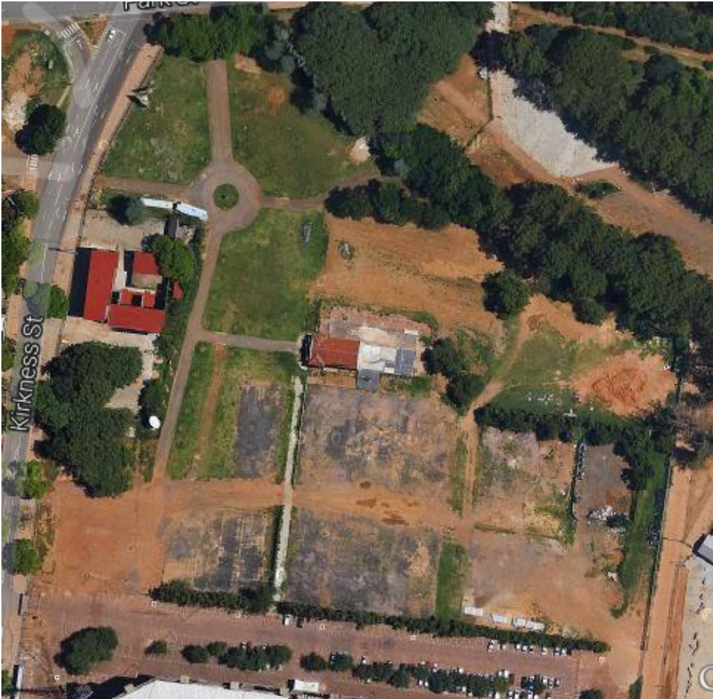
Figure 17 Current state of the playing fields. The outline of the spatial structure can be discerned, partly due to still extant retaining walls. (Google Earth)
