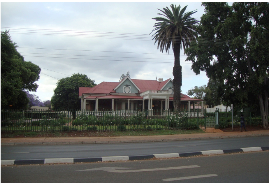
Figure 21 Kingston House, located on the corner of Kirkness and Park Streets.
