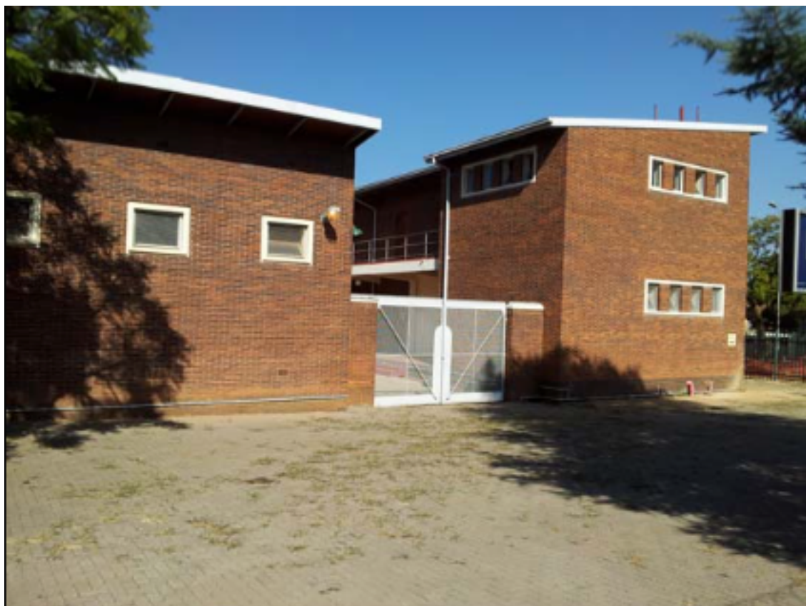
Figure 28 The Loftus Substation (FP Coetzee, 2012)
