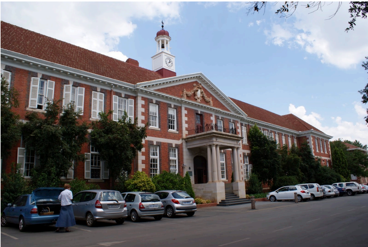
Figure 25 The main building of the Pretoria High School for Girls
