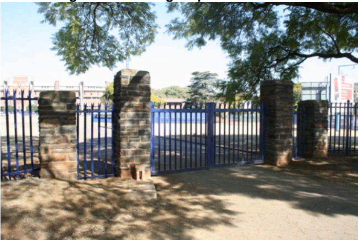
Figure 44 The posts of the gates to the sports fields on Park Street, just off the corner of Kirkness Street.
