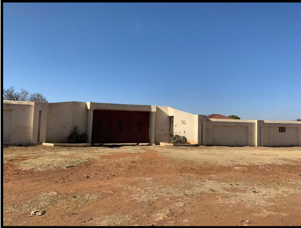
Photograph 2: General area where Water Pipe Line will be situated
