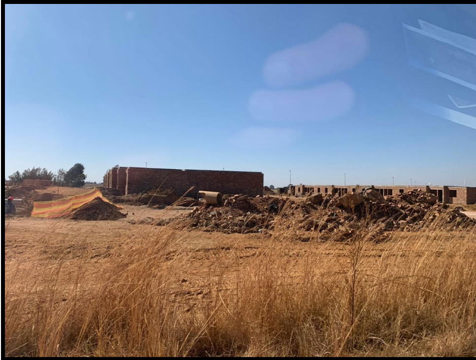
Photograph 6: General area where Water Pipe Line will be situated
