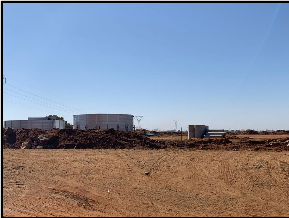
Photograph 5: General area where water Pipe Line will be situated
