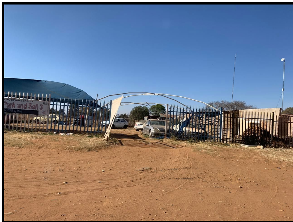
Photograph 1: General area where Water Pipe line will be situated
