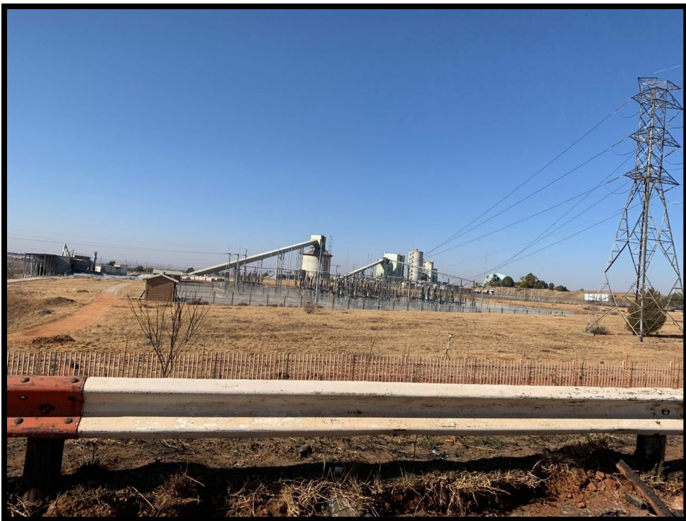
Photograph 13: General area where Water Pipe Line will be situated
