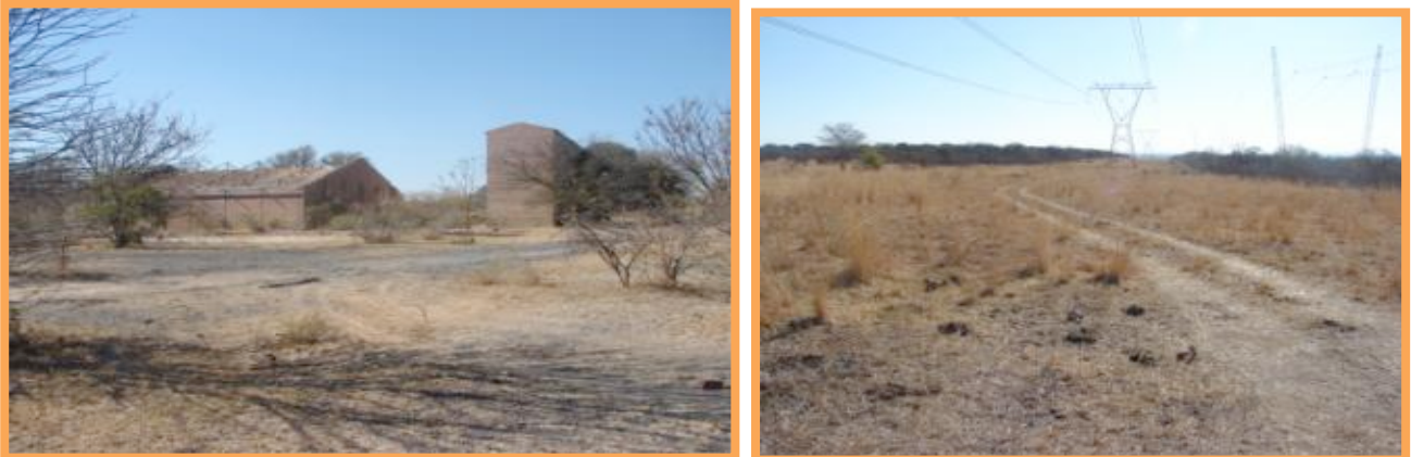
Plates 10 and 11: Pictorial views of dilapidated farm infrastructure near alternative Platreef powerline route (Left) and the terminal position of the proposed powerline route at the proposed Borutho Substation site (Right).
