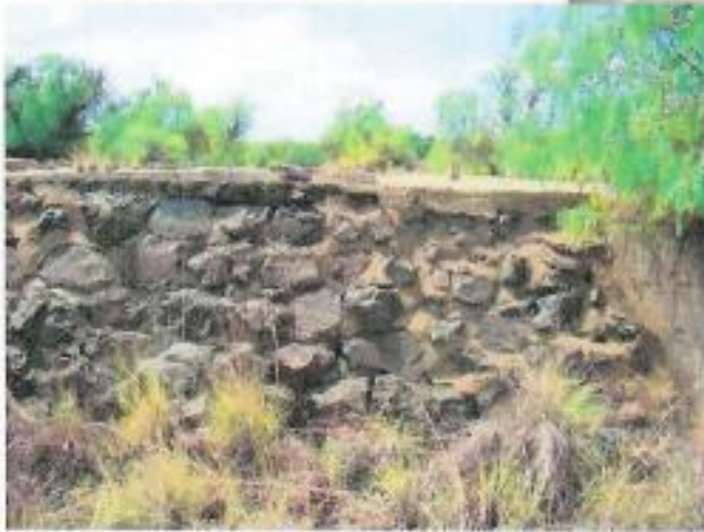
Figure 24 (group): Top and side views of dam on northern side of the Rock Shaft Plant – constructed of cement and rocks
