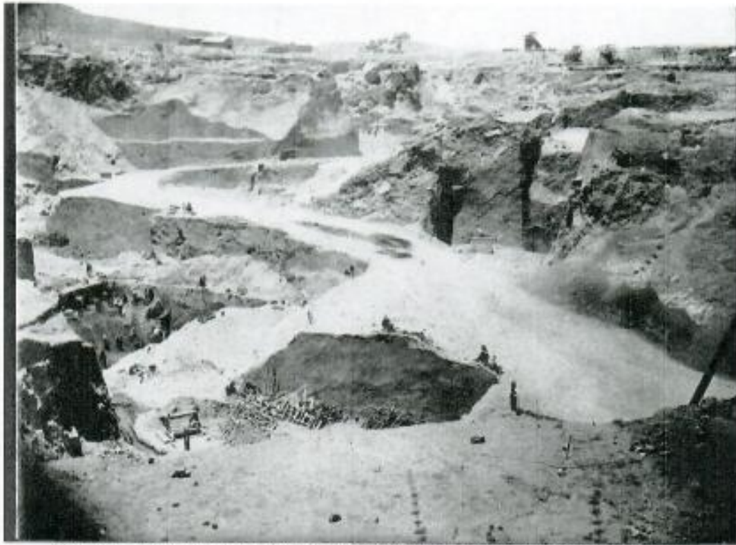
Figure 6: Photograph of the early years of the open mine pit area (DBMC archives)
