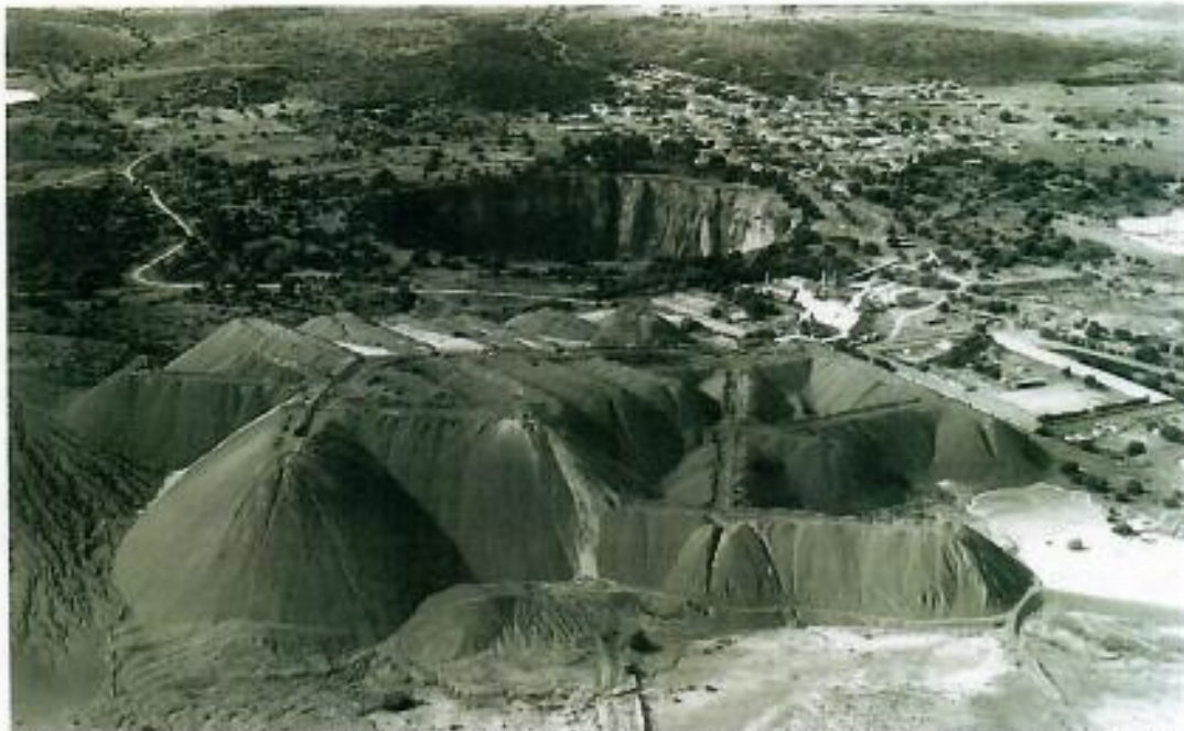
Figure 9: Aerial view of the mining area with the Modern Tailings Dump in the foreground, the new compound (the large rectangular set of buildings to the right) and the modern washing plant immediately north of that in line with the open pit mine. (DBMC archives)
