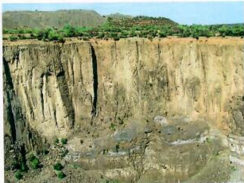
Figure 14: Southern side of open pit mine
