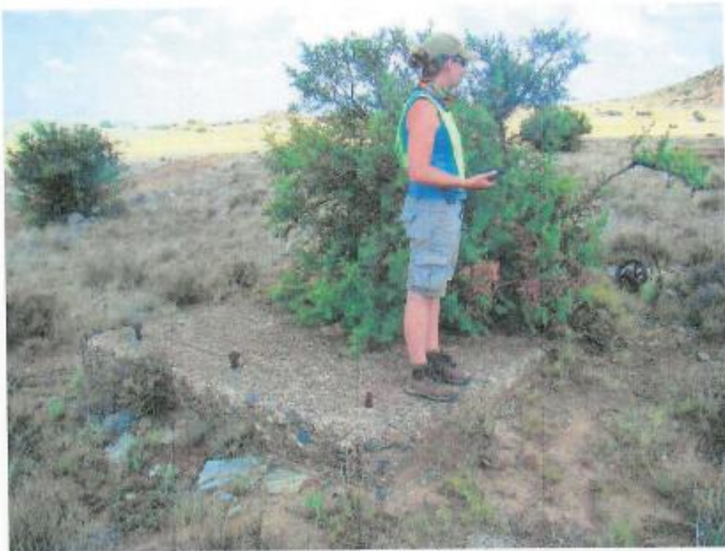
Figure 18: Concrete slabs in "floors" area
