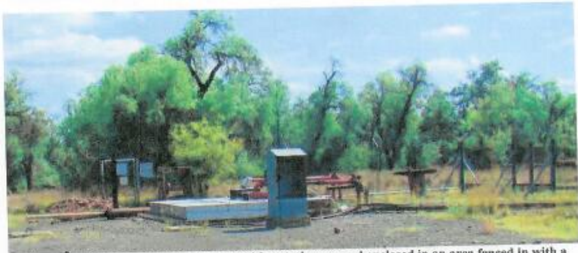
Figure 21: No 1 M.R. Shaft is covered with a steel cover and enclosed in an area fenced in with a high security fence and a padlocked gate. The headgear is now at the museum at the northern side of the open pit mine.
