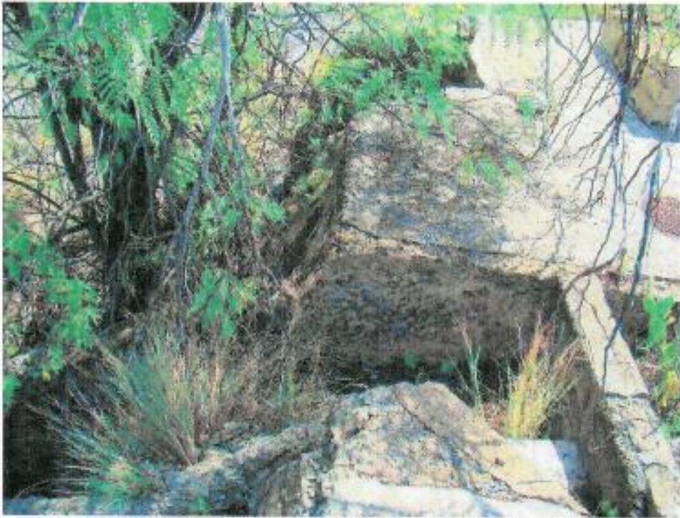
Figure 25: Unidentified concrete foundations at Rock Shaft area
