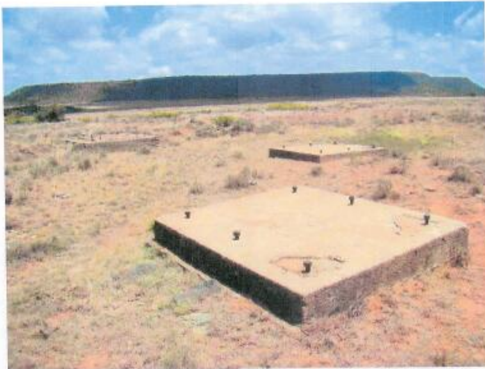
Figure 17: Concrete slabs - remains of haulage system at floors area (see map of South Section on page 33)
