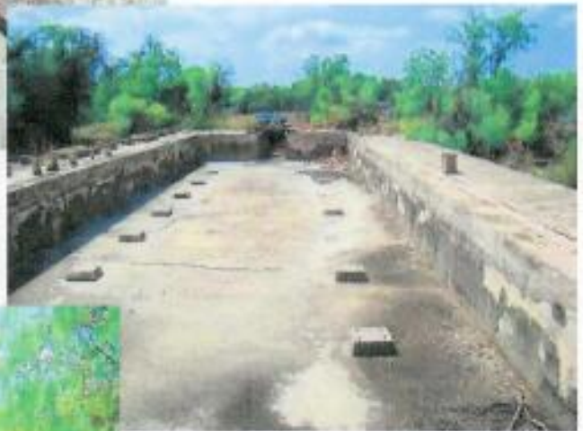
Figure 24 (group): Top and side views of dam on northern side of the Rock Shaft Plant – constructed of cement and rocks
