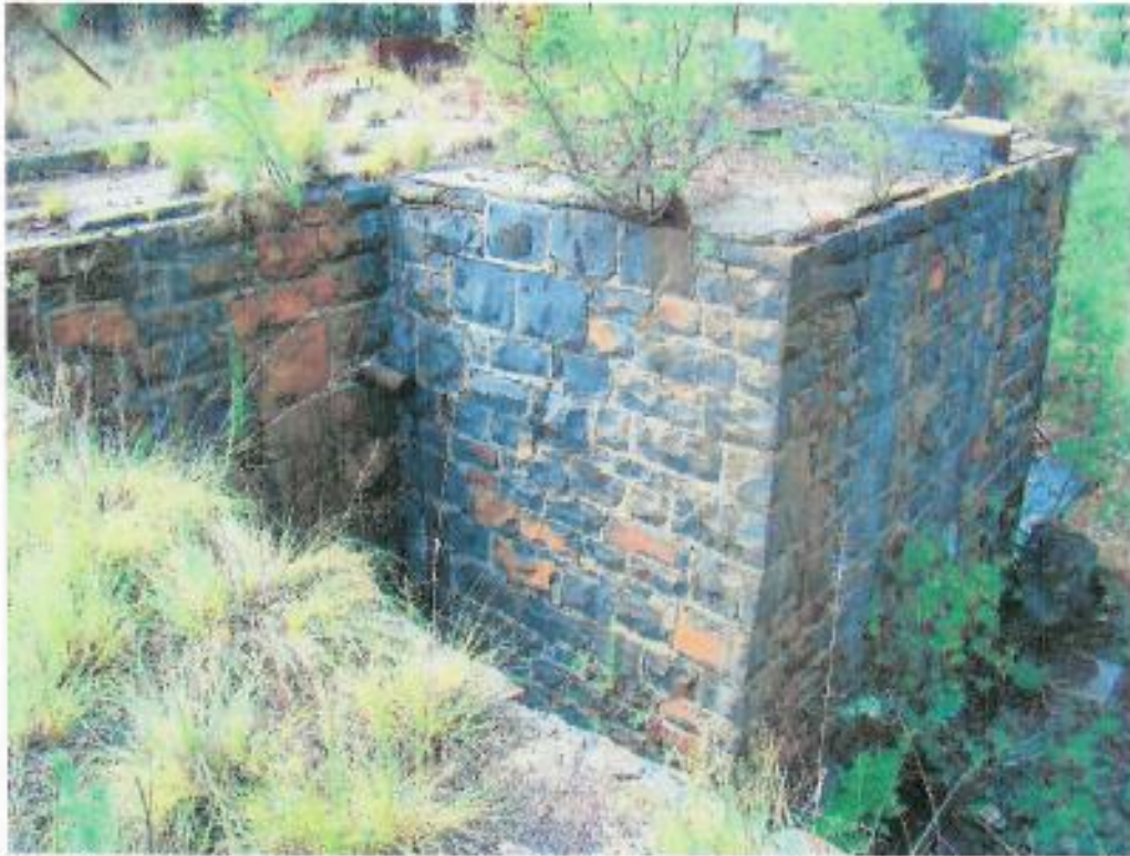
Figure 27: On the south-eastern side of the dam in the previous pictures are the remains of the following structures – remains of shaft office in far background
