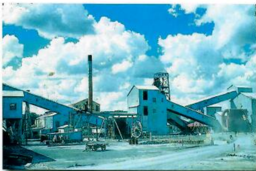
Jagersfontein Mine : No. 1 Rock Hoist and a section of the Treatment Plant on day of closing 28 th May 1971
