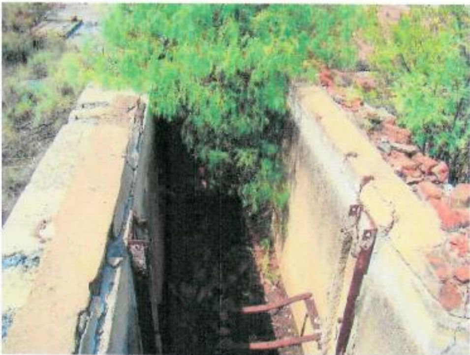
Figure 26: Concrete canal at Rock Shaft area
