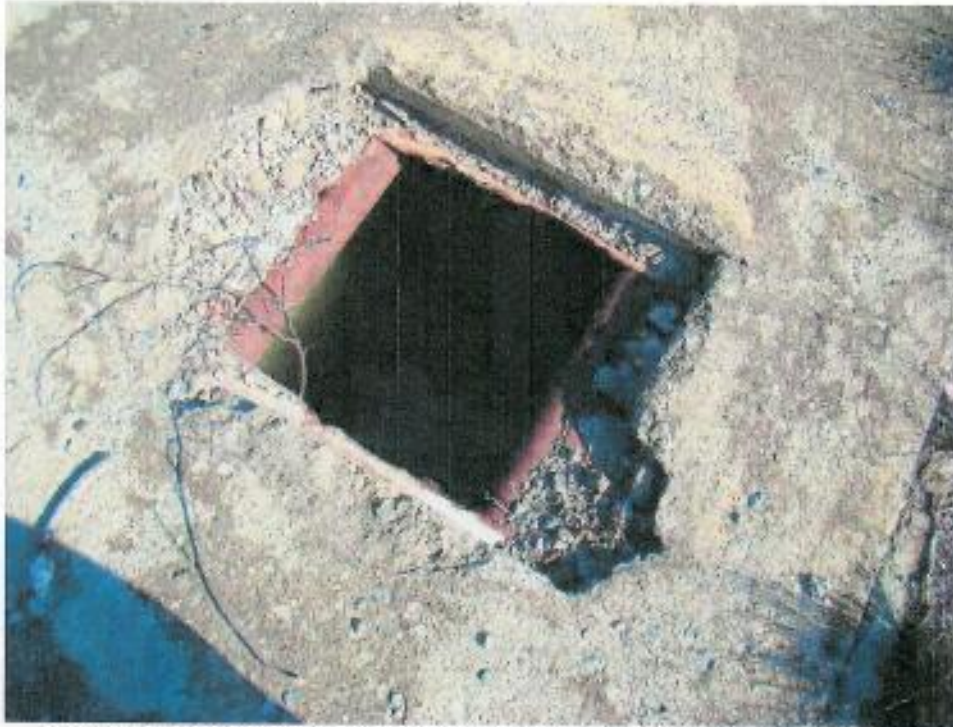
Figure 73: Detail of metal fixtures to concrete surface at Washing Plant area (2)
