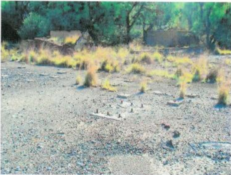
Figure 74: Detail of metal fixtures to surface of Washing Plant area (3)
