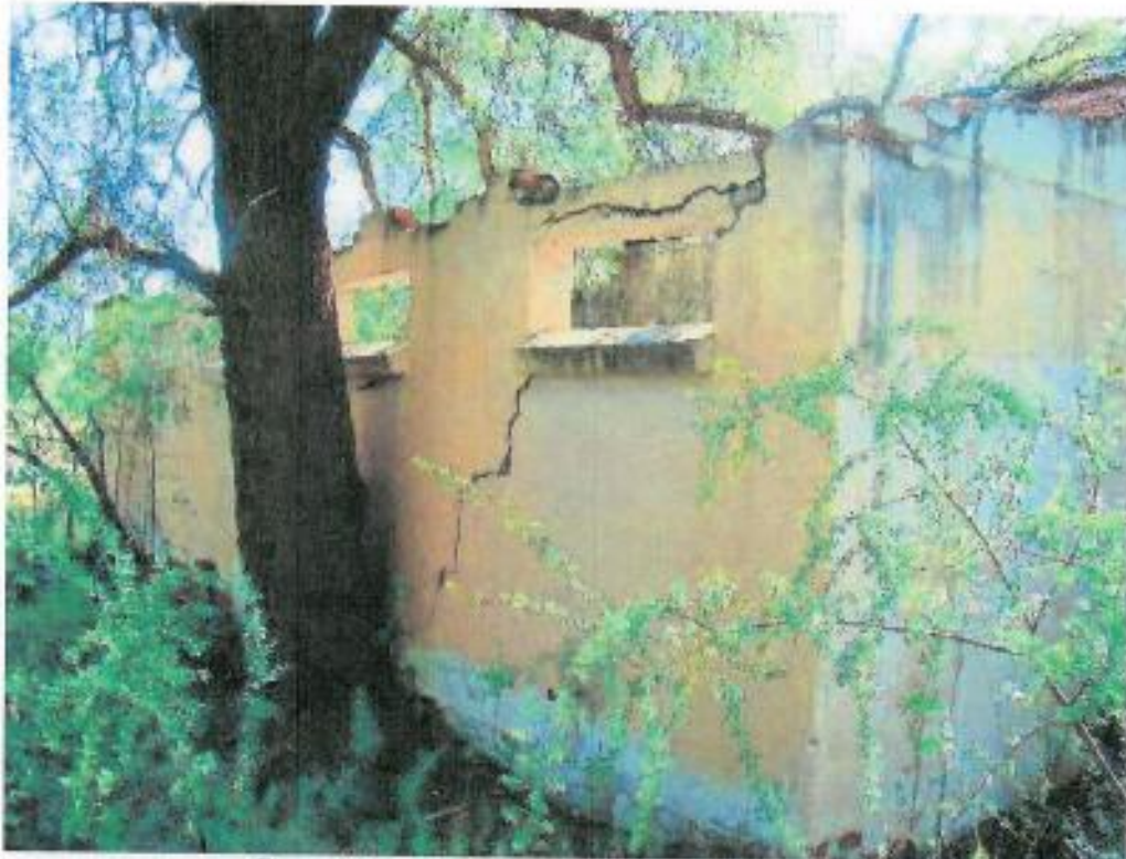
Figure 44: Eastern side of exterior of Shaft Offices
