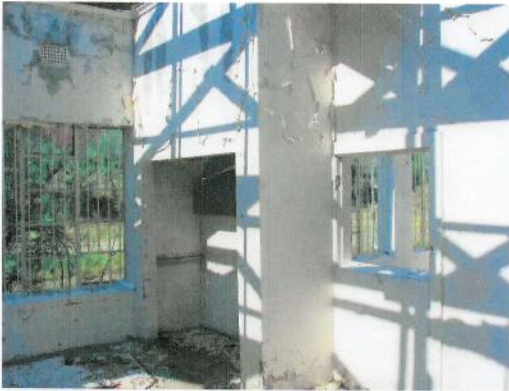
Figure 87: Interior of offices at Washing Plant area (1)
