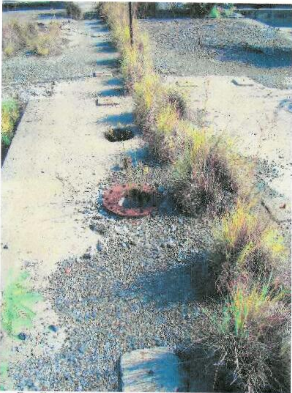
Figure 72: Detail of metal fixtures to concrete surfaces at Washing Plant area (1)
