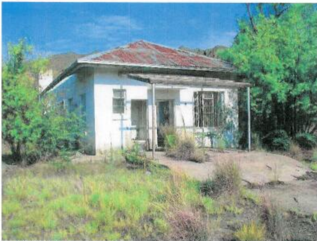
Figure 86: Eastern entrance of offices at Washing Plant area (western orientation)
