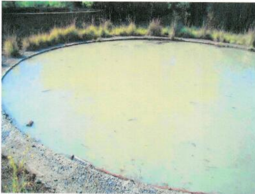
Figure 81: Detail of sunken dam in picture 36 above. Depth unknown.
