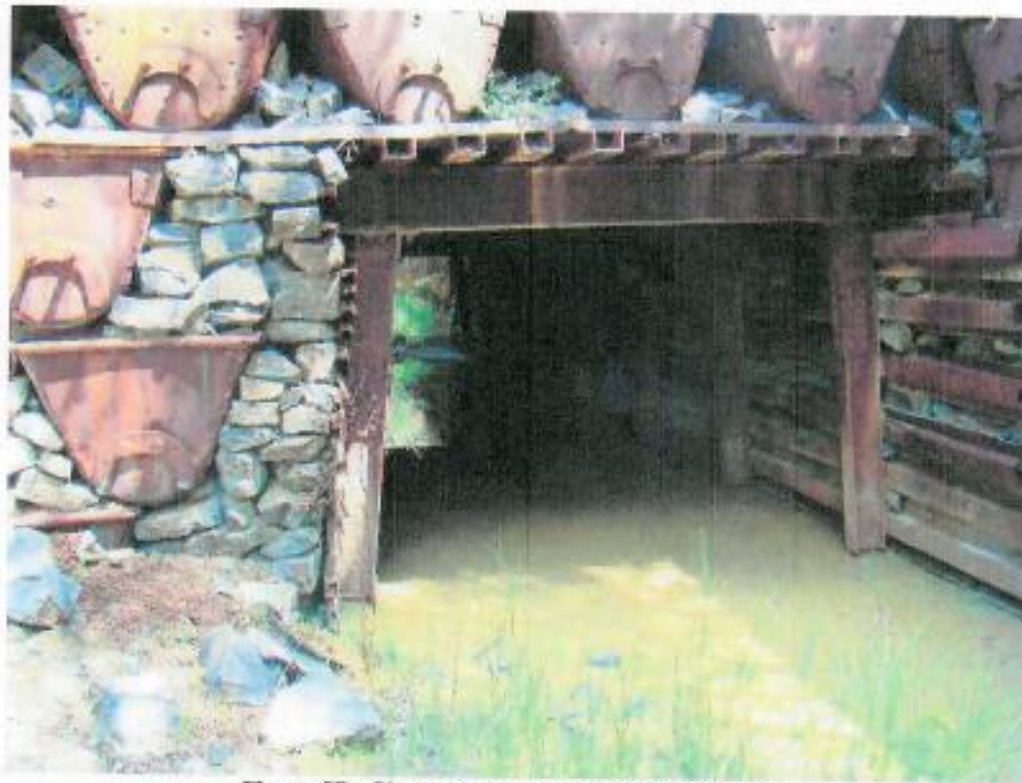
Figure 57: Close-up view of canal passage in wall
