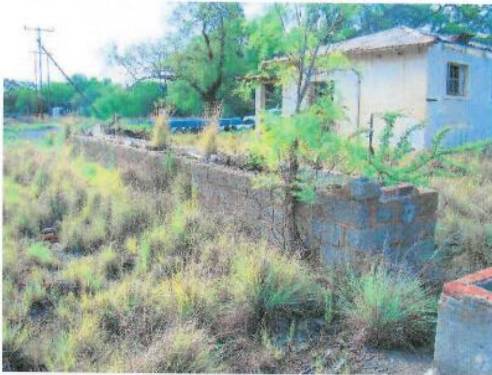
Figure 48: Structures on northern side of Shaft Offices
