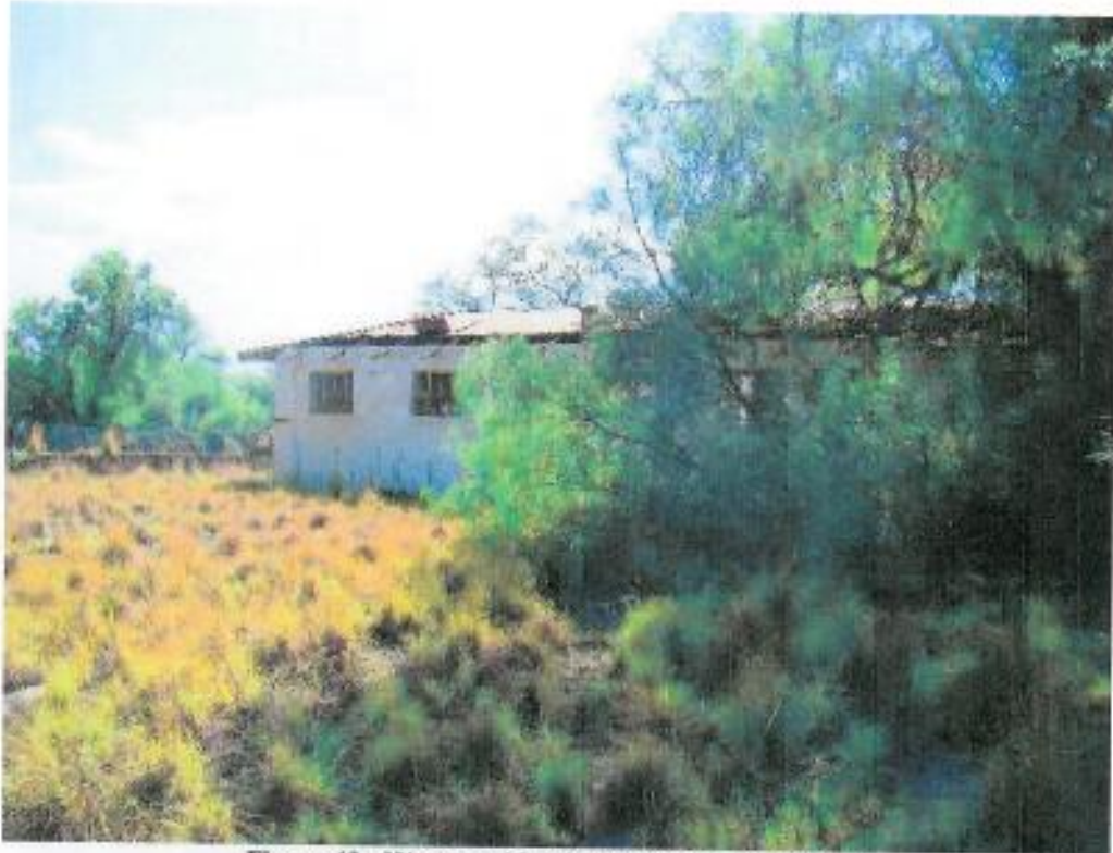
Figure 43: Western side of exterior of Shaft Offices
