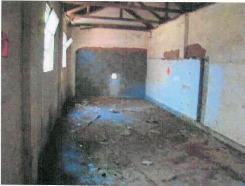
Figure 41: Interior of Change House adjacent Shaft Offices (eastern section)
