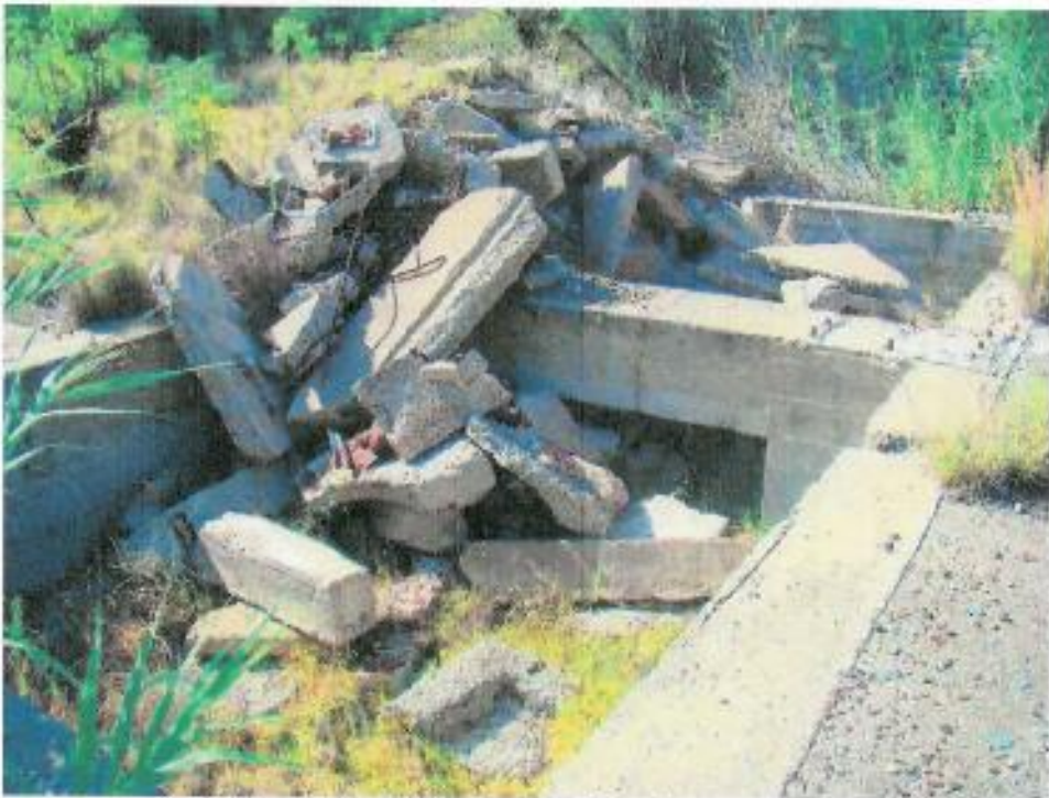
Figure 79: Debris from Washing Plant area (2)
