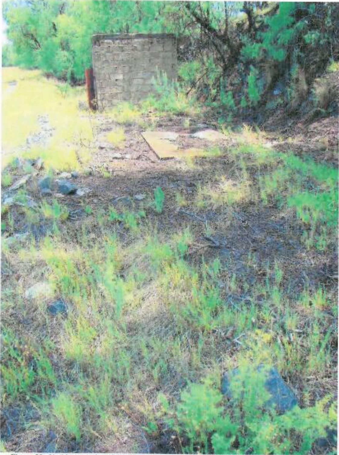
Figure 55: Nothing remains of the Timber area that is on the southern side of the retainer wall discussed below. The cement slab and cement structure seem to be later additions
