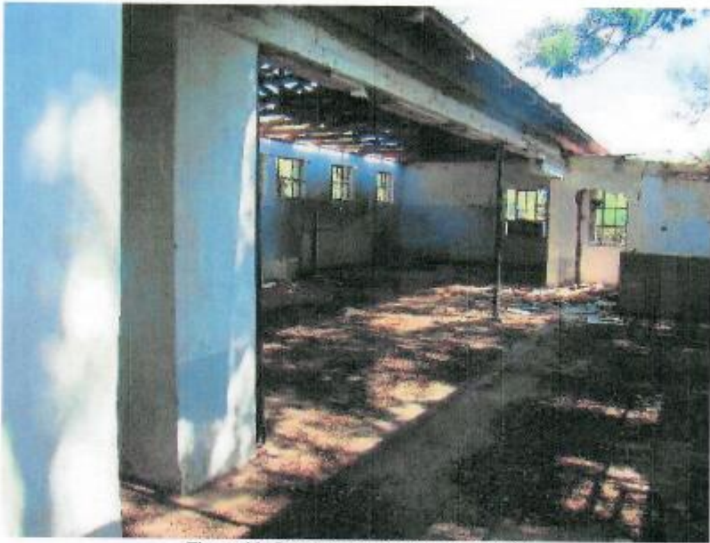
Figure 46: Interior view of Shaft Offices (2)
