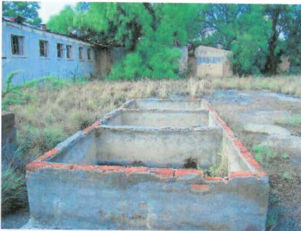
Figure 47: Structures on western side of Shaft Offices
