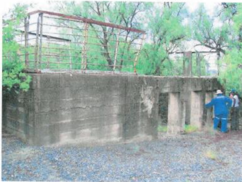
Figure 92: As above (orientation north-west)
