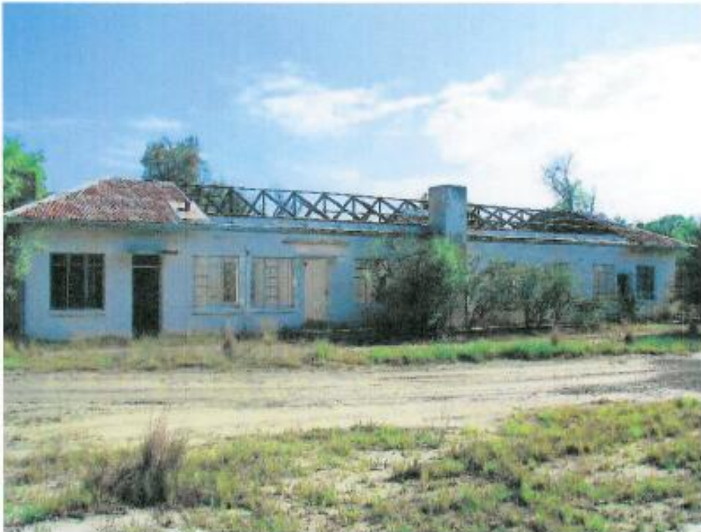
Figure 85: Offices in Washing Plant area (north-easterly orientation)
