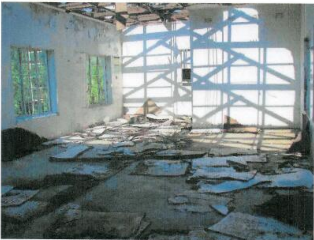
Figure 88: Interior of offices at Washing Plant area (2)
