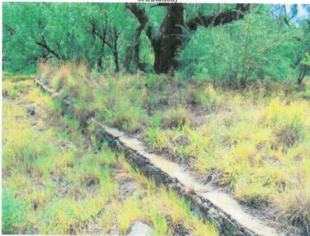
Figure 54: Foundation of unknown structure - orientation north-east
