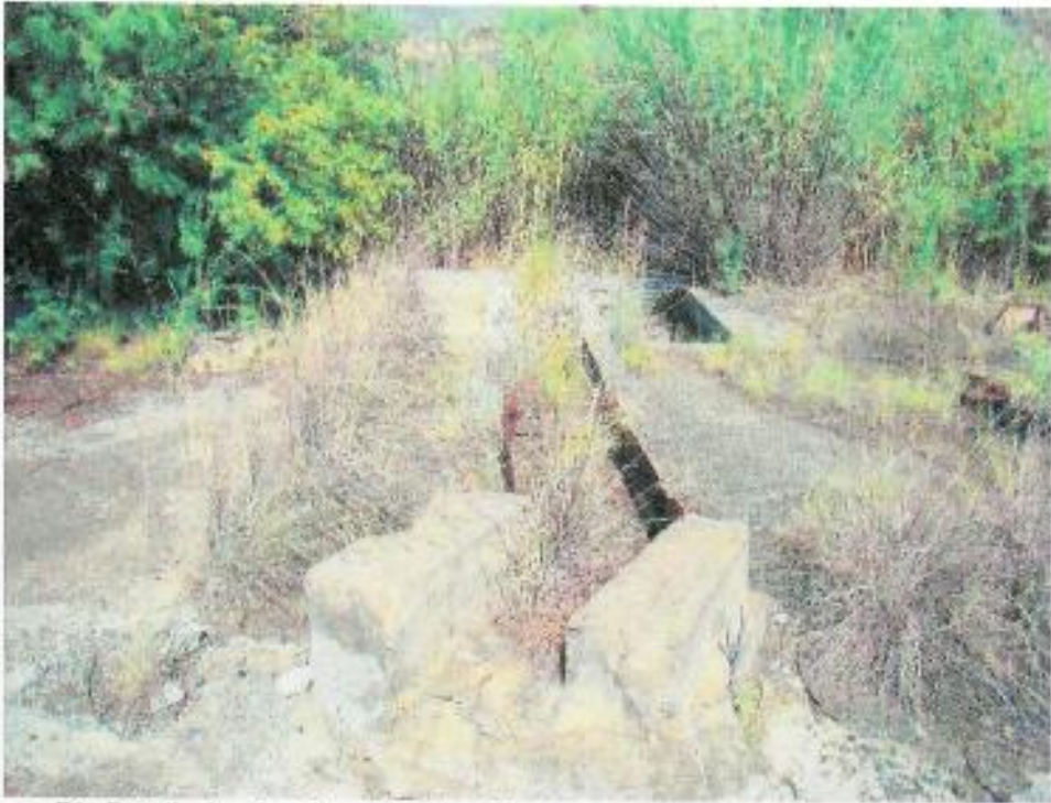
Figure 76: Detail of outlets from Washing Plant area to Settlement dams on western side (2)
