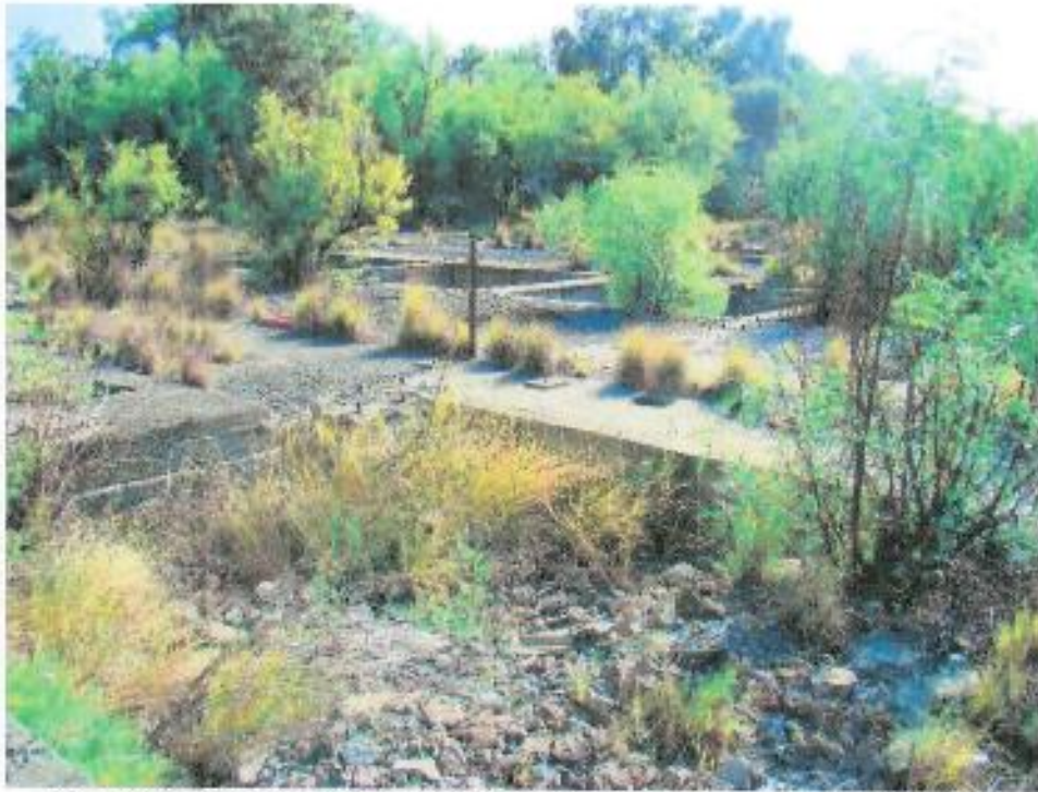
Figure 63: Overall view of Washing Plant surface – north-easterly orientation
