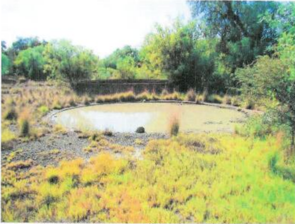
Figure 80: Dams in area between Settling Dams and Washing Plant
