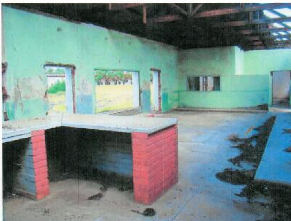
Figure 128: Interior of shop area
