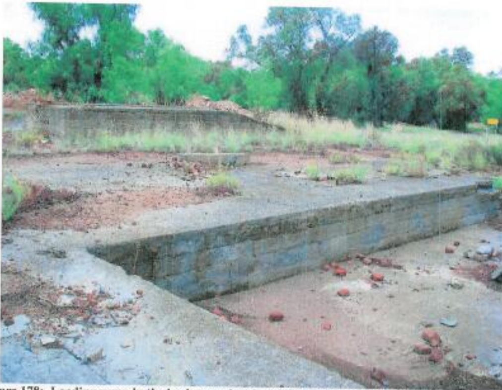
Figure 178: Loading ramp in the background and a sunken rectangular construction with an open end in the foreground
