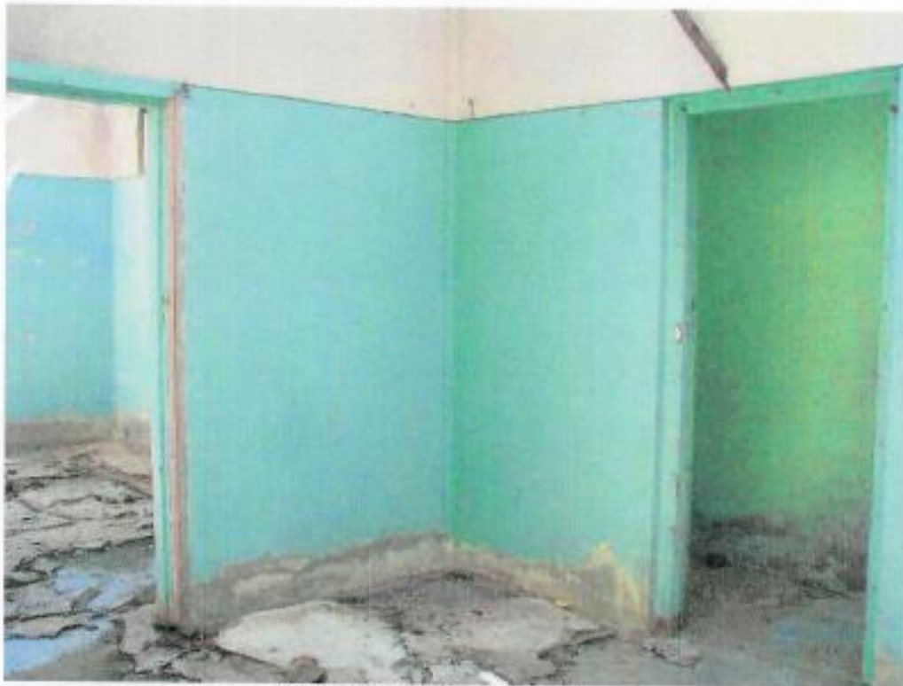
Figure 141: Interior of hospital area
