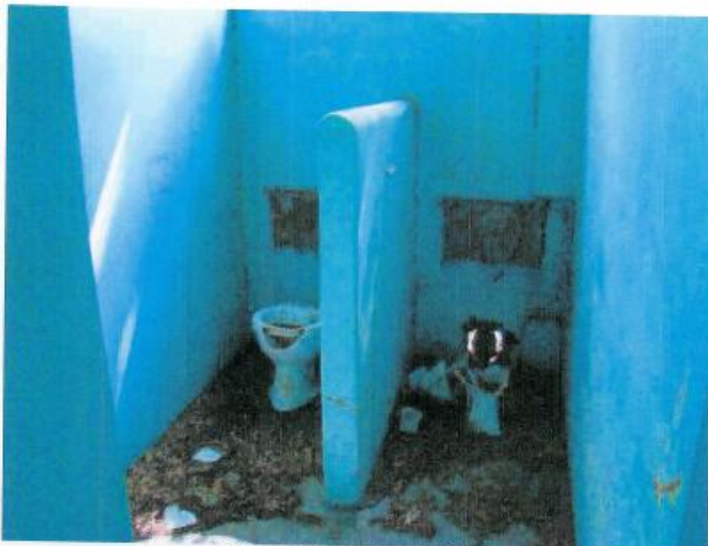
Figure 114: Senior Quarters Toilets
