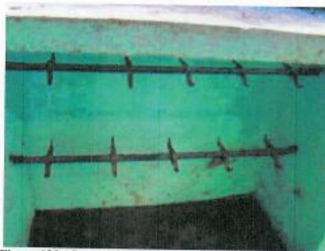
Figure 123: Space in storage area for cooking pots to hang
