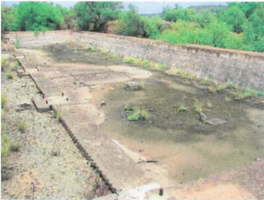
Figure 152: To the west of this lies a succession of cement channels that leads from this reservoir (view photographs below) Judged by the bolts and nuts in both the middle and sides of the dam as well as the patterned edge this structure probably served as foundation for machinery or tanks that were housed in a corrugated iron structure.
