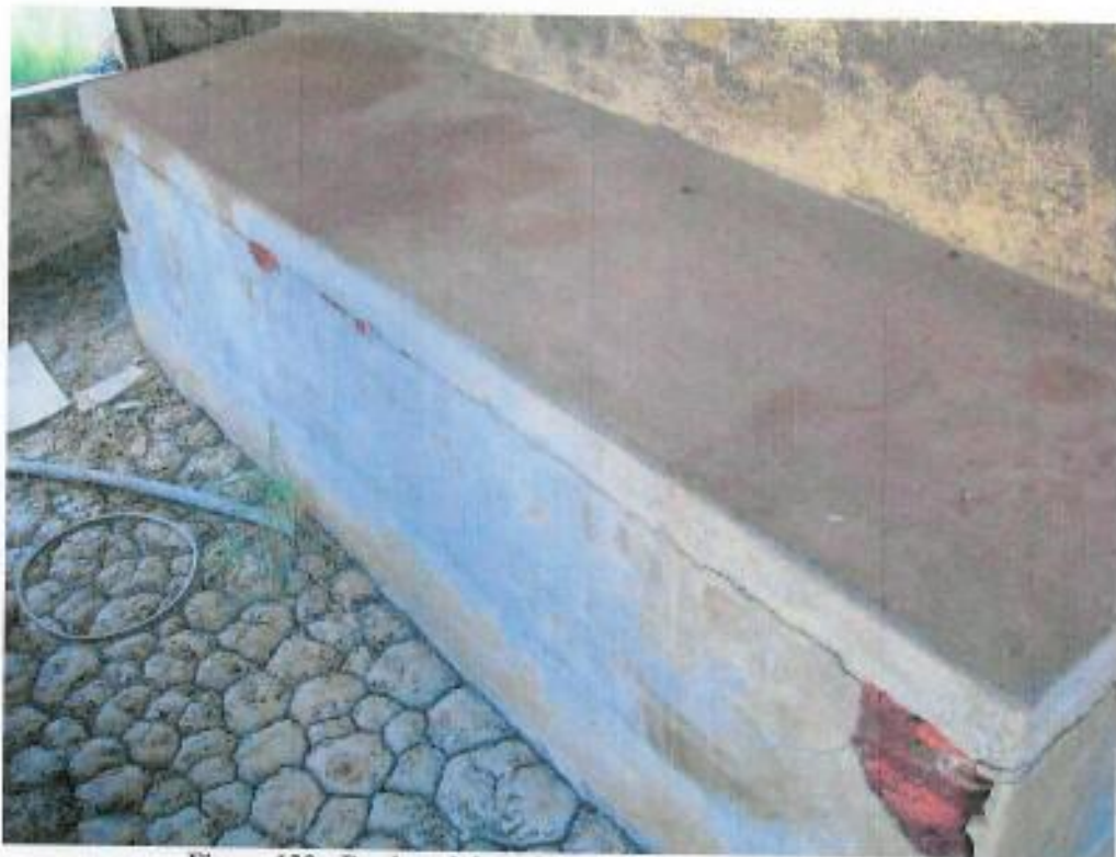
Figure 139: Bunker slab to the right of the examination table
