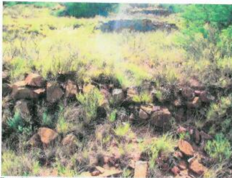
Figure 166: From this angle the different sections of this building are clearly visible with the middle row of stones the divider wall between the two areas.
