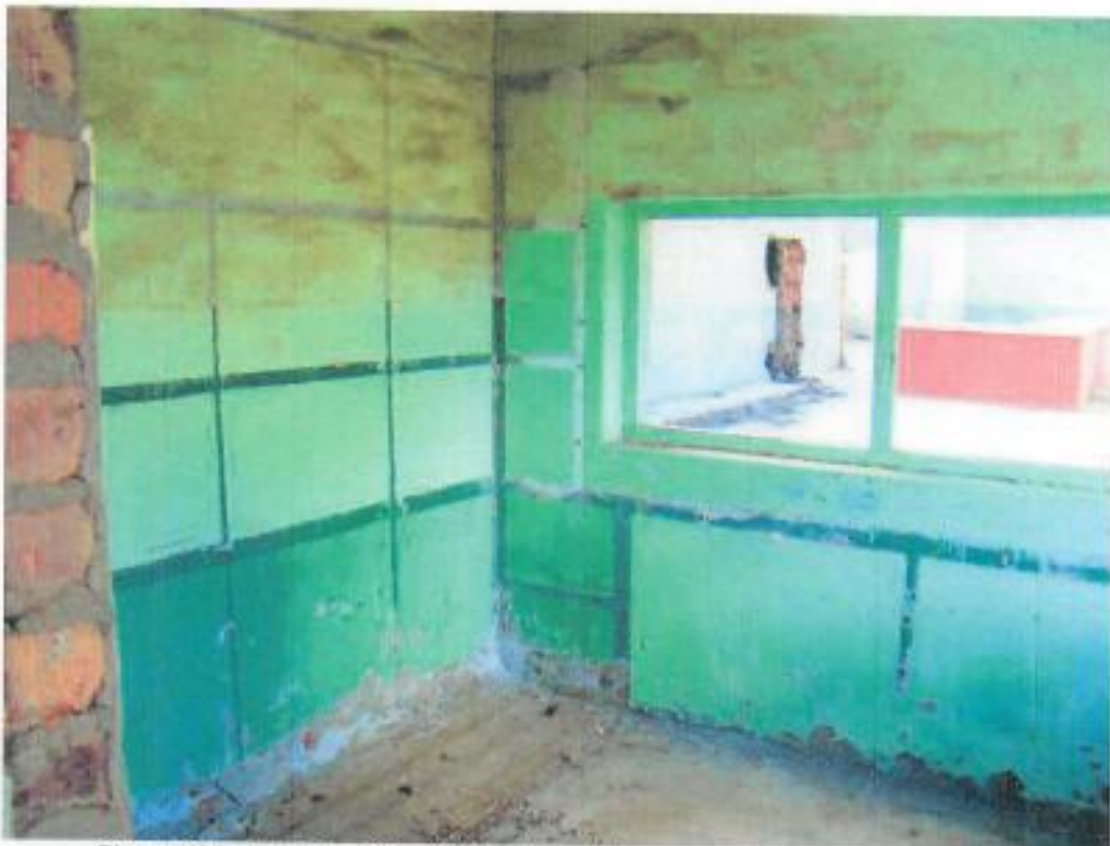
Figure 127: Interior of Post Office Area (Shop area visible through window)
