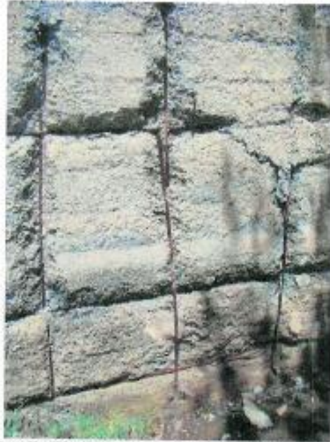
Figure 146: Detail of building material (steel reinforced concrete slabs)
