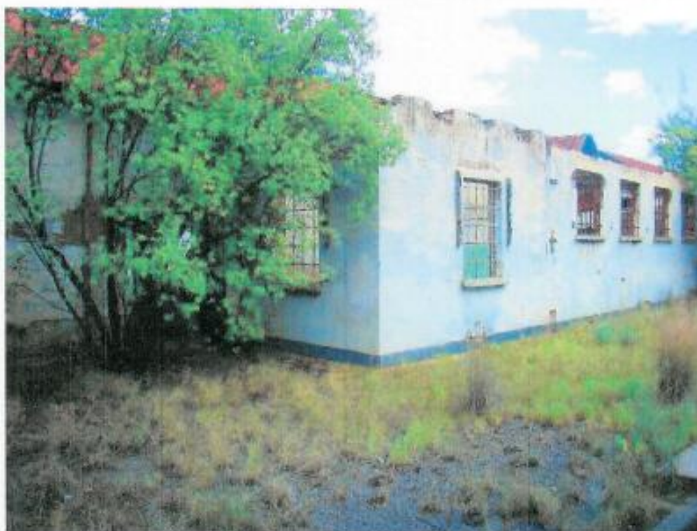
Figure 125: Close up of eastern wall of office area
