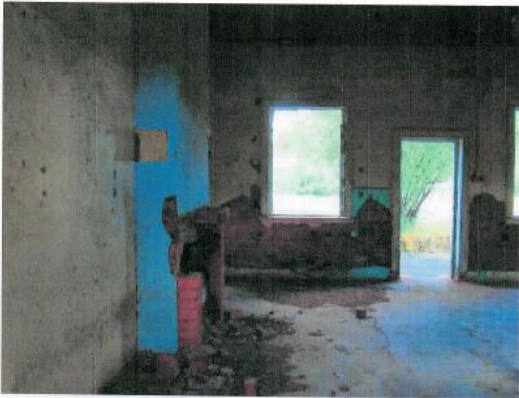
Figure 126: Interior of office area
