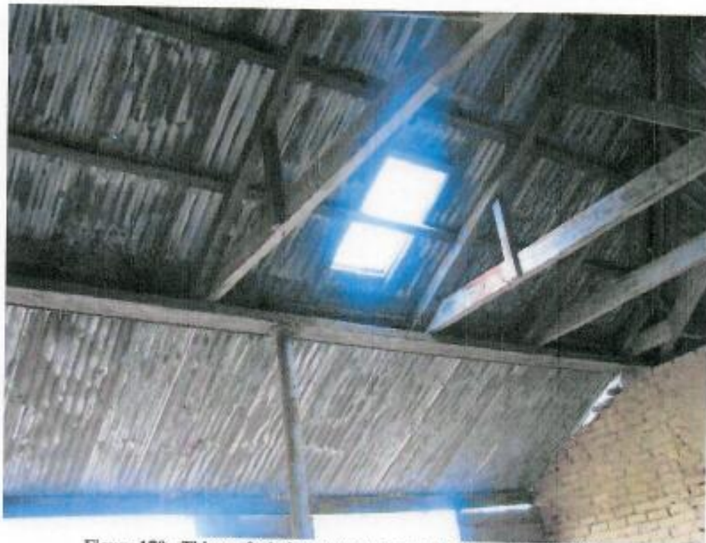
Figure 170: This roof window seems to be part of the original building
