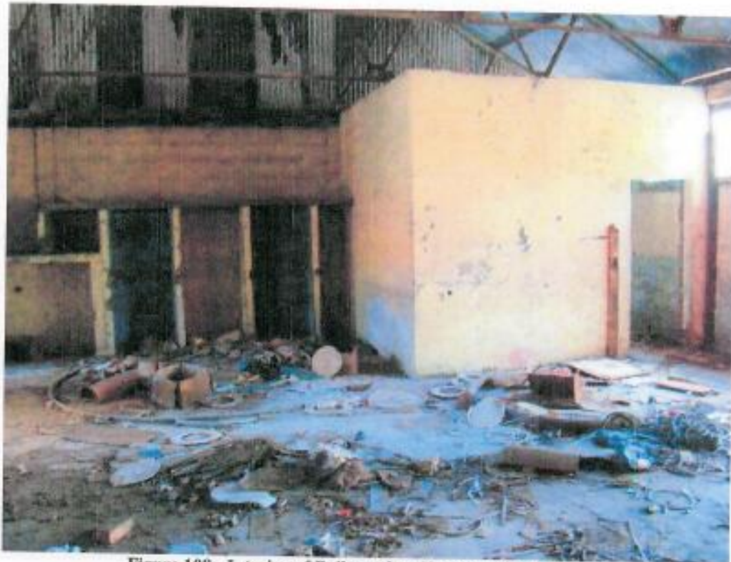
Figure 108: Interior of Boilermaker Shop – orientation west
