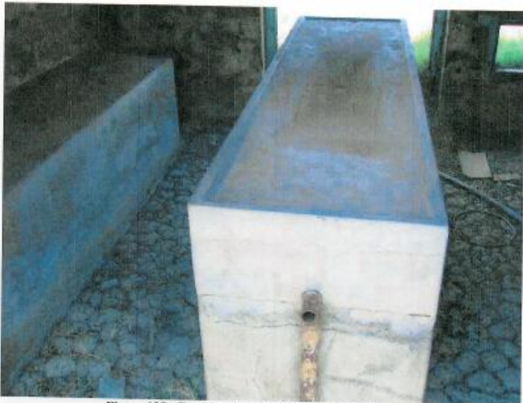
Figure 138: Examination slab with bunker slab on left
