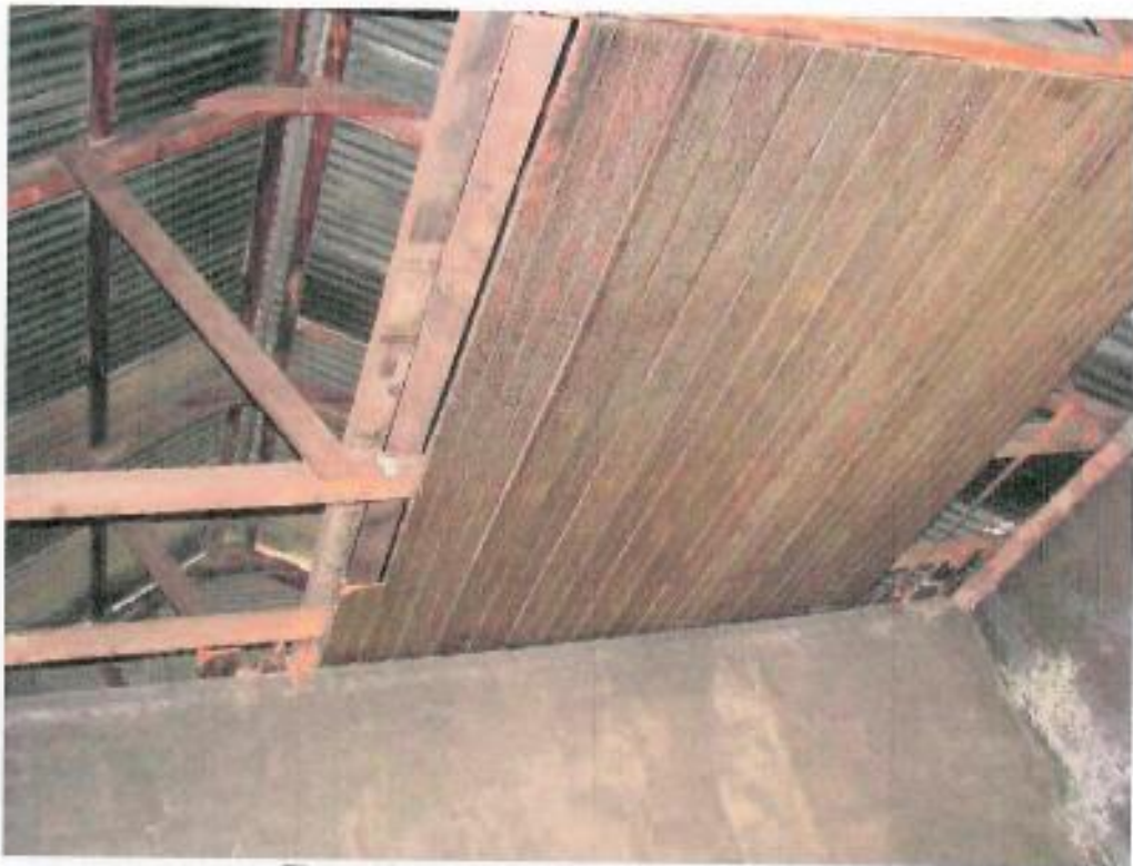
Figure 135: Wooden ceiling of Isolation Ward
