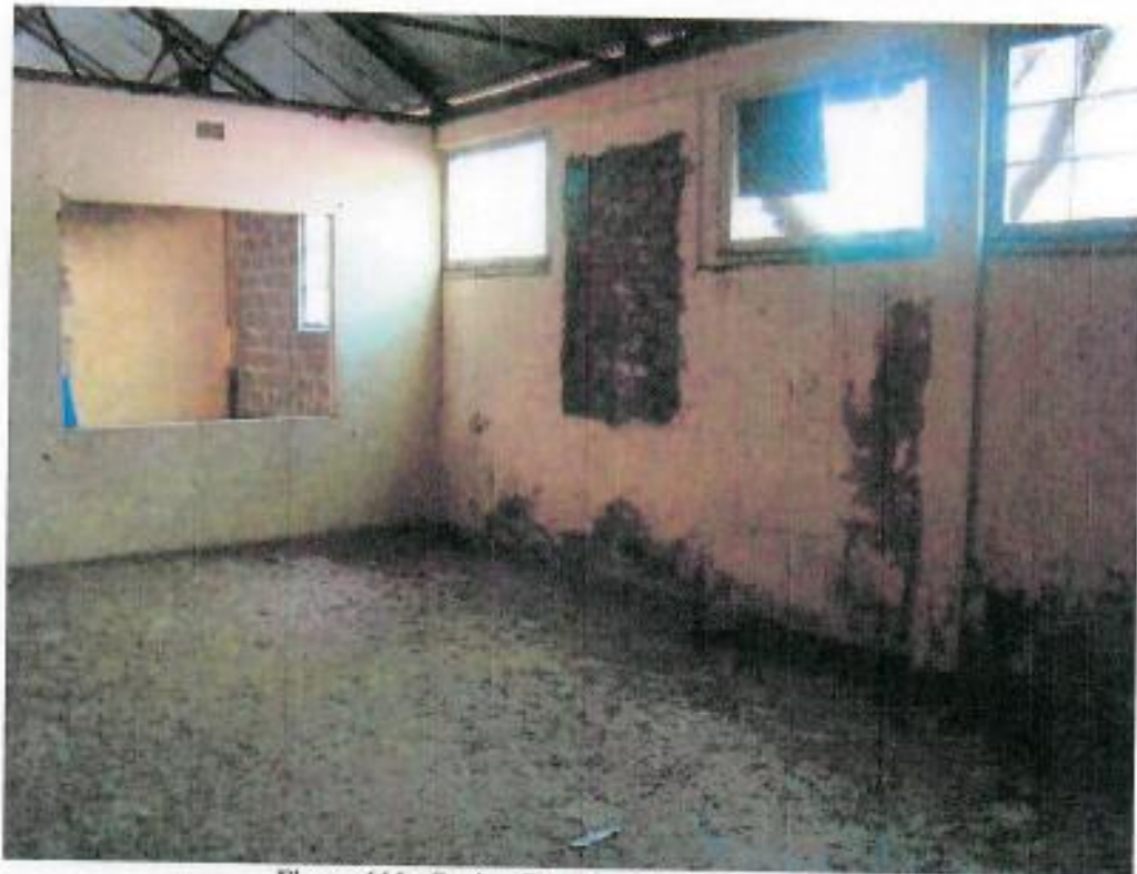
Figure 111: Senior Quarters Recreational Area
