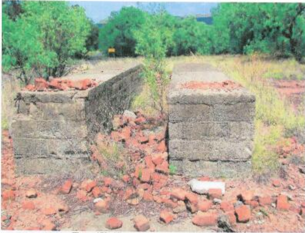
Figure 179: View of loading ramp from the back
