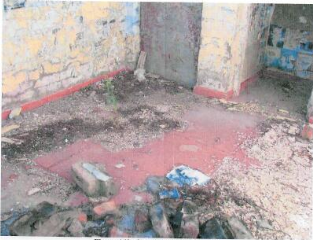
Figure 142: Interior of hospital area
