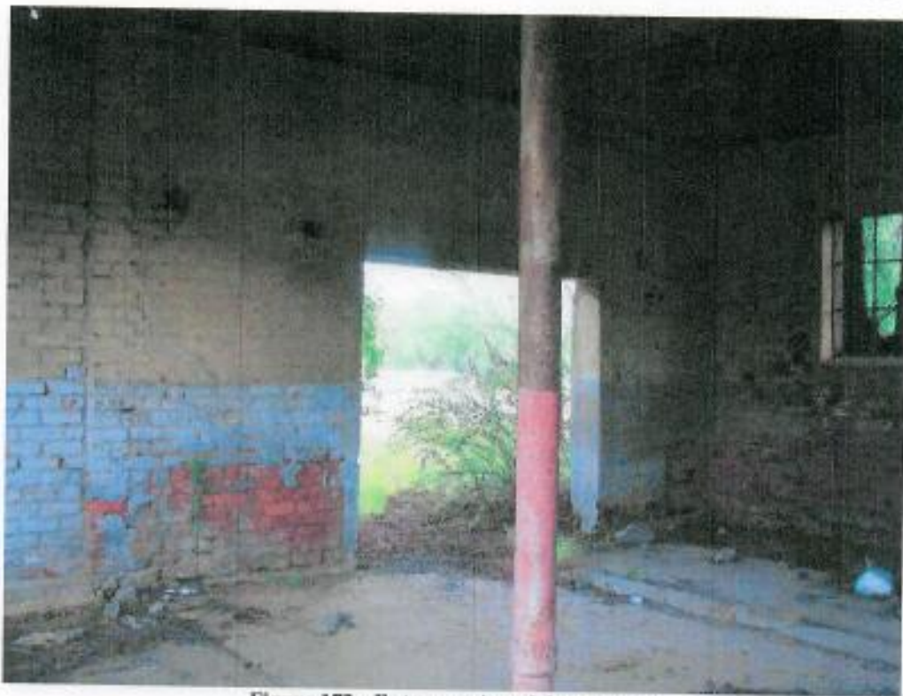
Figure 172: Entrance viewed from inside
