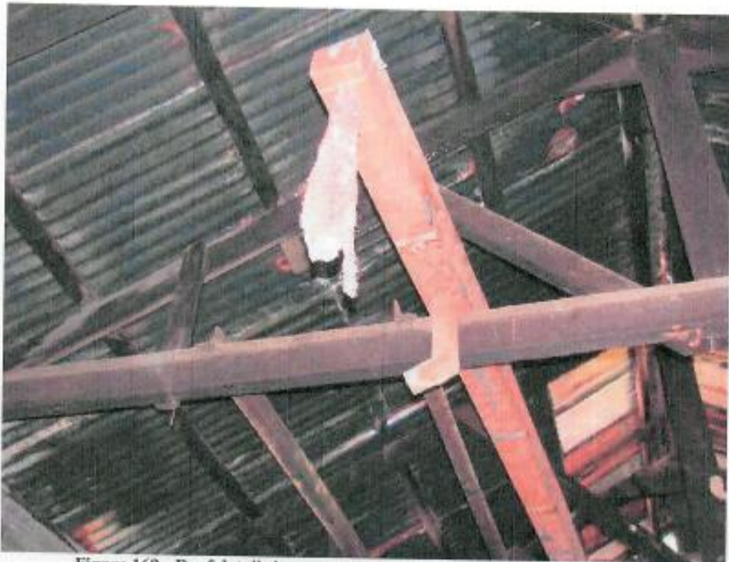
Figure 169: Roof detail shows a gutter resting on the roof support beams
