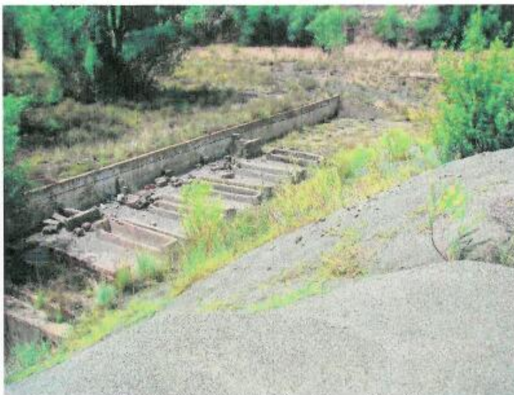
Figure 204: Remaining foundations of power station (1)
