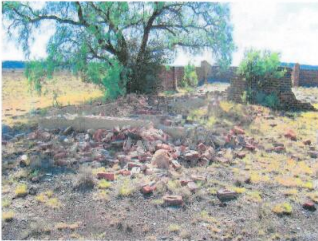
Figure 229: Demolished section (orientation south-west)
