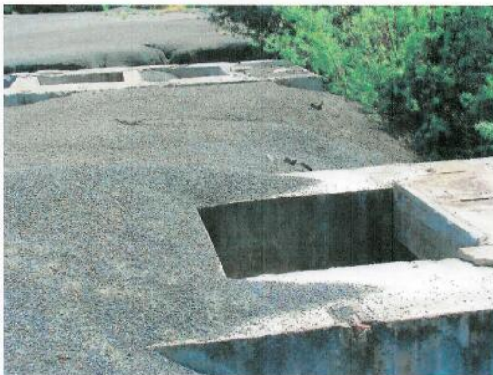
Figure 205: Remaining foundation of Power Station (2)
