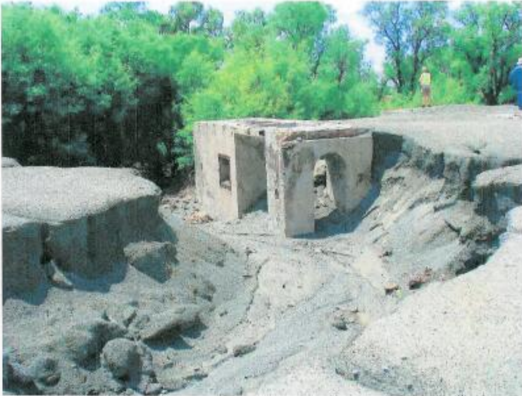
Figure 206: Remaining foundation of Power Station (3)
