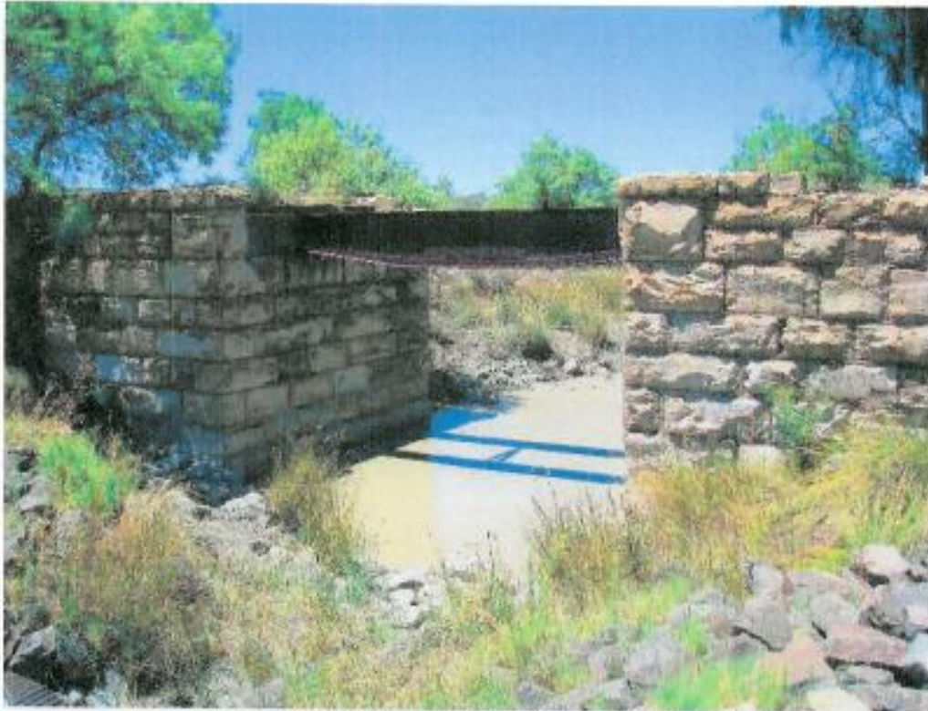
Figure 220: Remains of sideline railway bridge (1)
