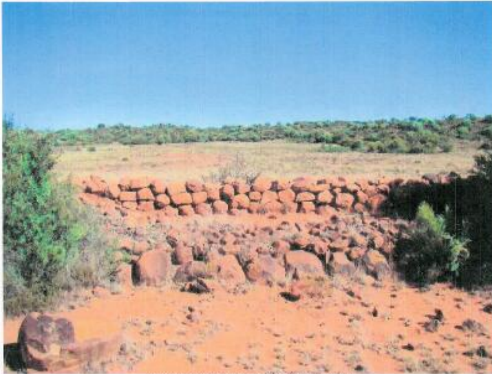
Figure 183: Retainer wall at dam area
