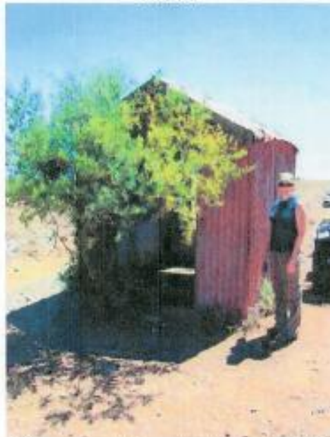
Figure 233: Close-up view of the corrugated iron structure - the interior suggests this to have been used as bathroom (toilets)
