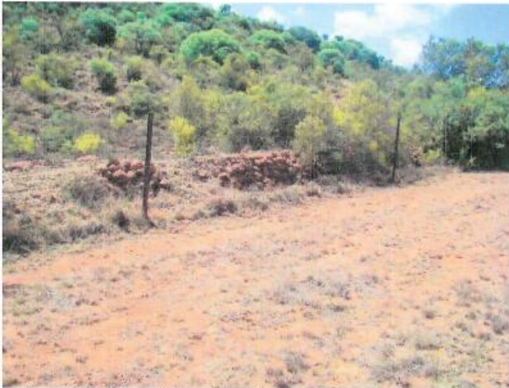
Figure 187: Retainer wall in southern section of surveyed area - see map on page 33
