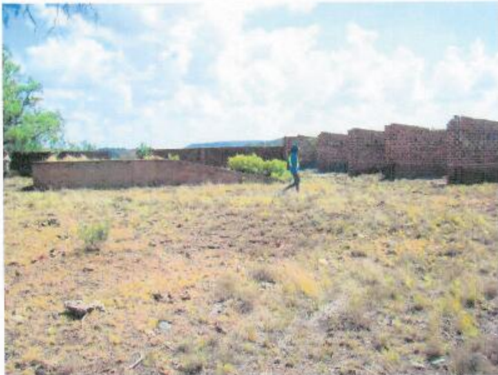
Figure 231: Loading ramp with cubicles on right hand side (orientation south)
