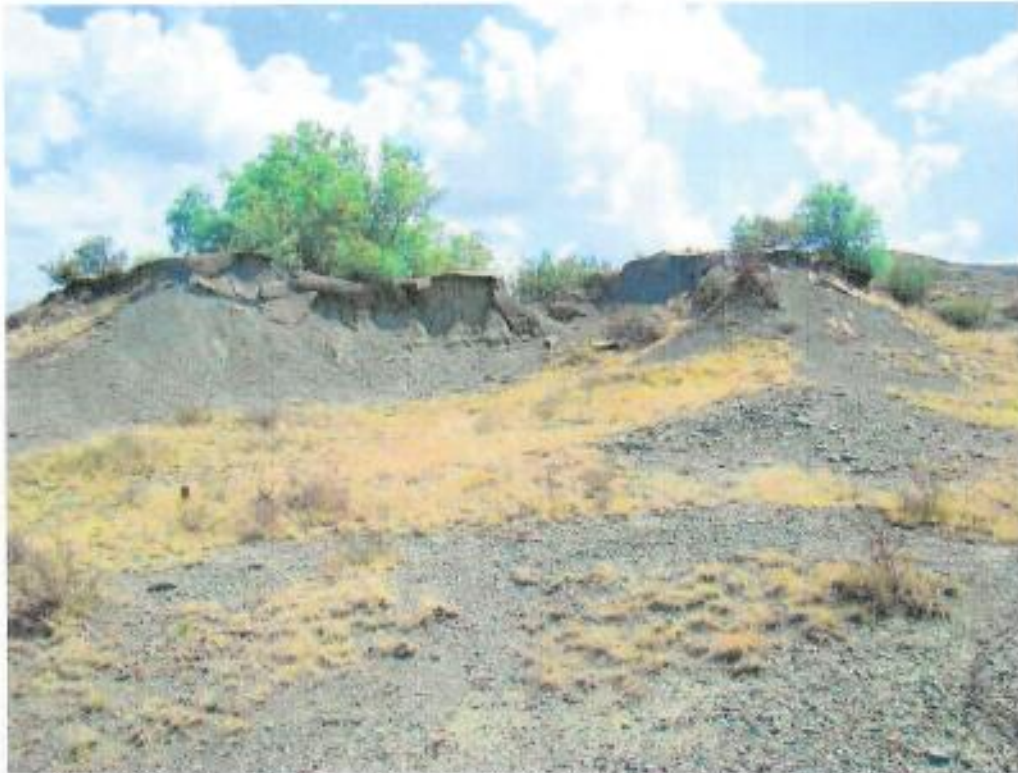
Figure 223: side view of the hollowed out structure (partially dismantled or collapsed)
