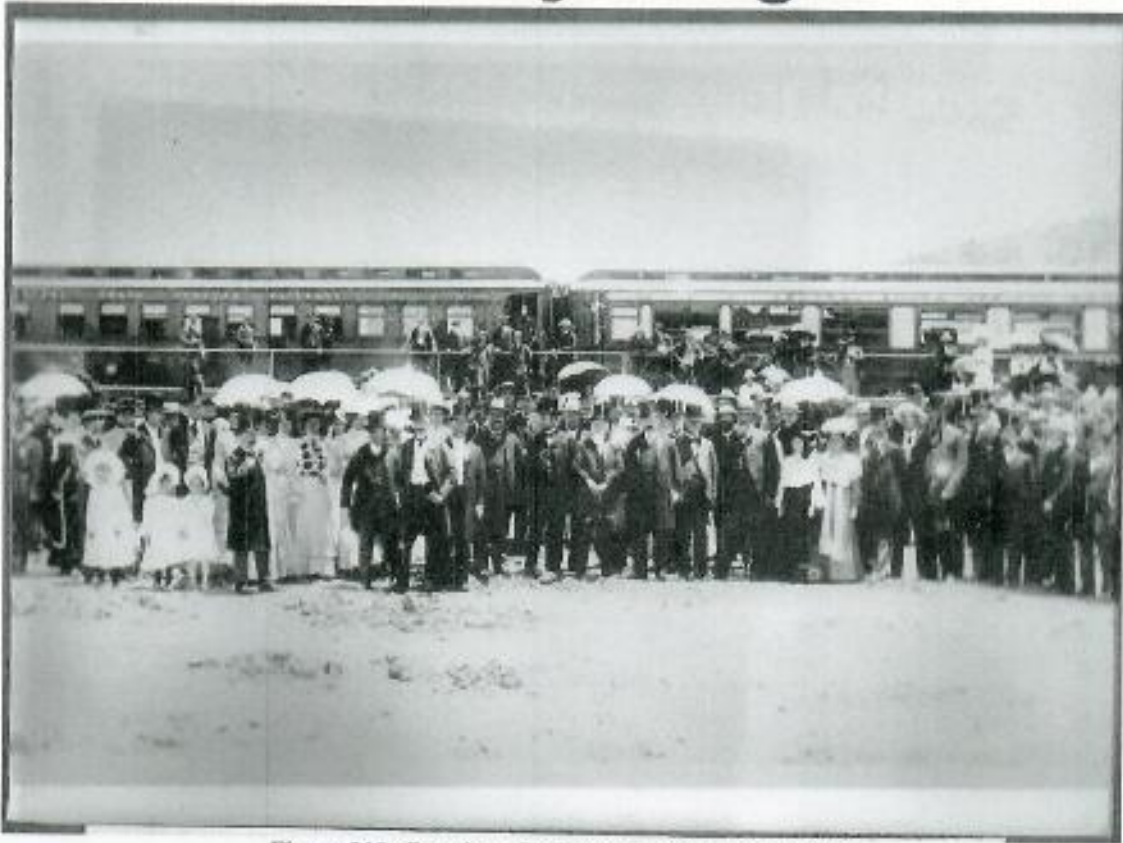
Figure 219: Opening of railway line 31 January 1905
