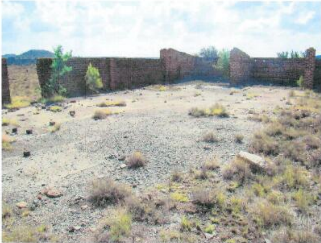
Figure 228: Cubicles or rooms for coal storage (orientation west)
