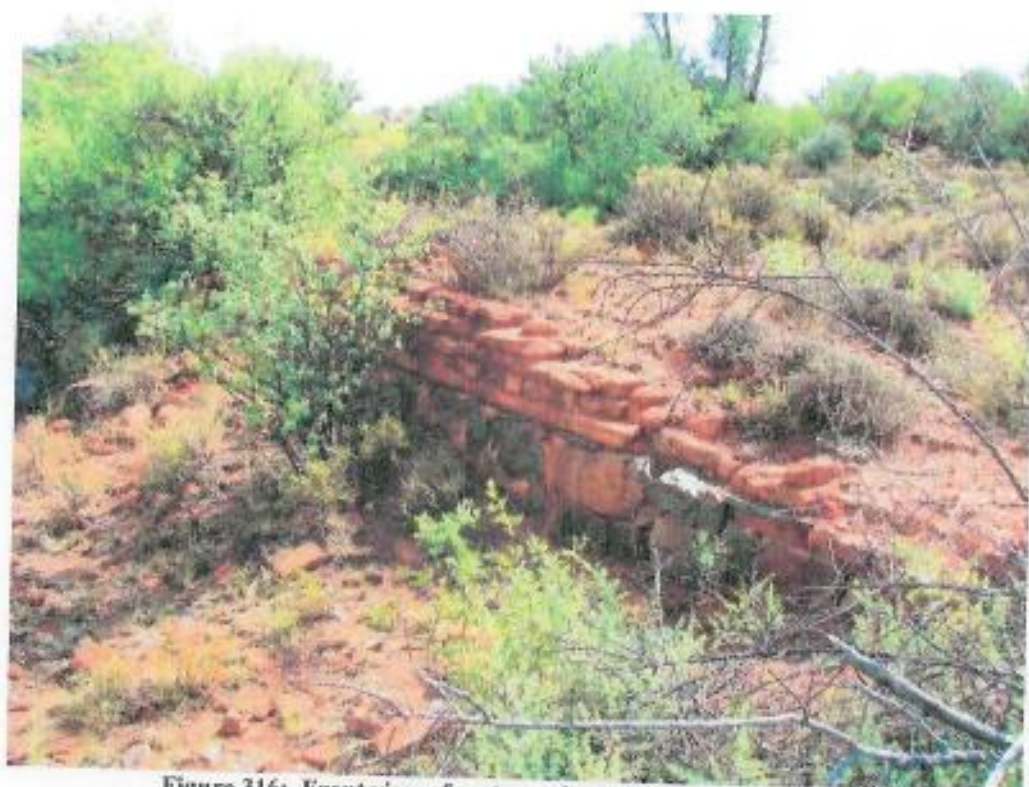
Figure 316: Front view of eastern wing (orientation south-west)
