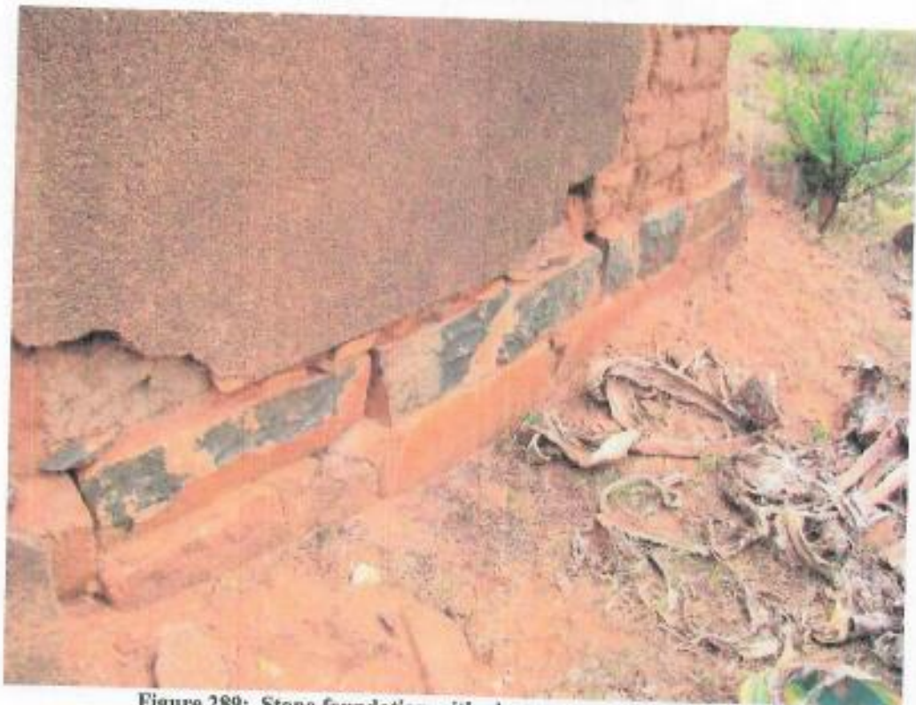
Figure 289: Stone foundation with plaster over mudstone bricks
