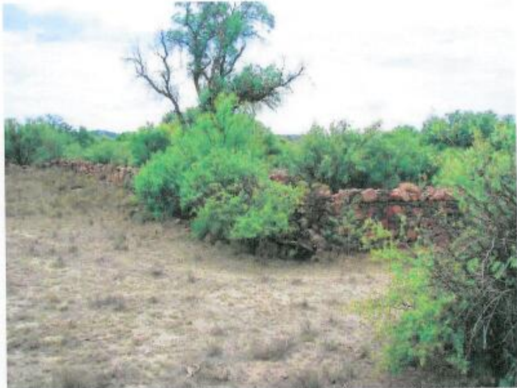
Figure 262: Large opening (on right hand side in photograph) in eastern wall viewed from inside the enclosed courtyard area
