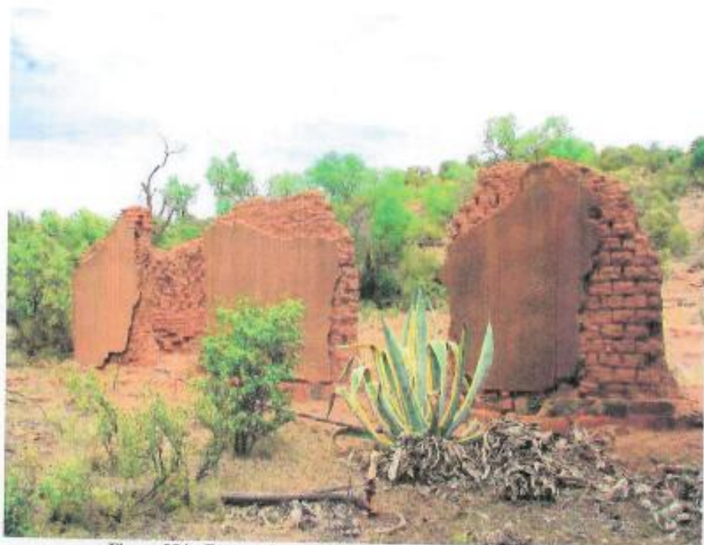
Figure 284: Eastern face of the remains (orientation south-west)
