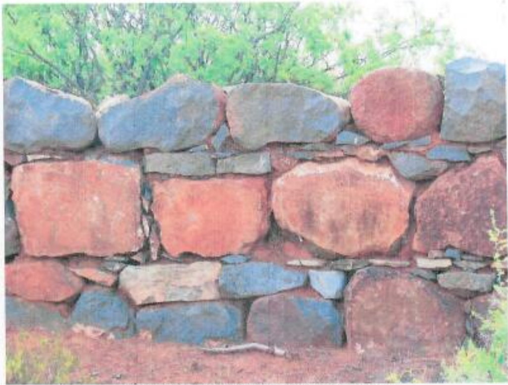
Figure 256: Detail of constructed stone wall (1)
