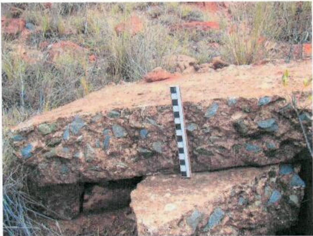
Figure 265: Portion of cement slab on outside of western wall
