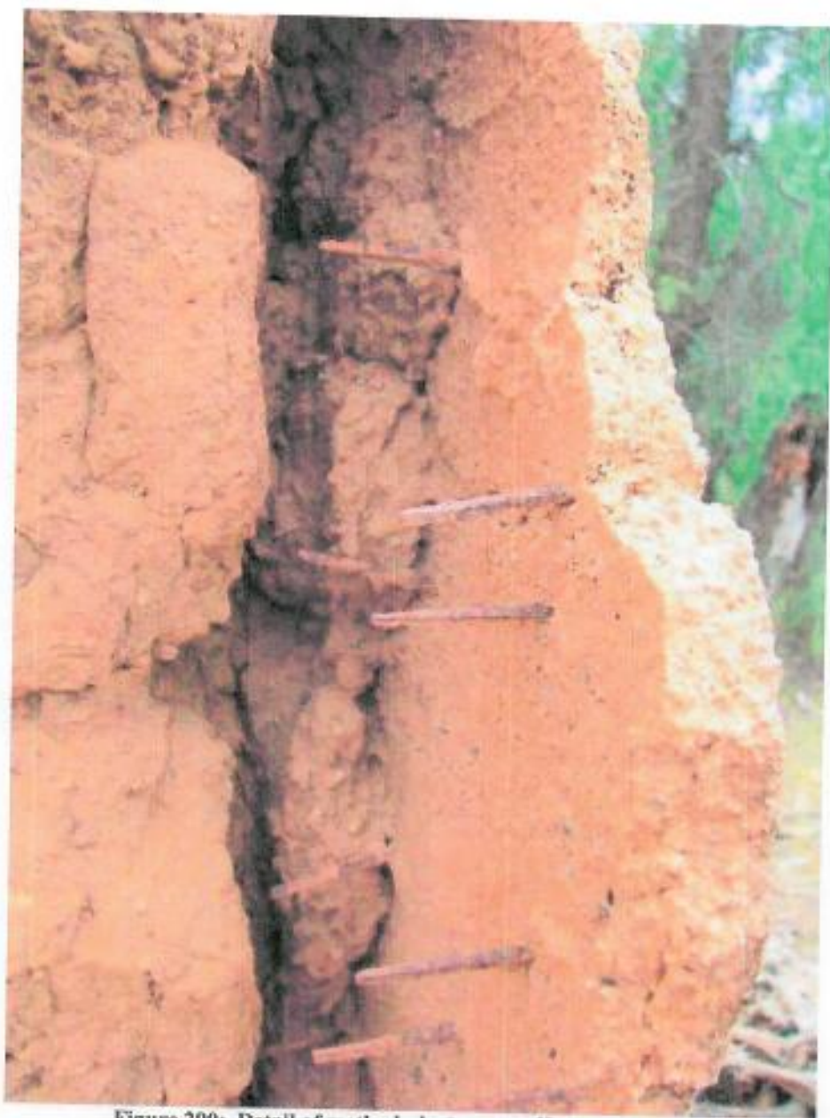
Figure 290: Detail of method plaster was affixed to the walls
