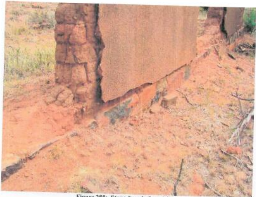
Figure 288: Stone foundation visible
