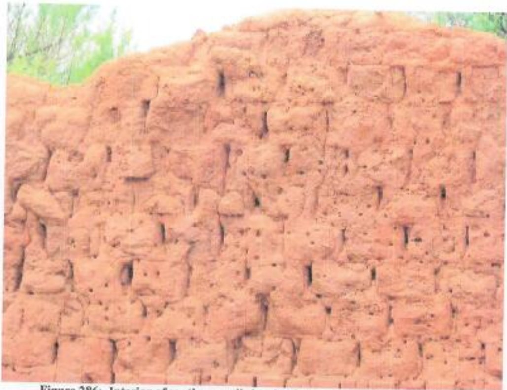
Figure 286: Interior of southern wall showing holes where plaster was affixed
