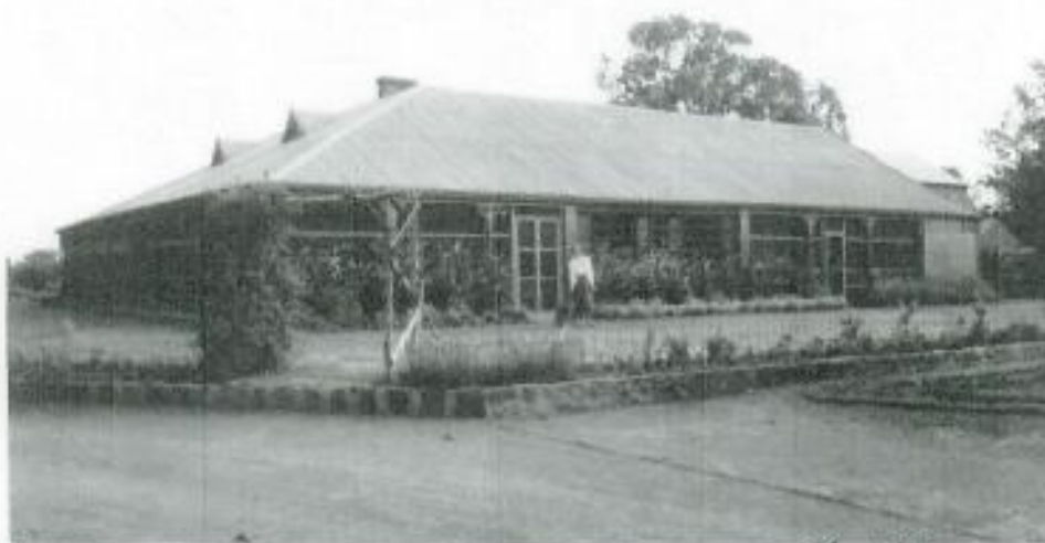
Figure 385: DBMC archive photograph of the General Manager's house in 1959
