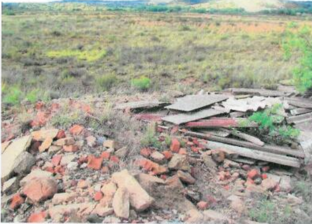
Figure 370: Remains of a demolished building
