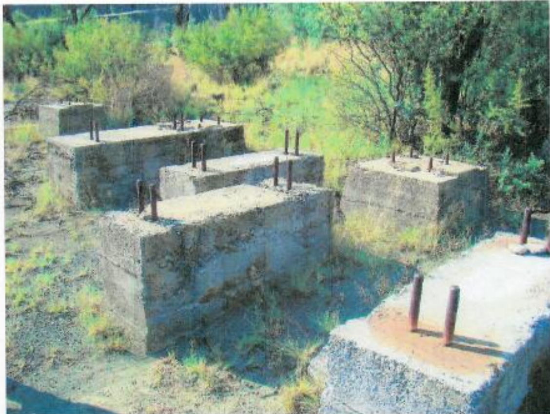
Figure 350: Remains of the old haulage system
