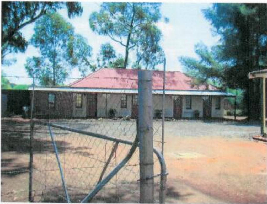
Figure 387: Outbuildings at Manager's House
