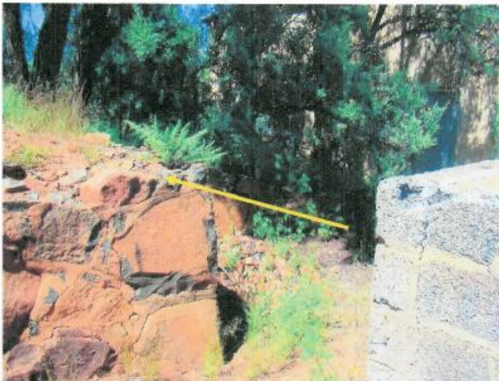
Figure 348: Stone foundations of a building with a stone ramp (arrow) immediately north of the Moth Building visible in the background
