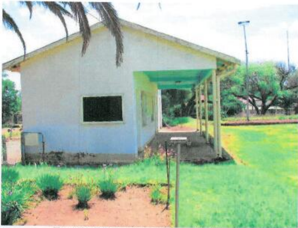
Figure 404: Side view of equipment house at bowling green
