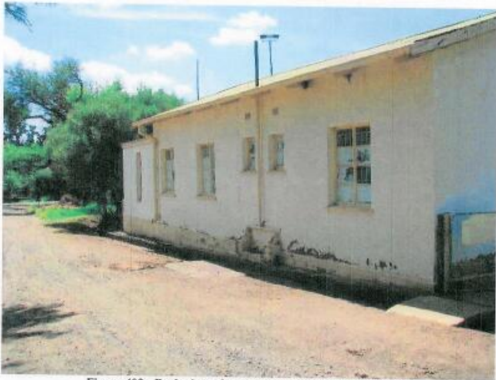
Figure 403: Back view of equipment house at bowling green
