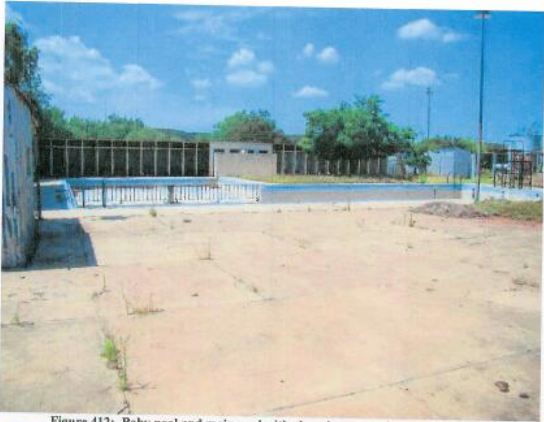
Figure 412: Baby pool and main pool with changing rooms in the background
