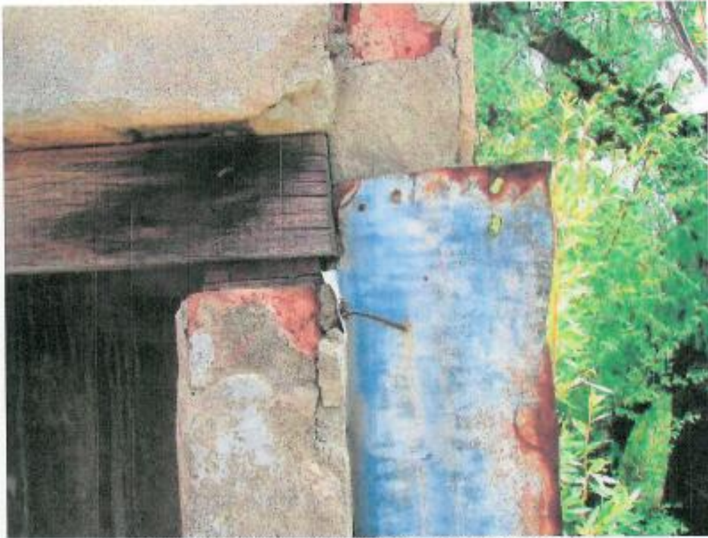
Figure 336: Close-up view of building material of chimney
