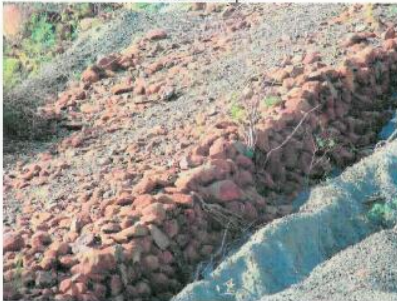
Figure 366: Close-up view of stone-packed ramp
