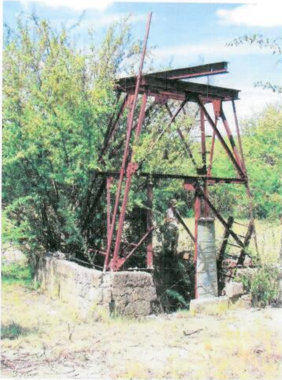
Figure 333: Remains of an old water shaft north-west of the open pit mine
