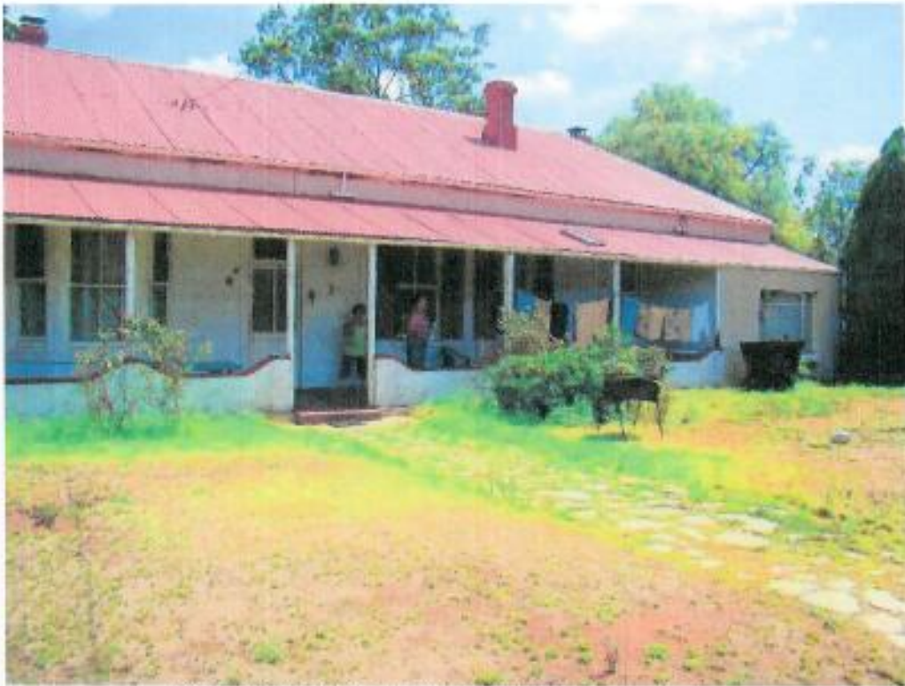
Figure 390: Front view of Underground Manager's house
