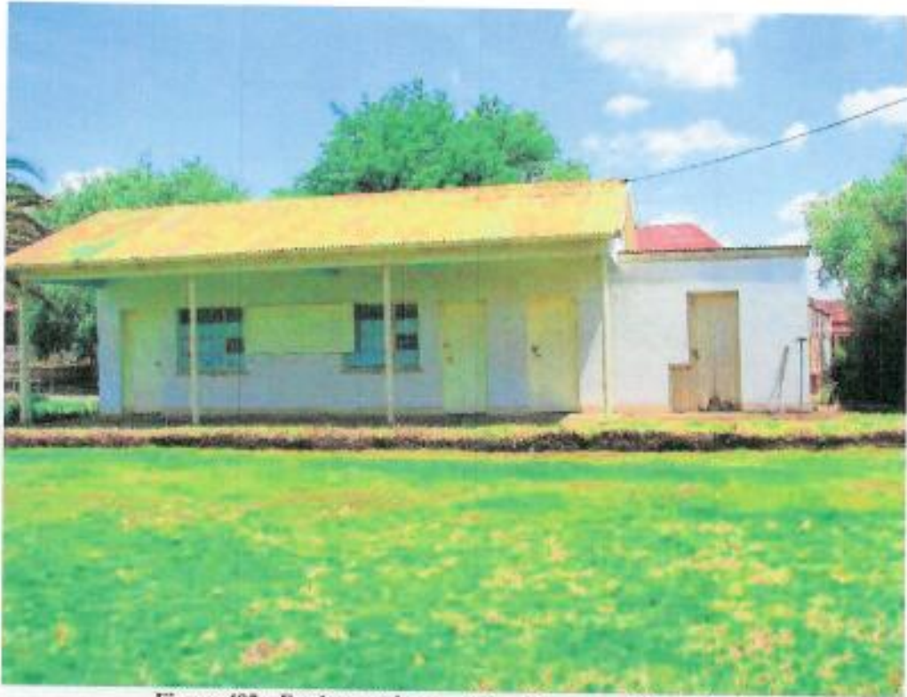
Figure 402: Equipment house at Bowling green (Front view)
