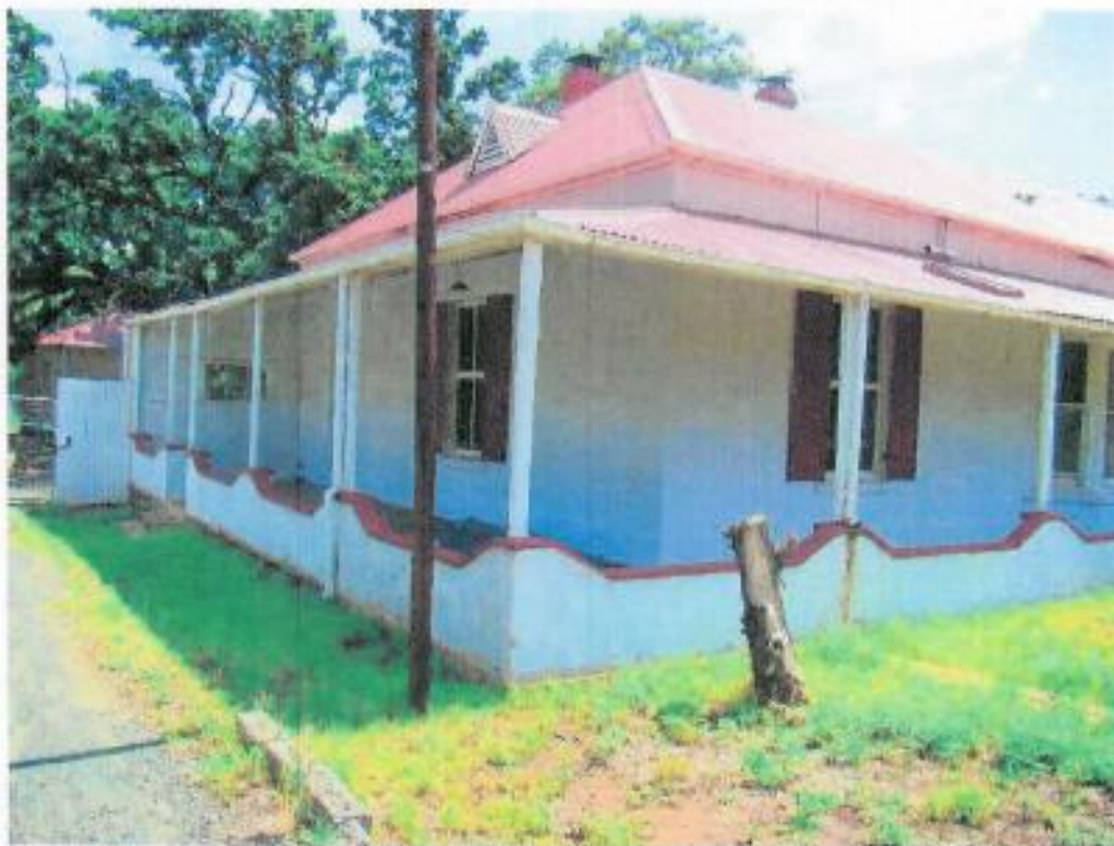
Figure 391: Side view (eastern) of Underground Manager's House
