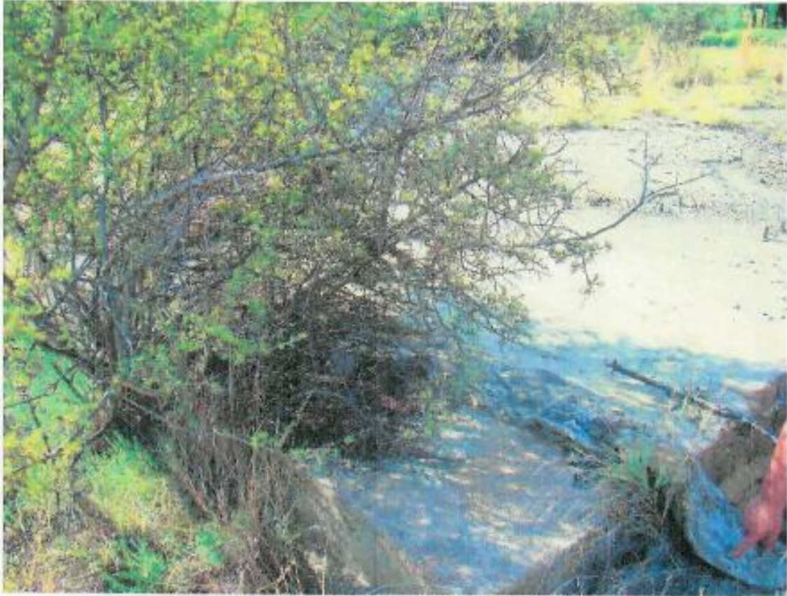
Figure 354: Remains of a cement foundation
