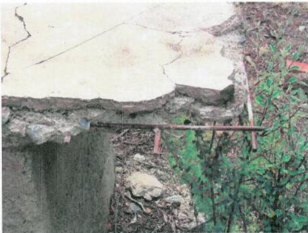
Figure 337: Close-up view of steel reinforced table top
