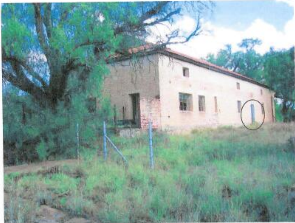
Figure 450: Unidentified building (no 25 on map)
