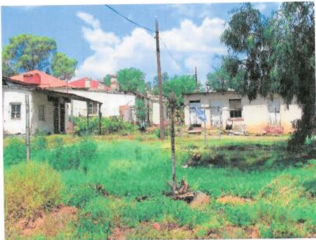
Figure 433: Outbuildings at the back of house at position 20 on map
