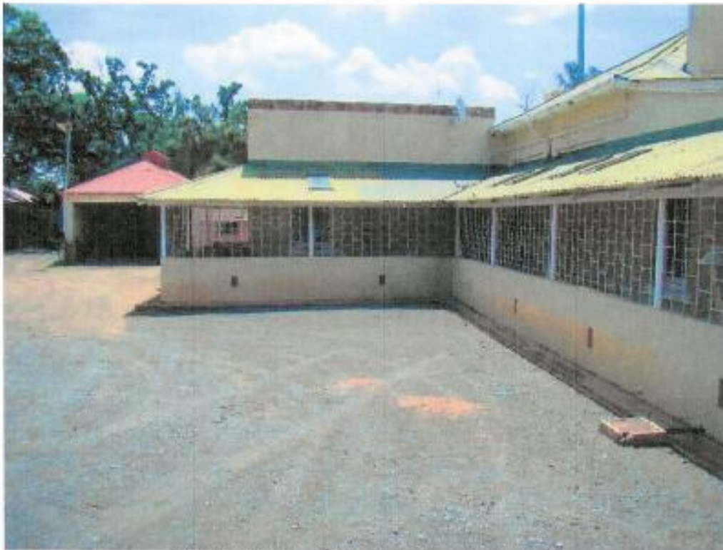
Figure 438: Head Office Building - western flank
