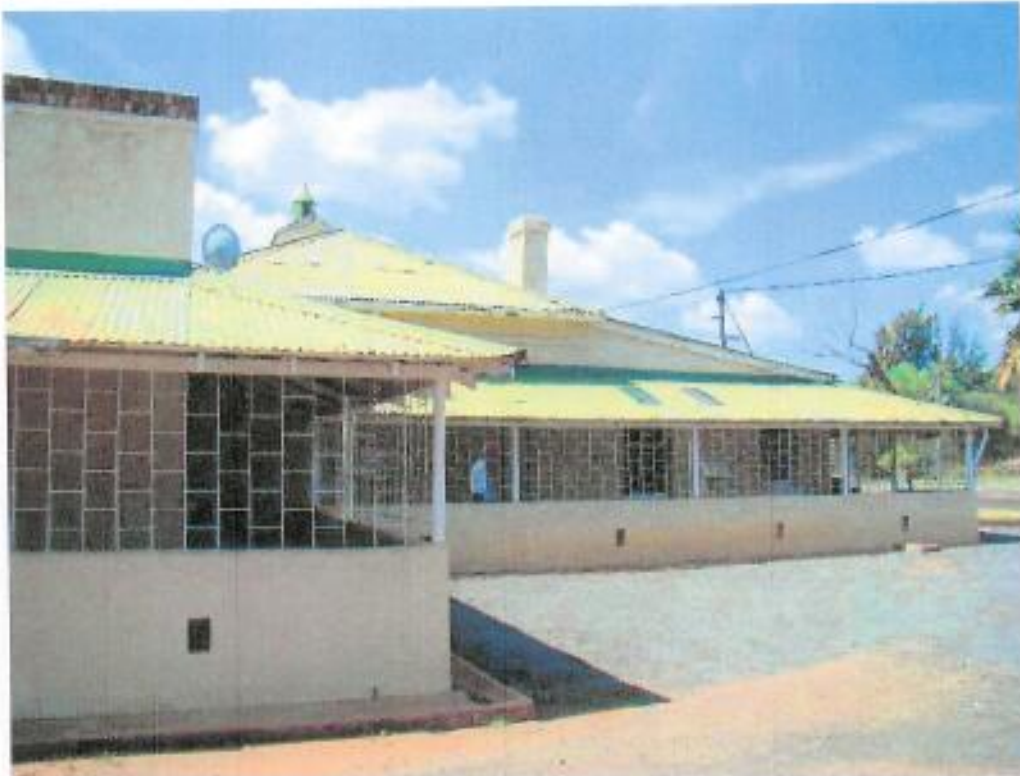
Figure 439: Head Office Building - side view (western)
