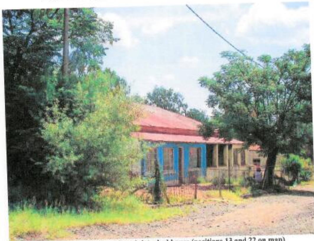
Figure 422: Right side of semi-detached house (Position 13 on map)
