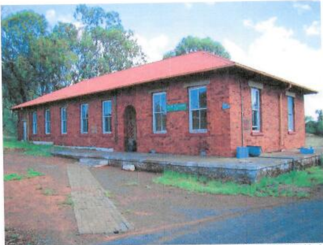
Figure 443: Engineers Office as viewed from the mine entrance gate (This building is inside the mining area)
