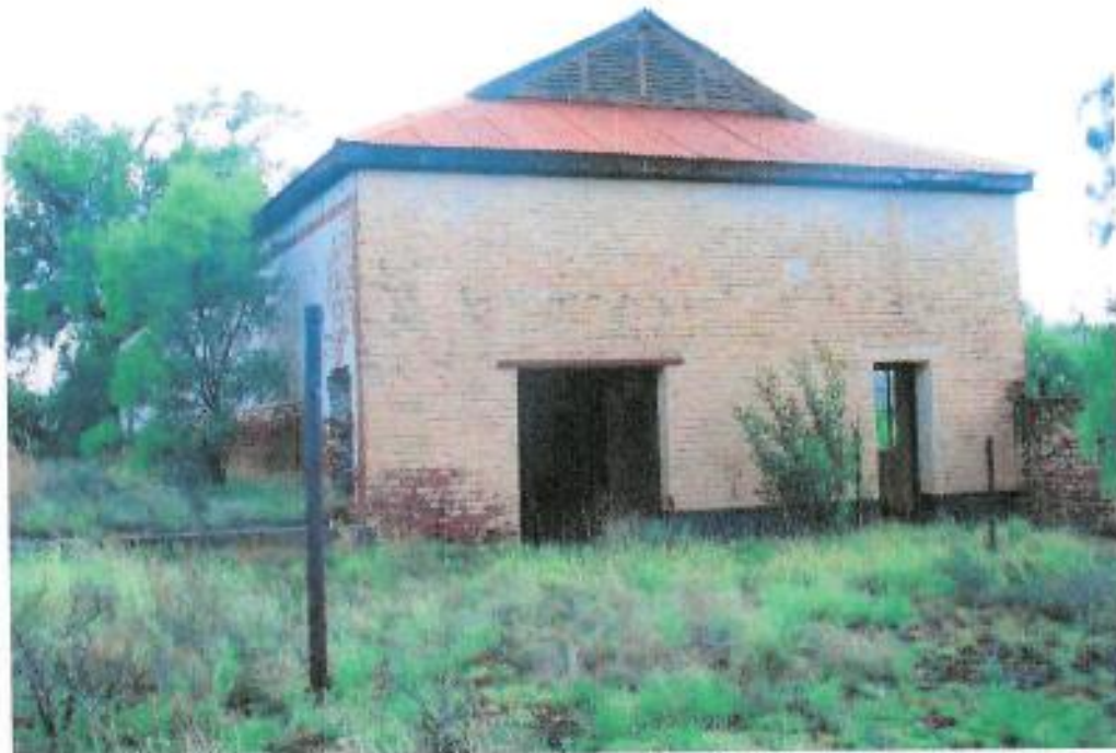
Figure 452: Northern side of unidentified structure
