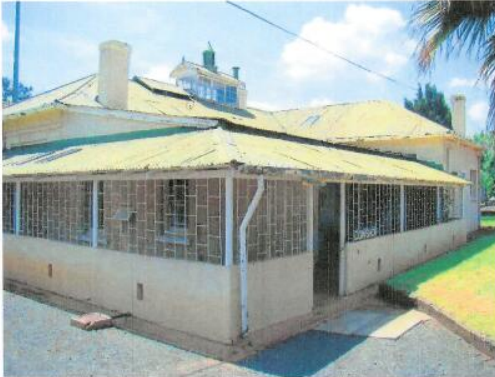
Figure 437: Head Office Building - front entrance (Position 6 on map)
