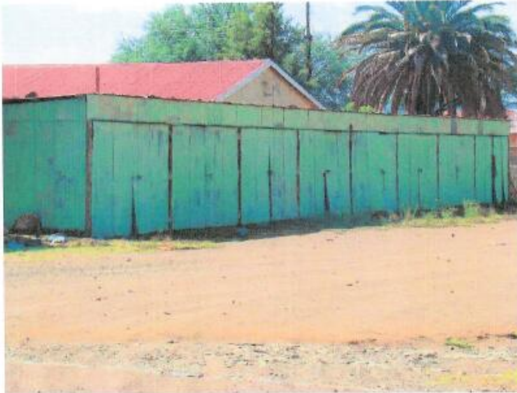
Figure 465: Corrugated iron communal garages
