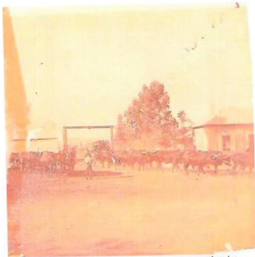
Figure 456: DBMC archive picture of the entrance to the mine
