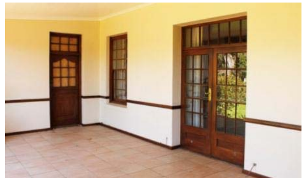
Figure 33: The front stoep of the homestead, with typical 1920s timberwork
