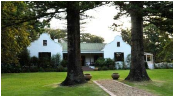
Figure 30: The front garden elevation of the Lategan homestead, built in c1894 and remodelled on the 1920s
