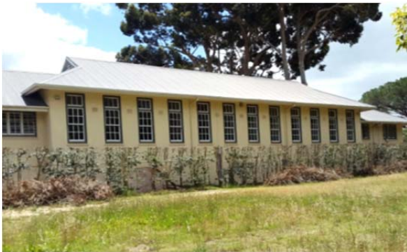
Figure 22: The former Tokai Primary School (1918), more recently known as the River Café, viewed from the south.
