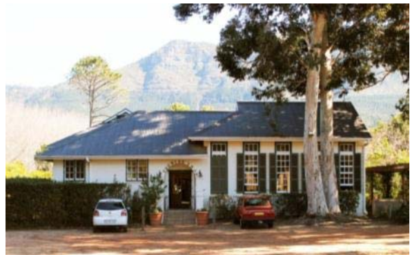
Figure 23: The main entrance to the River Café restaurant and wine shop from the parking area on the eastern side.
