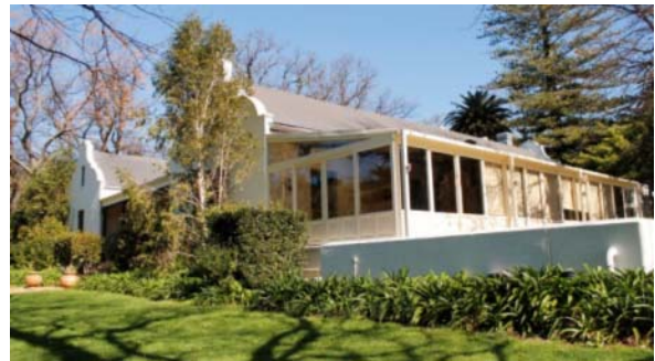
Figure 31: The intrusive 1993 conservatory addition and restaurant terrace viewed from the north.
